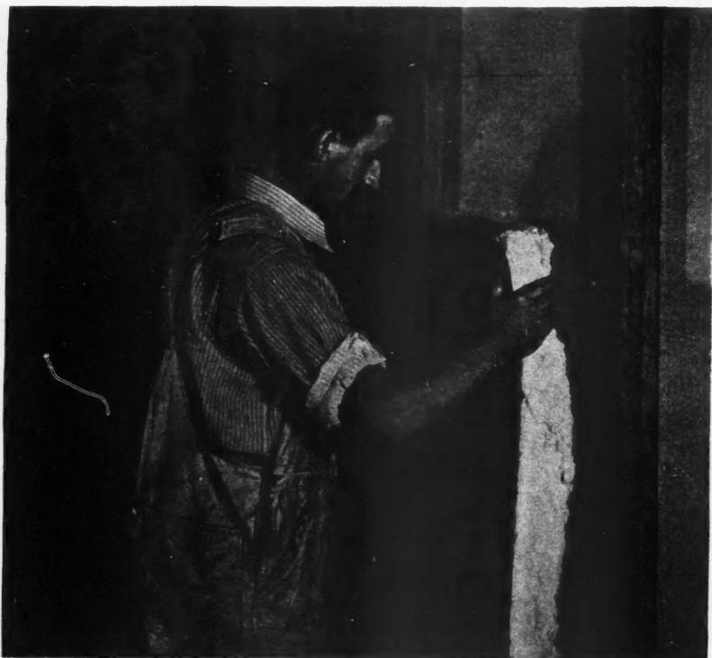
**MINERAL WOOL** in batt form simplified installation. The latest improvement is the addition of vapor-proof paper backs. All forms of insulation now are available with vapor seals, to eliminate condensation in sidewalls and attics.
