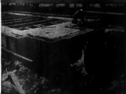
Versatile PLYSCORD Sheathing can be used for foundation forms—concrete partitions in residential construction. When used for joint formwork, the smooth concrete surface and ease of stripping the forms are noted.
