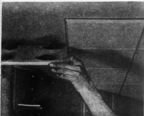
**FIBRE** board cutting tool for hand grooving allows a wide choice of panel and border patterns to be worked into the walls and ceilings.
