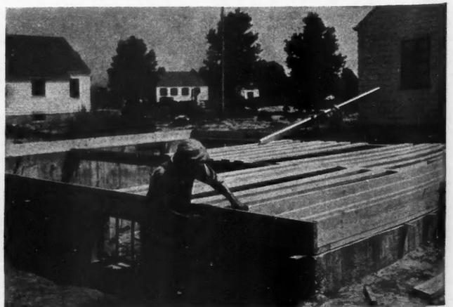
ON MILLS AND SONS houses, joists of stock length quickly set in place for spiking after box sills are built and leveled.
