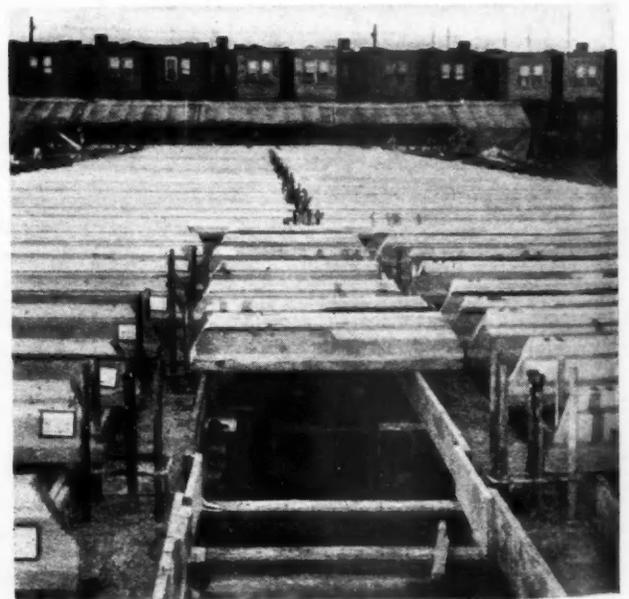
CONCRETE floor joists in place in Philadelphia's Tasker Street housing project, which required some 45 miles of joists.
