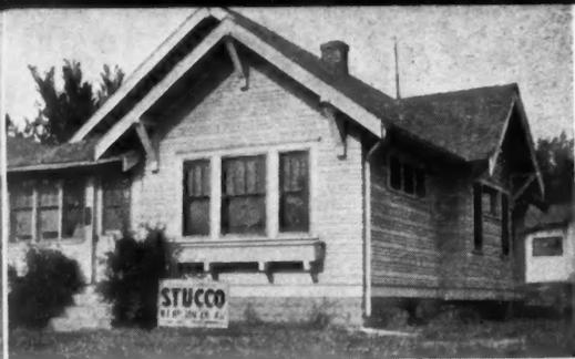
THE top illustration at the left (1) shows a small bungalow just before Nelson resurfacers start work; paint failure due to structural faults is to be remedied (2) with a stucco overcoating.
