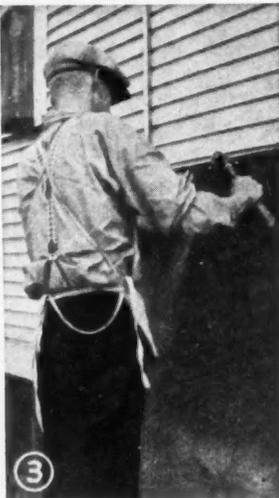
THE paper applicators are the first crew to come on the job, tightly covering building with well lapped asphalt paper (3). This is followed with the installation of mouldings at openings by carpenter crew (4).
