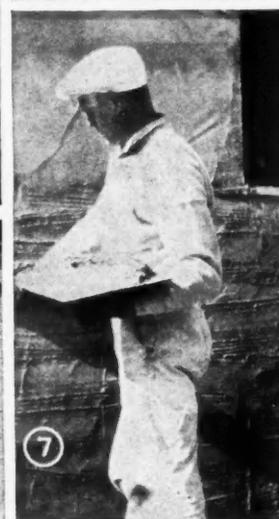
AFTER galvanized metal lath has been put on with galvanized nails (5), the browners apply the first coat of high early strength portland cement stucco (6). This is followed with a scratch coat of cement stucco (7).
