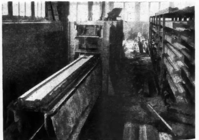
LITH-I-BAR concrete joists emerging from W. E. Dunn machine in Formigli plant, Philadelphia, for U. S. housing project.
