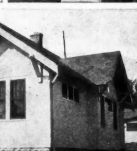
THE final or dash coat of white portland cement, white silica sand and mineral colors, if a tint is specified, finishes the job (8); the resurfaced home (9) again presents an attractive exterior.
