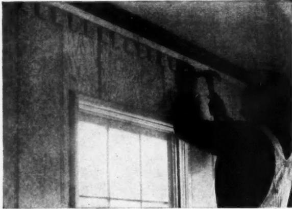
DECORATIVE plywood in living room. Dentil is made from 1" x 4" crown mould and 1 3/4" x 2 1/4" blocks individually nailed.
