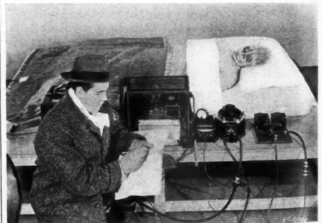
**MAGGIE'S ELECTRIC UNDERWEAR**—Shown above is "Maggie," a bedridden dummy maintained on the roof of the General Electric factory at Bridgeport, Conn., for purely scientific purposes. She not only has an electrically heated blanket, such as was mentioned in this column recently, but wears an electrically heated suit of underwear such as G-E is making for U. S. aviators.
