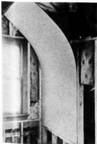
WALLBOARD of asbestos-cement is flexible enough to be curved.
