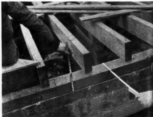
SEASONED substantial framing is used as illustrated in this photograph, showing 4 x 6 notched and lapped sill and 3 x 8 joists.
