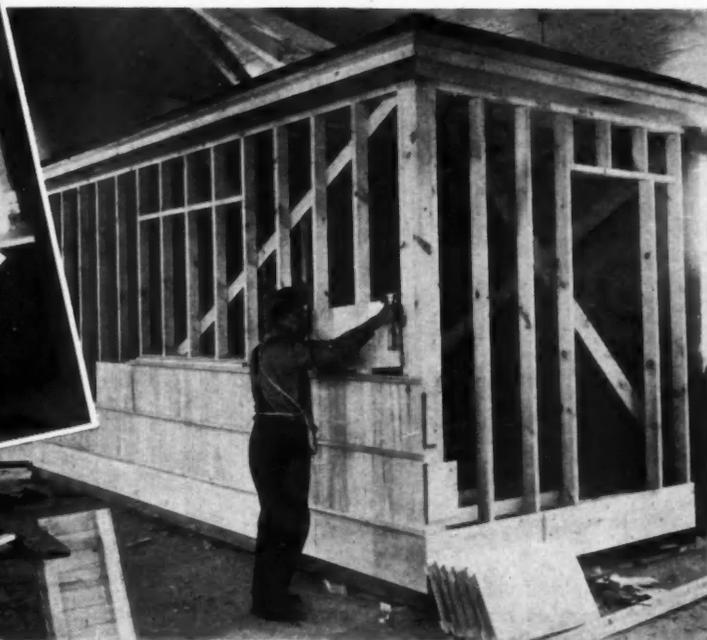
**RIGHT:** Placing exterior panels on standard stud frame, 16 inch centers. Panels are 16 x 32 inches. **ABOVE:** Close-up of panel.
