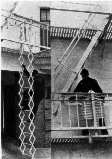
"SAFEXIT" in lowered position and (at right) retracted when not in use.
