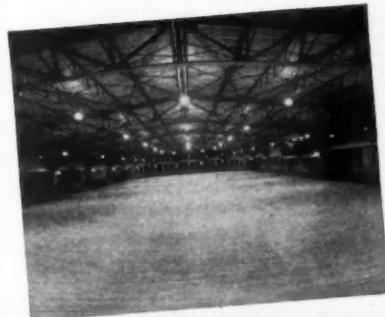
Floor designed, laid in mastic over concrete, by Cincinnati Floor Company. Flooring was lateral-nailed and rolled with heavy roller before sanding. Result is a remarkably level, smooth and quiet roller rink floor.
