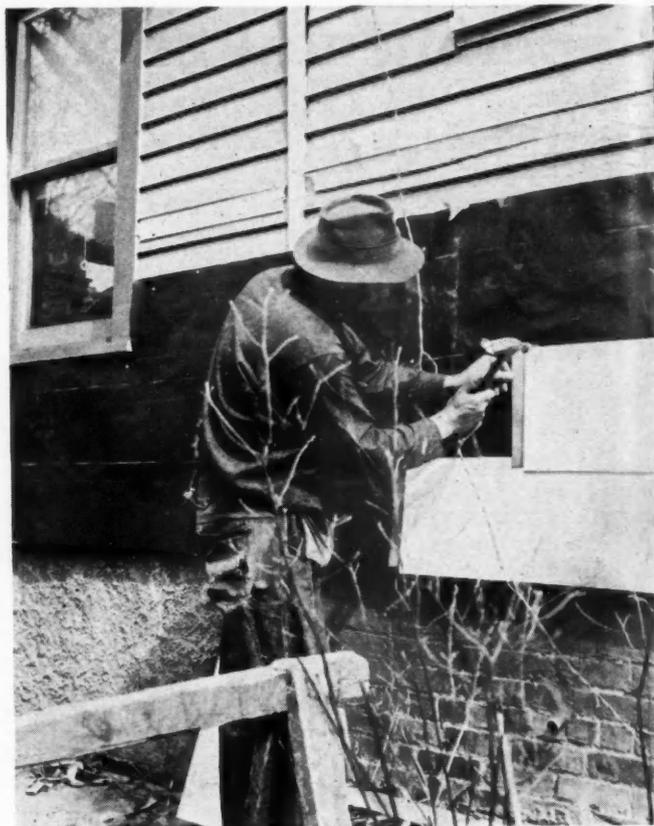
FELT BACKER strips are placed behind vertical joints. Wood bevel strips (above) provide smooth nailing surface.
