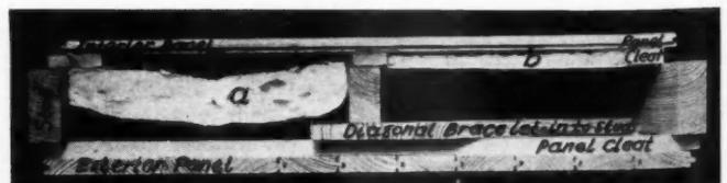
CROSS-section through complete wall showing alternate forms of insulation.
