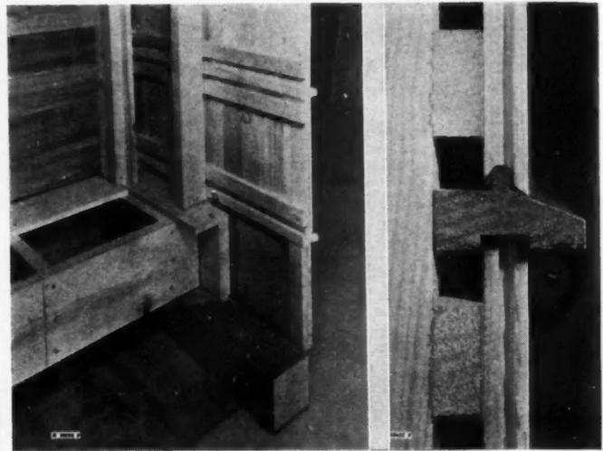
LEFT: Back view of exterior wall showing panel unit cleats and mullion bars against studs. RIGHT: Vertical section through horizontal mullion bar showing rain protection.
