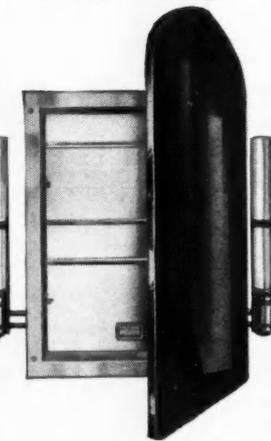
(Left) Cabinet with lighted interior. Open door—light switches on. Close door—light switches off. For night light, leave cabinet door open. Tubular light brackets are equipped with revolving shields that direct light onto mirror or into room.
