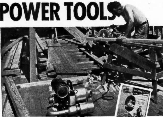
Run your electric hand tools with Homelite Portable Generators. You eliminate power installation difficulties—delays, expenses, red tape. You have electricity instantly available for every job, large or small. All you do is carry your 83 pound Homelite Generator from tool box or truck to spot where men are working. You start its built-in gasoline engine—instantly you get 1800 watts at 110 volts, enough power to run several tools at top capacity.
