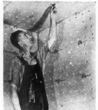
TILE AND PLANK Clips provide effective concealed fastening for insulating tile and plank, having tongue and groove joints, without marring the surface of the board; utilize wood lath instead of more costly furring.
