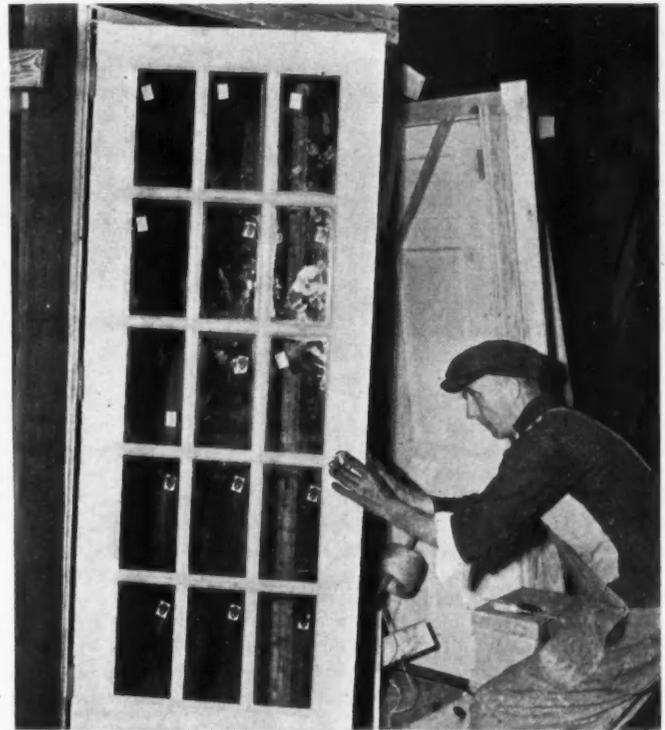
**DOOR IS HUNG** in factory and delivered to job complete with hardware, latches, locks, hinges, glass and prime coat. The same is true for all other items such as cabinets, drawers and cases.
