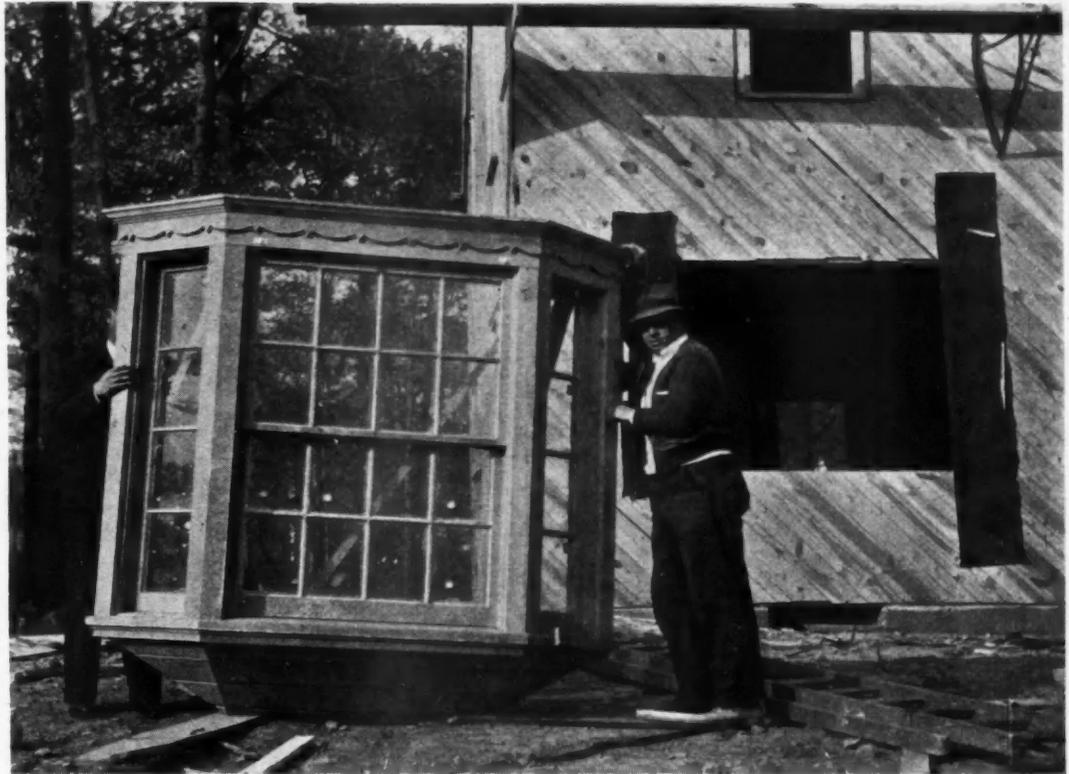
**SEEN BELOW** are additional millwork items as delivered to the job complete with flashing, hardware and prime coat. Practically all skilled woodworking is handled in the shop.
