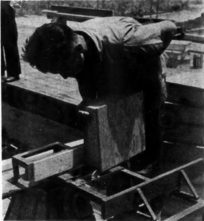
**FLANGES** of the Plycell units are glued on a gluing machine before placing in the wall. Waterproof casein glue is used.
