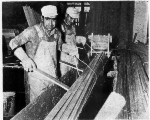
ALL MOULDING AND TRIM are given a paint dip in the Mott factory before going out to the job.
