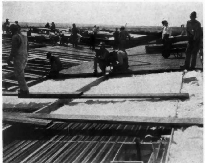
FIBERGLAS and steel being combined in successive layers in roof of Ft. Worth bomber plant. Below, view of completed framework.
