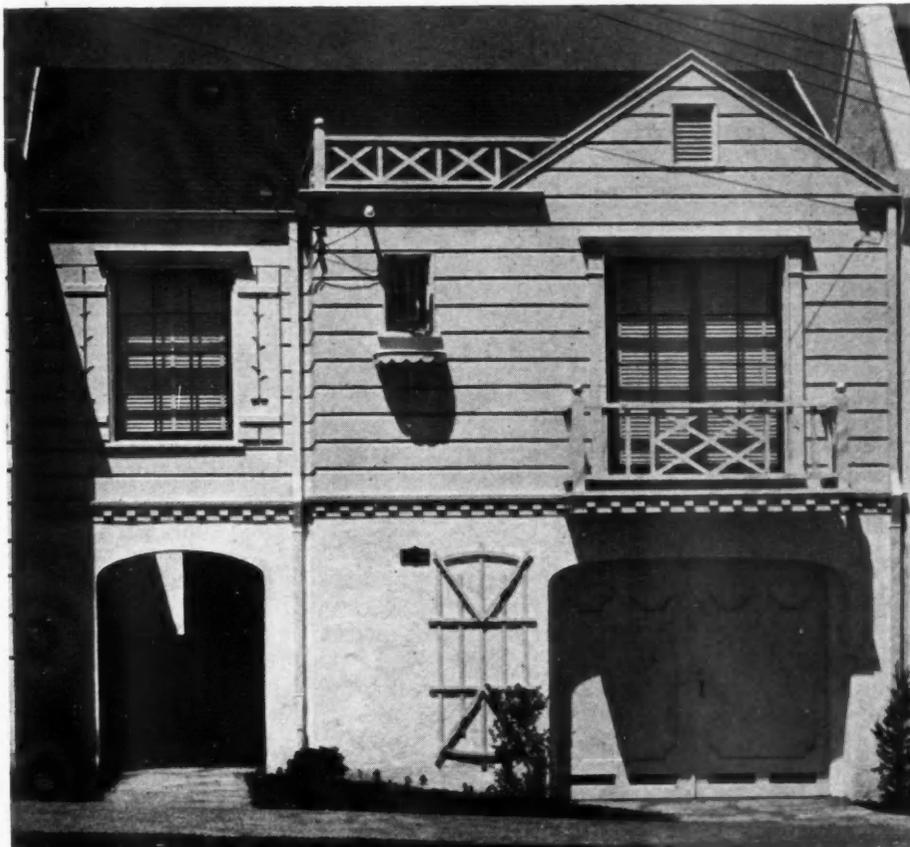
ABOVE: A typical Doelger model row house with rooms placed over "above ground" basement, used for garage and entrance (through arch at left.) Arrangement is typical, and planned for 25-foot lot, standard for this area.
