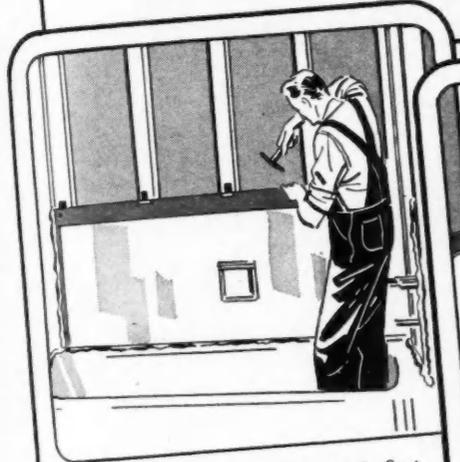
**2. SET PLATE** at back of tub first. Merely nail through plasterboard flanges and use special clips supplied.
