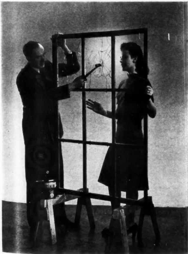
NEW LIQUID coating prevents flying glass during air raids.
