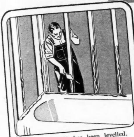
**1. AFTER TUB** has been levelled, place roll of mastic around rim for waterproofing. Butter studs with mastic before setting glass.
