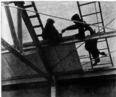
View showing workmen applying Porcelok. No scaffolding required. Application from upper surface of roof. ABOVE: Detail of side joint.
