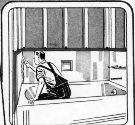
**4. CLEAN GLASS** and fill joints carefully with pointing compound supplied. This assures thorough waterproofing.
