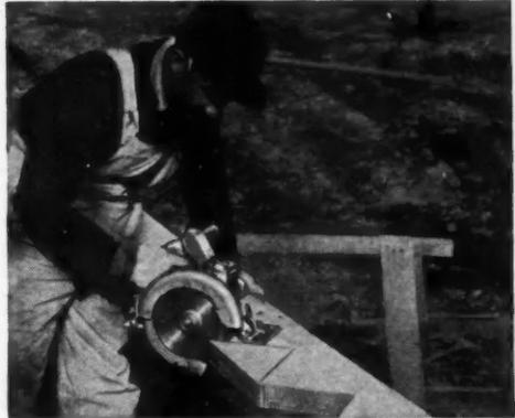
**CUTTING** stair carriages with Black & Decker Electric Saw takes only 35 minutes for a set of 3 carriages—compared to the cost of a half day's work when done by usual hand-sawing methods.
