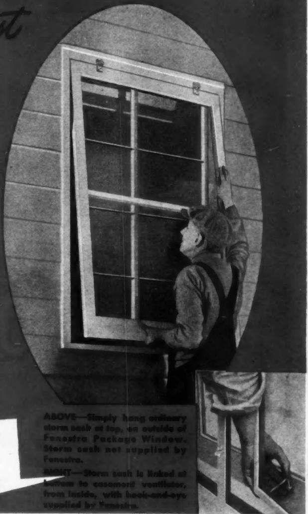
ABOVE—Simply hang ordinary storm sash at top, on outside of Fenestra Package Window. Storm sash not supplied by Fenestra.
