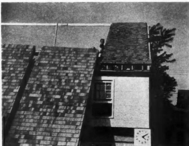
SHINGLED roof sections being moved into place.
