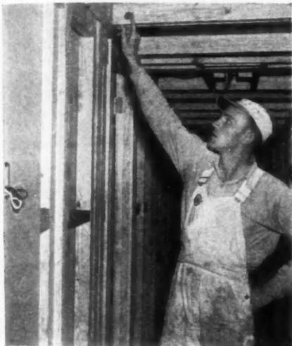
ABOVE: Workman points out one of the bolts which holds the demountable bunkhouse sections together. Exterior view, floor plan, section and elevation of this interesting housing shown on this and the opposite page.
