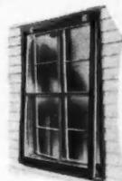
When this double window is opened for winter ventilation, the storm sash forms a protecting canopy—keeps snow or rain from entering a room.
