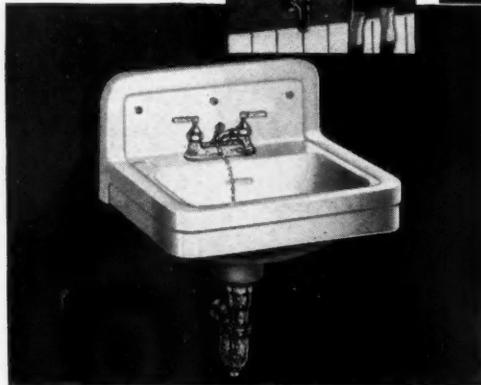
● CE-764 new "Victory Cantonment" lavatory. Made of easily cleaned vitreous china with cast iron trim, heavily galvanized. Mounts directly on the wall with screws—no hangers needed. Uses a minimum of critical materials.
