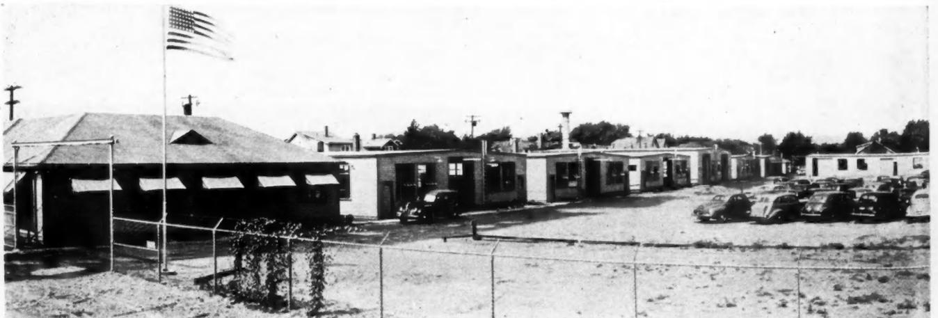
**CRITICAL MATERIALS CONSERVED** in this new plant for The Ready-Power Company, Detroit, Michigan. Eight wooden unit buildings, each 60' x 80', give required floor space, light, air, and break up fire hazards.
