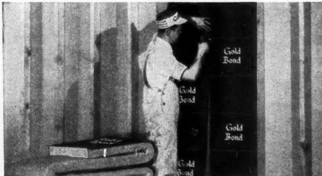
**1. SUGGEST ROCK WOOL INSULATION!** Attic rooms should be insulated for comfort. You can get all the Gold Bond Rock Wool you need in a hurry—in batt, blanket and loose form. It can be applied to walls and ceilings in a jiffy, and without specially-trained workmen. It is fireproof, vermin-proof, permanent in efficiency. Cuts heating fuel consumption as much as 33 $\frac{1}{3}$ %!
