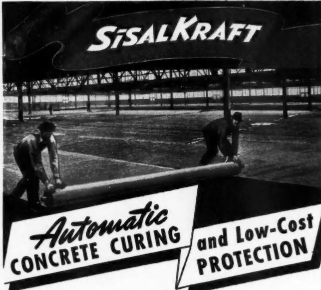
The SISALKRAFT method of concrete curing is simple, positive, economical. Cover the freshly finished slab with SISALKRAFT and forget it. No sprinkling or flooding — no sand, straw or burlap. The paper can often be re-used many times, offering great economy in both material and manpower. Write for complete data and sample.
