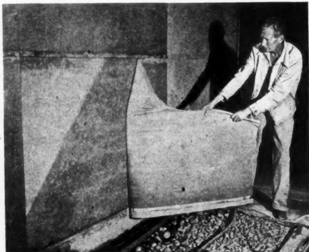
CONCRETE cast against the new Hydron form linings is several times as resistant to weather and abrasion as ordinary concrete.
