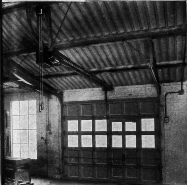
Electrically operated "OVERHEAD DOORS" may be controlled by pull station, push button station or key switch station located at any convenient point.
