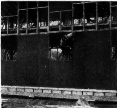
**Gold Bond Exterior Board** is a combination sheathing and siding material which covers up to 20 square feet in one operation, saving time and money on the job. It's made of husky extra-thick Gypsum Board panels with durable overcoat of weatherproof asphalt roofing. A rigid, sturdy type of construction for plants and farm buildings.
