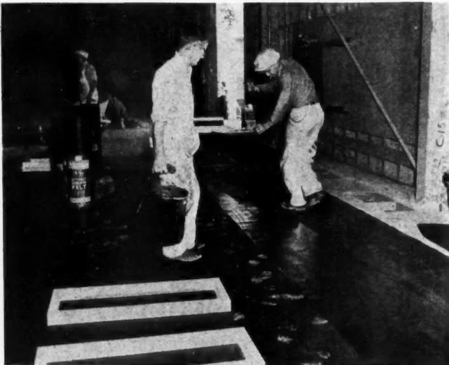
IN CONSTRUCTING the "floating floor," the first step is to mop two layers of saturated felt on the dry-clean concrete slab. RIGHT: After the felt has been laid, kiln-dried sand is spread over the
