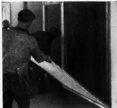
**Gold Bond 1" Solid Partition Panels** save time, materials and expense in factories and offices. They go up in a hurry and are held in place by mouldings—no nails are required for the panels themselves. Tough enough to withstand the hardest usage. Can be completely salvaged when temporary structures are torn down.
