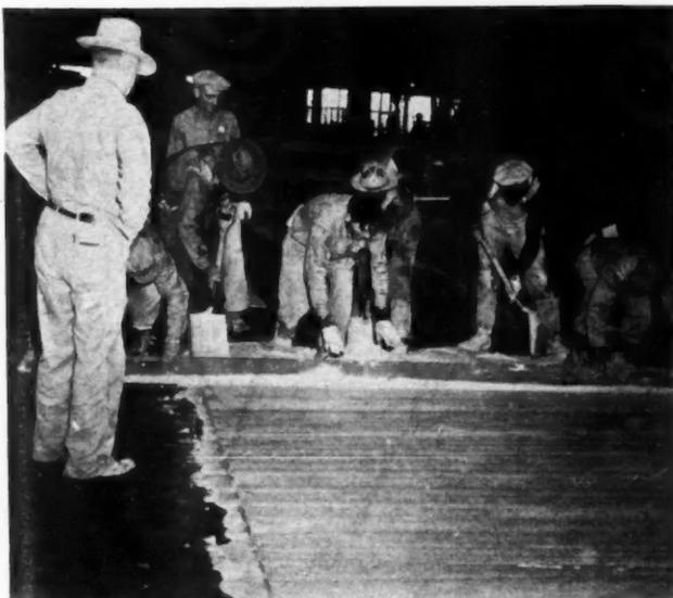
WHITE CEMENT topping being applied over grey concrete base. Can be applied to new or old floors to provide clean, light-reflecting surface that conserves power, increases production.
