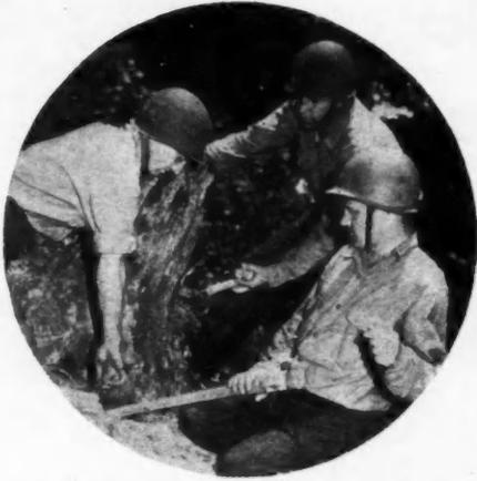
**FROM CIVILIAN** construction work to the Navy's Seabees these men went. Here they are inserting sticks of dynamite to blast a stump out of the way.
