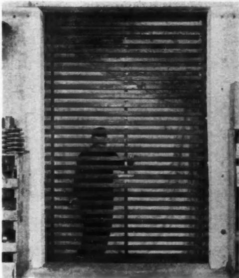
NEW rolling wood grille or barrier which uses a minimum of critical materials.
