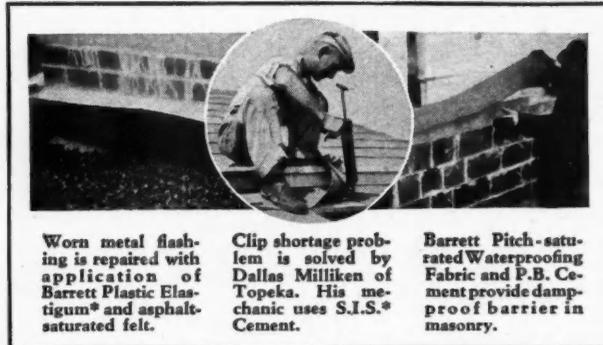
Worn metal flashing is repaired with application of Barrett Plastic Elastigum\* and asphalt-saturated felt.
