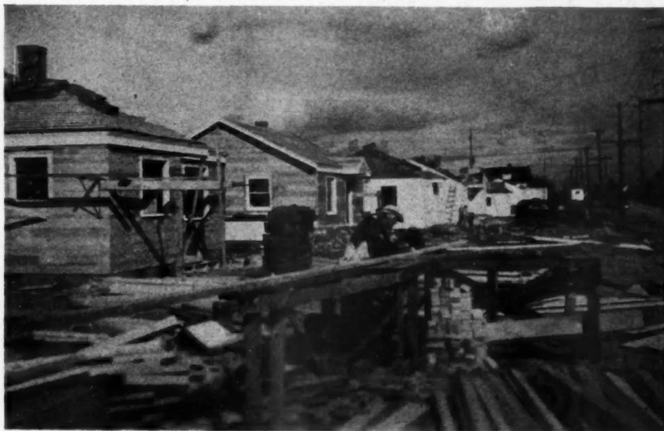
POWER SAW and one man cut all framing lumber to length on the job.
