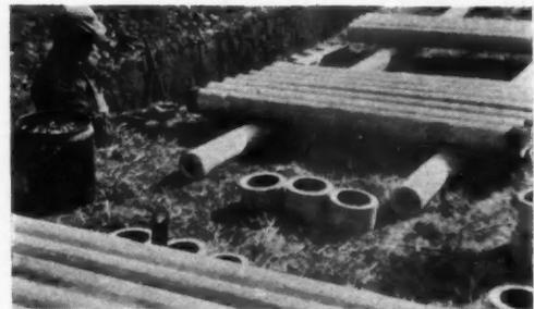
WORKMAN applying joint sealing compound to asbestos-cement conduit.
