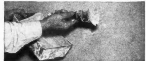
After Taping Cement is dry, apply the white Finishing Cement on the joints.
