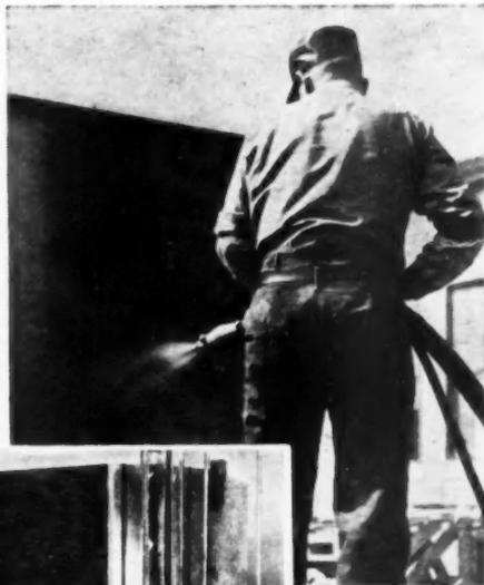
**WORKMAN,** above, applying pneumatically shot concrete to test panel; Colburn system model is shown at left.
