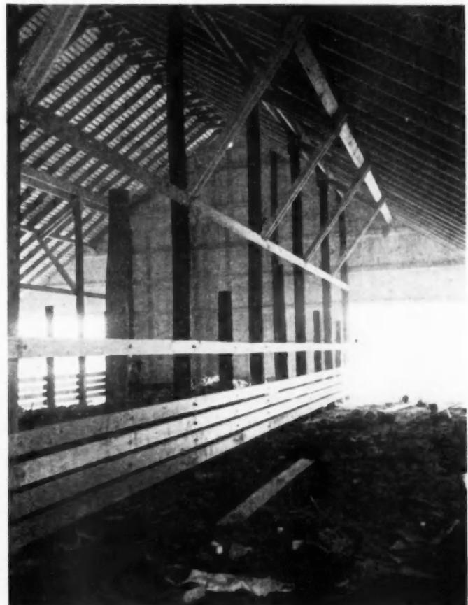
STEPS IN ERECTING a pole & rafter barn. Left, workmen set the butt-treated poles plumb, on concrete footing pads; then cut off tops to desired height, as shown above. Braces, side girts, rafters, and outside covering are added as shown in photos to right.
