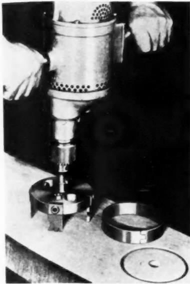
The advantages of ring-connector joining in timber construction have been known for some time; this power-driven cutting tool has eliminated much of the tedious hand labor formerly required, and has speeded up this type of construction.
