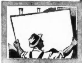
The big panels of Insulite Bildrite Sheathing fit quickly into place and cover a large surface in one operation. Insulite Bildrite Sheathing provides four times the bracing strength of ordinary wood sheathing, horizontally applied.
