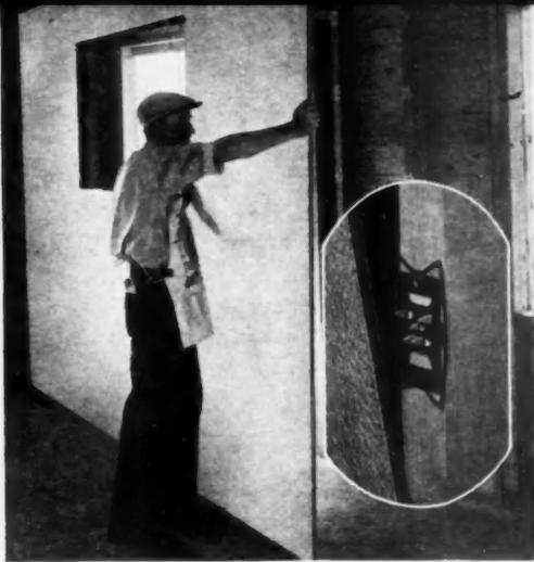
A unique feature permits movement of the panel to compensate for normal structural settlement. No face nailing. No taping of joints. No nail holes to fill. No battens.
