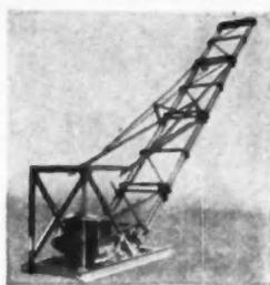
Jaeger Self-Raising Tower, quickly assembled on ground and raised by its 17 H.P. "Hoister," can be moved around job on its own skids — elevates loads up to 2000 lbs. Cage, with Automatic Safety Lock, handles largest concrete cart or 2 barrows. Standard height is 37 ft.—10 ft. sections up to 67 ft. can be added. Saves time, material, labor, pays for itself in no time.
