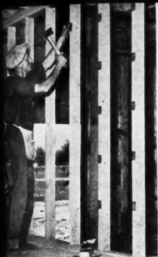
Upon Floating Fasteners are nailed directly to studs and joists for anchoring Strong-Bilt Panels securely from the back.
