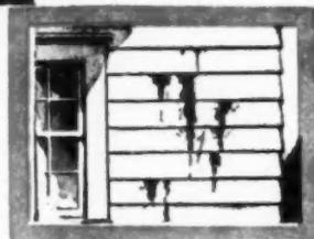
Brown stain or paint blisters can be an indication of destructive condensation within the walls. With the Insulite Approved Wall of Protection this problem is minimized.
