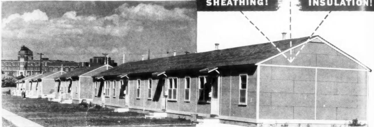
Row of four-family houses in Bill Holt FPHA Housing Project, Great Falls, Montana, with walls constructed with multiple-function Celo-Siding.
