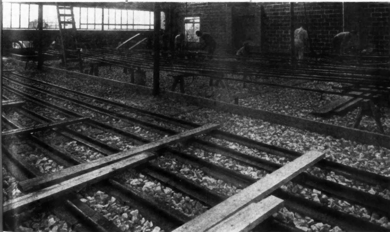
WELDING the three banks of grid coils for the Murray Corporation radiant heating installation; straight runs for 1¼-inch wrought iron pipe resting on 8-inch wide strips of 1-inch Celotex. To complete floor, 6-inch slab was laid; drawing at left shows layout.
