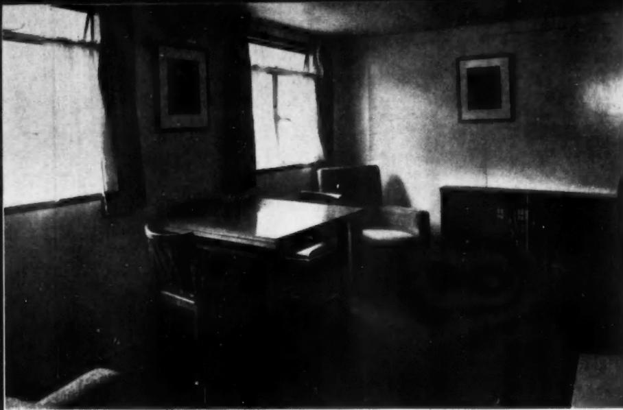
**LIVING ROOM** of British prefabricated home planned as temporary units for bombed out families, has plywood walls, ceiling and steel sash. Heating unit is on opposite side.
