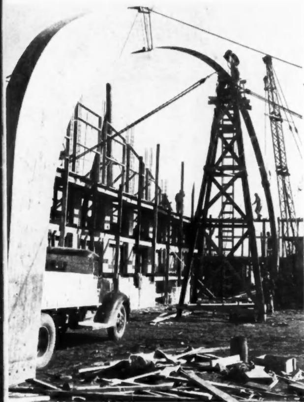
**FEEDING THE FOLKS** who make the B-17 Flying Fortresses and the B-29 Superbombers at the Seattle main plant of the Boeing Aircraft Company; view at right shows new Cafeteria in use. Upper construction shots reveal how the giant arch trusses were erected.
