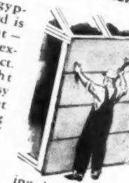
Celo-Rok Weather-Proof Siding is a fire-resistant gypsum board for use in place of both sheathing and siding. Treated with weather-proofing compound. Green-finished exterior requires no painting. 1" thick with ship-lapped long edges; 1 $\frac{1}{2}$ " thick with T&G long edges. Sizes: 24' x 6', 8', 9' and 10'.
