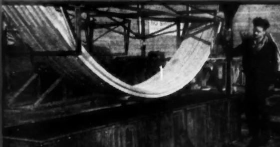
\* This is a hydraulic-plunger type of operation. In this model dead weights are eliminated, submerging is achieved by top side pressure. Tanks of this type are used for structural members and for fabricated pre-shaped stock, such as the Quonset arches pictured. Quantities of stock handled per immersion are comparatively small.
