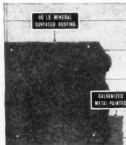
Install rigid drip edge extending  $\frac{3}{8}$ " beyond fascia board. Use galvanized iron painted both sides. As starter strip use Bird Black Mineral Surfaced Roofing at least 6" wider than roof overhang. Lay parallel to eaves with lower edge flush with drip edge. Spot nail in place. Apply shingles.
