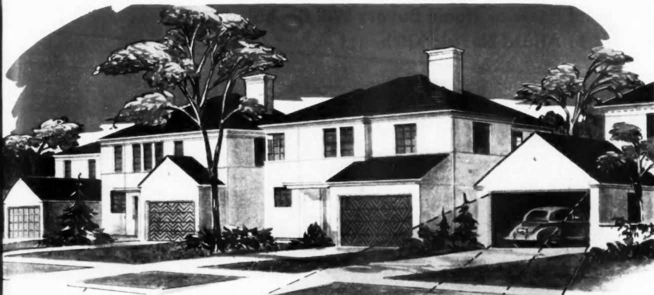
This door, custom-built by Crawford, is a four-section, two-car unit, mounted in Crawford standard hardware. The sections consist of a sturdy framework covered with plywood in which the design is reproduced by routing.
