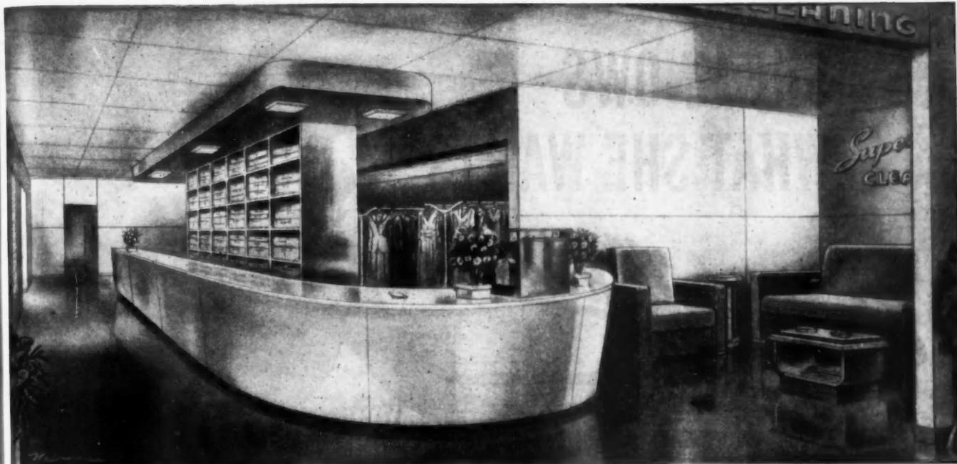
This attractive, modern dry cleaning sales office has walls and ceilings of beautiful Douglas fir plywood. Curved counter treatment is accomplished with plywood, too, for this versatile "miracle wood" can be easily bent to simple curves without steaming and without the use of special tools.
