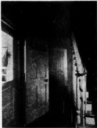
*This entrance door, an attractive stock design of Ponderosa Pine, effectively bars out cold because it is machined accurately to fit snugly for maximum weathertightness. Note that the door is hung with three hinges for correct balance.*
