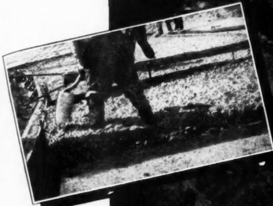
PLASTICITY. Although the Air-Entrained concrete in above photo looks dry, its plasticity is shown by the worker's feet which have sunk clear through the mass.
