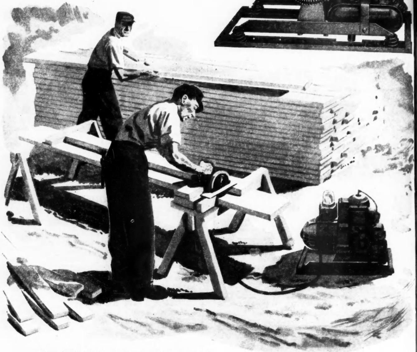
... Use the Homelite power method ... the mass production method. All you do is line up your lumber, plug a power saw into a Homelite Portable Generator and the job is but a few seconds from being done.
