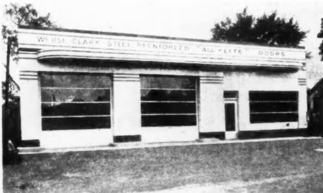
usage, according to the manufacturer. Because the new type door eliminates the wood divisions, it presents a very attractive appearance. Unobstructed glass lights to a width of twelve feet can be manufactured. One of the reasons for successful operation of this door is because the lights are set in a wood frame which is protected by specially designed reinforcement and steel angles.
