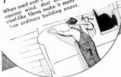
Sisalkraft does a thorough job. Applied over sheathing, as a flashing around door and window openings, under floors and beneath roofs, Sisalkraft is unmatched as a moisture barrier. It shuts out wind and dust as no other building paper can — makes homes more comfortable. Use it—explain its benefits to your prospective home buyers. They will appreciate your foresight in assuring their greater comfort—your consideration in helping reduce their fuel bills.
