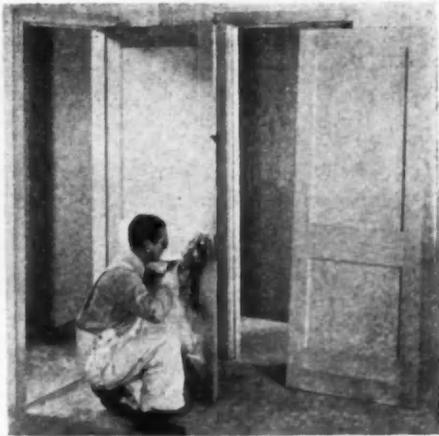
Pre-fit doors eliminate cutting, fitting.
