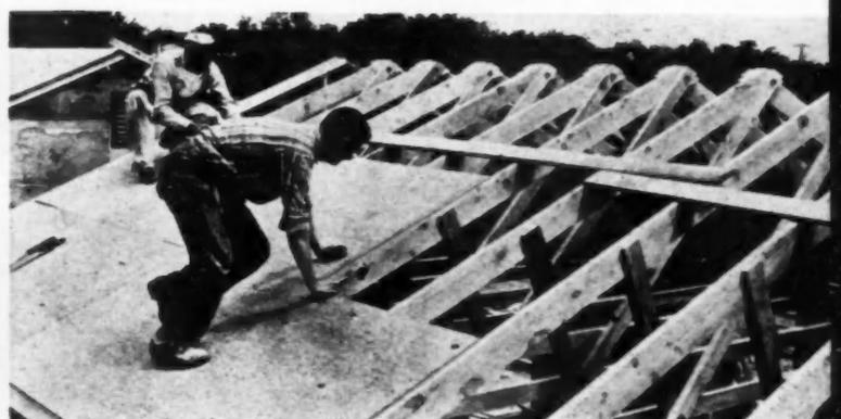
Plywood roof sheathing being applied over new Teco truss rafters which eliminate need for bearing partitions.
