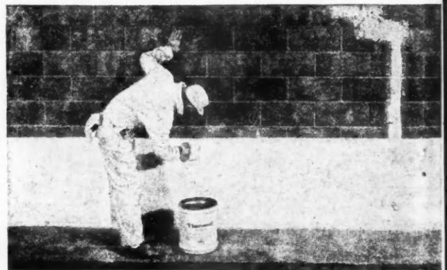
**B. THOROSEAL**, a slow-set hydraulic compound, gives the applicator 3 to 4 hours before set begins, to brush THOROSEAL into the masonry surface. (Scrubbing not necessary, as THOROSEAL is prepared especially to flow easily and quickly into every crack, void and defect in the surface, where it becomes structurally stronger than the surface to which applied.)
