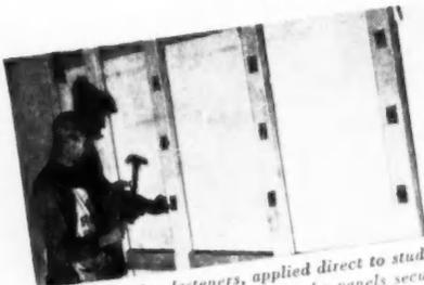
Upson floating fasteners, applied direct to studs or furring on 16" centers, anchor the panels securely from the back. No ugly nail holes to countersink or fill.
