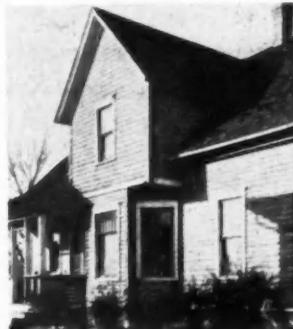
Exterior walls refinished with asbestos-cement shingles. Photo: Keasbey & Mattison.
