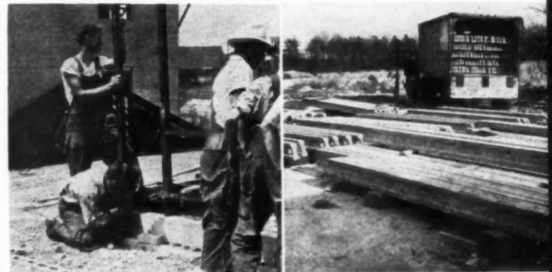
Welder anchors steel frame assembly to joists. Photo: Great Lakes Steel Corp. Precast concrete joists ready for delivery. Photo: W. E. Dunn.
