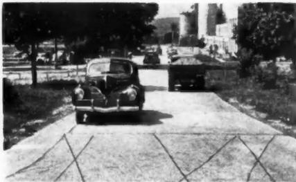
Scaling indicated on normal slab in foreground. Air entraining on balance was scale resistant.
