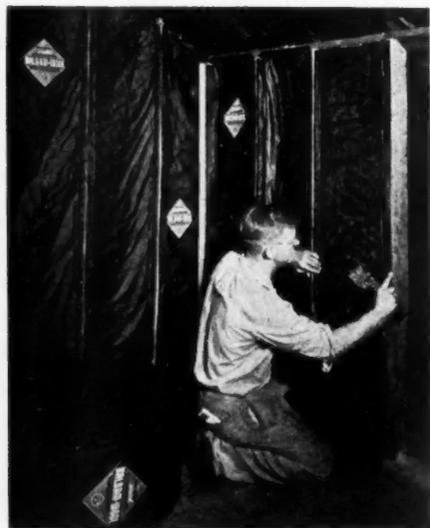
Wood fiber blanket insulation showing typical installation. Photo: Wood Conversion Co.
