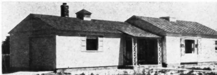
Improved concrete block sidewalls and concrete tile roof do the job here.
