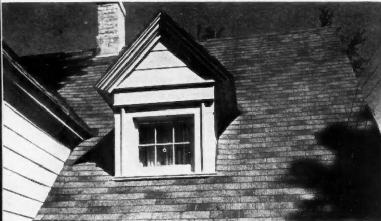
Typical asphalt shingle roof which can be applied in a wide variety of color combinations and designs.
