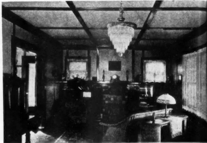
Example of fiberboard installation of the early '20's. Note how moldings contrast sharply with panels. Photo: Upson Co.
