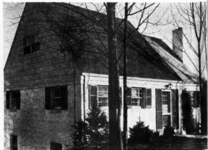
Recently developed and improved products shown here include asbestos shingles, asbestos siding shingles and waterproofed concrete block sidewall. Photo: Johns-Manville.
