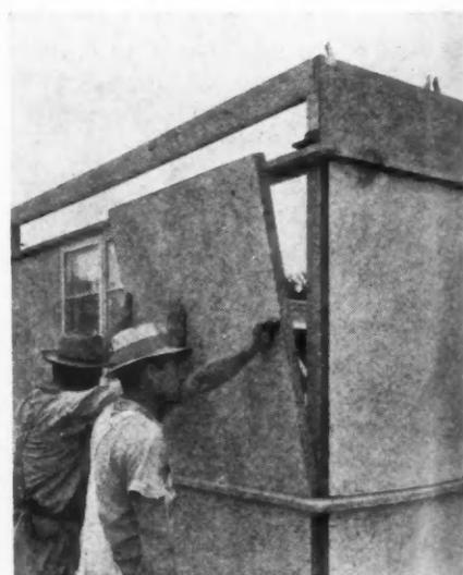
Single thickness wall material providing strength, insulation and finish. Photo: Calotex Corp.
