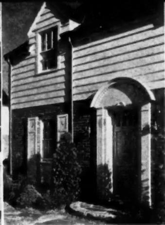
Combination brick veneer, wood bevel siding, slate roof and copper gutters.
