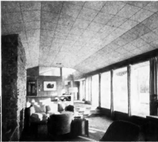
Insulating board tile ceiling job in modern solar heated home. Photo: Wood Conversion Co.
