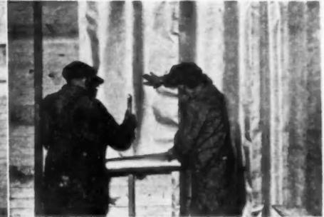
Flaked aluminum bonded to Sisakraft to form reflective insulation and vapor barrier.
