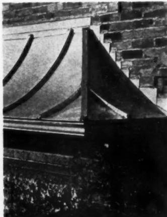
Typical example of standing seam metal roofing installed on garage entrance canopy. Photo: American Rolling Mill.
