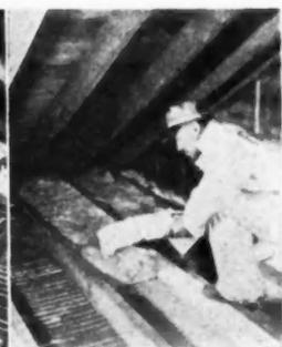
Left to right: Ceiling job with batts; roll blanket going in sidewall; recommended method of cutting roll blanket; ceiling application of blowing
