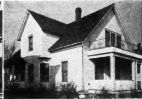
Flat asbestos-cement board covers sidewalls. Photo: The Ruberoid Co.
