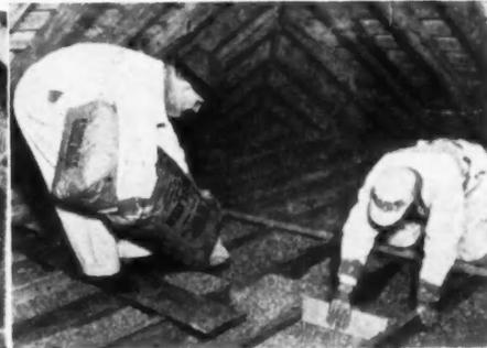
Use of vermiculite fill insulation in homes is on the increase.
