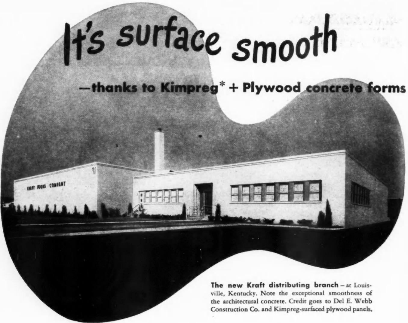
The new Kraft distributing branch — at Louisville, Kentucky. Note the exceptional smoothness of the architectural concrete. Credit goes to Del E. Webb Construction Co. and Kimpreg-surfaced plywood panels.
