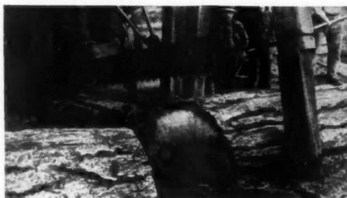
1. Only the finest fir timber is selected for processing at Peninsula . . . where skilled workers cut the huge "peeler" logs into proper lengths for the lathes.
