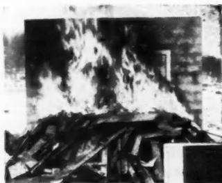
THE new door can be fitted and installed with ordinary carpenter tools. Photo at right shows fire demonstration of the door 14 minutes after the fire was started. Conventional panel door is at the left
