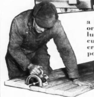
This one tool—the Model 60 MallSaw—does the work of many tools. Used as a hand saw, it will crosscut, rip or angle cut rough or dressed lumber, groove mortar joints, cut metal, cut or score tile, concrete and other aggregate compositions. When set in a sturdy, portable floor stand, it serves as a table saw—complete with rip fence and mitre guide; as a shaper for contour grooving, quarter round and tongue groove work; as a drum or face sander, as a wire brush, or as a grinder.
