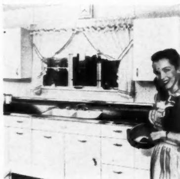
corners where back splash meets the flat top. The floor cabinets are bolted together and the tops joined with a watertight seal, giving a one-piece custom-built effect. This method of fitting tops makes the joints waterproof, greaseproof and dirtproof. Developed by the Midwest Manufacturing Co., Galesburg, Ill., this top is identified as their Kustomized Top.
