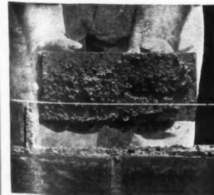
Thus the mortar will stick to the brick on top of it as well as to the brick below it.
