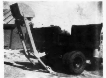
rear wheels on the loader's pads. No power take-off is required, and the truck driver may control the loading operation without getting out of the cab. It requires 10 seconds to fill one bucket and dump it in the truck. The loading device is called the "S-C Truck-Loader."
