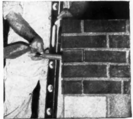
**BRIXMENT** mortar's extreme plasticity greatly encourages accurate bricklaying. Its higher water-retaining capacity also lengthens the time in which adjustments can be made, before the mortar has set. Once laid, Brixment mortar makes a stronger,
