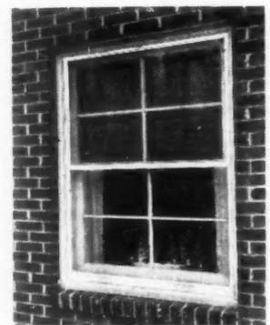
cause they mount close to the basic window. Because narrow-rolled 52S aluminum is used in the frames, they are thin enough to allow for screen or sash storage when not in use. A flat screw-type lock makes draft-free ventilation possible by holding the lower sash in any desired position.
