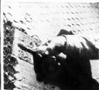
Plasterers like Keymesh because the surface is smooth to the trowel in any direction. Keeps its proper distance from the backing, insuring a "true" wall of even thickness.
