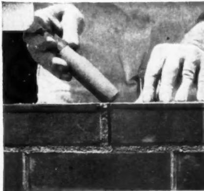
its position should never thereafter be changed. Shifting the brick breaks the bond between the brick and the mortar, and causes cracks in the wall.
