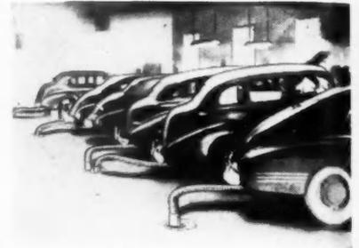
tion system, in a complete packaged kit, also includes a specially designed blower, and steel underground ducts; two double "Dial-O-Vent" floor assemblies, each capable of serving two cars at the same time; four flexible metal tubes to carry exhaust gas from tailpipe to floor vent; fabricated duct work necessary to carry exhaust gas to outside of building; roof flange and weather hood.
