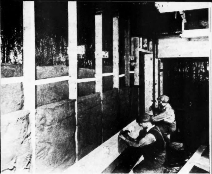
LEFT: Workman installing mineral wool in block form; at right, installing mineral wool in felt form
