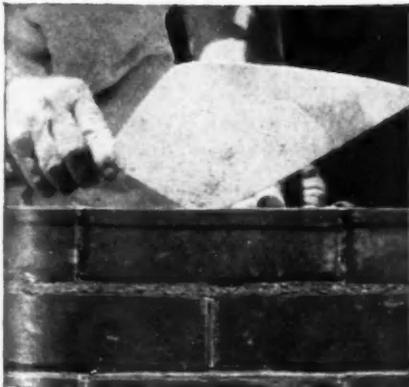
If a brick is not laid true to the line when originally placed, and if the bricklayer comes back and taps it into place later, cracks will result.
