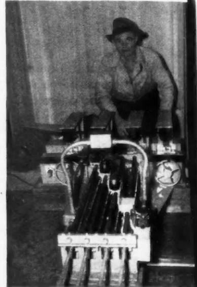
**ELECTRICAL CONTROL** for the spacing of edger saws is a typical Weyerhaeuser mill development toward greater efficiency.
