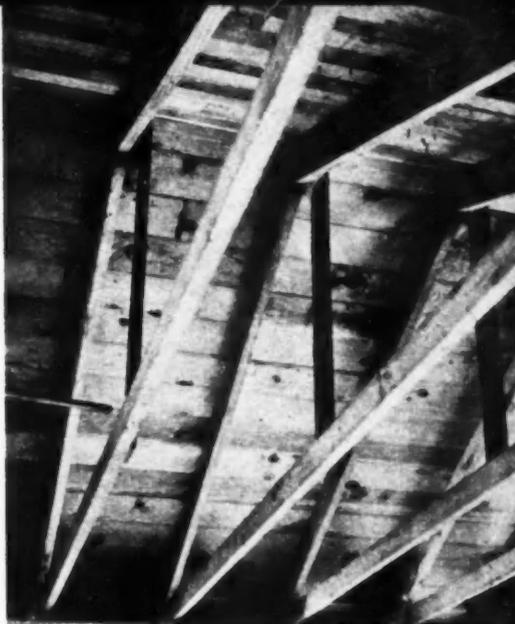
ROOF trusses for 16-foot span are fabricated on ground, raised in position
