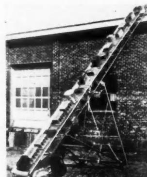
AB29143—Mulkey Portable Elevator. Sam Mulkey Co., Kansas City, Mo. Manufactured in four sizes. Easily maneuvered and placed in position. Adjustable to accommodate extensions. Balancing permits one man to handle and operate. Can be used for transporting all kinds of building materials. Savings in labor cut costs.
