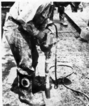
AB29377—Newest addition to the Mall vibrating line. Mall Tool Co., Chicago, Ill. A universal electric motor-driven, one-man vibrator for use in tight spots. Will place concrete fast and efficiently with a minimum of operator effort. The complete line of Mall power tools are subject of booklet offered free.
