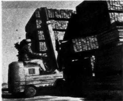
FORK-LIFT trucks move materials from storage yard into plant. Smaller loads are moved to fabricating points on dollies
