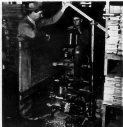
A SPECIALLY-BUILT drill press, designed by plant manager, bores holes in door for latch set in one easy, quick operation
