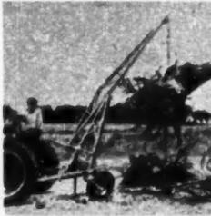
**AB2969**—CMC Handi-Hoist. Construction Machinery Co., Waterloo, Iowa. For lifting, loading, unloading or moving bulky, heavy equipment or supplies. Counterbalancing method utilizes weight of towing vehicle. Boom raises objects to height of 15 feet.
