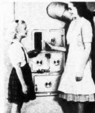
**AB29363—"Waste King" incinerator. Incinerator Products Co., Detroit 17, Mich. A packaged unit that installs in chimney base flush with wall. Will burn most waste with scrap paper for fuel; is provided with gas hook-up for wet loads. Of welded construction, has cast iron grates and doors, is thoroughly insulated.**
