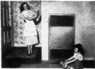
**WALL FURNACE**—Registers on both sides of the partition. 42,000 BTU. Output.
