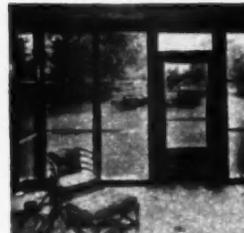
AB29322—Sliding ultra-violet glass panels with Lumite plastic screen. Self Storing Window Co., Inc., Minneapolis, Minn. Three channel jambs permit two-thirds open area at three levels. Optional door location. Glass areas set in rubber. Five sizes.
