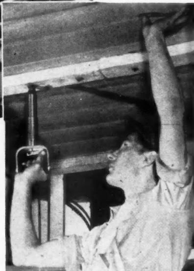
spring-loaded safety arm and holds it in position. If the tool is dropped the safety arm instantly pulls the firing pin out of reach of the cartridge. The stud is discharged when the barrel is held solidly against the material and pushed in sharply.
