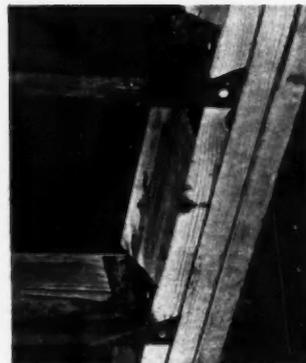
AB29167—Trip-L-Grip framing anchors. Eliminate toe-nailing in light wood frame construction. Recommended to home builders as joist hangers. Made in three types, both right-hand and left-hand, making six in all. Special nails are furnished with anchors. Product of the Timber Engineering Co., Washington 6, D.C.
