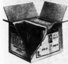
AB29319—Quality house unit package. Sargent & Co., New Haven, Conn. Lock and latch sets for two average small homes contained in one unit package. Inside master carton, lock and latch sets packed as complete house units. Are all suitably labeled.
