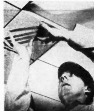
AB29381—Certile, incombustible acoustical tile. Certain-teed Products Corp., Ardmore, Penn. Fine strands of inorganic, flexible glass fibers, superimposed in crisscross fashion offer high degree of sound absorption. Tile has high insulation value. Not affected by changes in the weather. Will not rot or decay.
