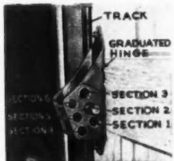
AB29314 - Raynor Graduated Seal for Up and Over wood sectional doors. Raynor Manufacturing Co., Dixon, Ill. Used in conjunction with tapered track. Seals each section of the door against jamb or molding when the door is in a closed position.
