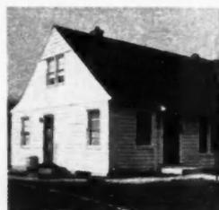
AB29345—Unit Construction. Unit Structures, Inc., Peshigo, Wis. Production-line techniques, mass purchasing, modern factory methods in conventional construction. Many interior, exterior layouts. Number of rooms and room sizes varied with house.
