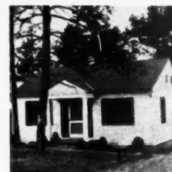
AB29272—Factory-built homes. Knox Corp., Thomson, Ga. Dimensions, 24 feet, 8 inches by 32 feet, 8 inches. Four rooms. Panels, cut to exact dimensions, are assembled on jigs to supply basic structural components. Three floor plans are available now.
