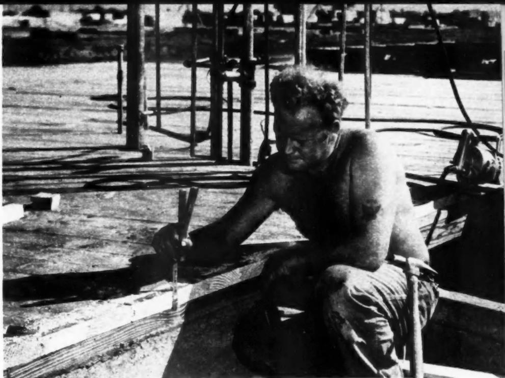
**ONE BUILDER** uses tongue and groove 2x6 sub-flooring over 4x6 girders for his floors
