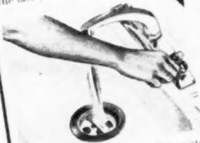
**3. Turn on cold water.** This automatically starts the Disposall action. Food waste is shredded into tiny particles, flushed into sewer or septic tank. The Disposall works perfectly with either sewer or septic tank.
