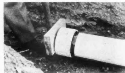
PUSH coupling over pipe with twisting motion. Then using rod and block of wood, push coupling firmly into position
