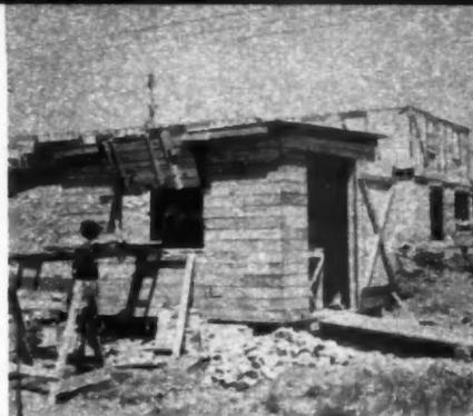
LEFT: One of the three portable sheds which house gasoline-powered saws, moved about the site to do heavy precutting. Right: Several of the forms used to precast concrete porches and steps, that would ordinarily be poured on the site. A porch section weighs about 2,300 pounds and is handled by heavy power equipment by use of special suction cups. A blast of compressed air releases units from forms
