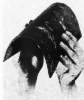
**AB29205**—A flooring material named Terraflex. Johns-Manville Co., New York, N.Y. is extremely flexible. Slightly heated, it can be curved to form stair nosings and coved bases. This quality permits floor to conform to any uneven surfaces and provides unusual resilience and comfort under foot. Offered in varied colors.
