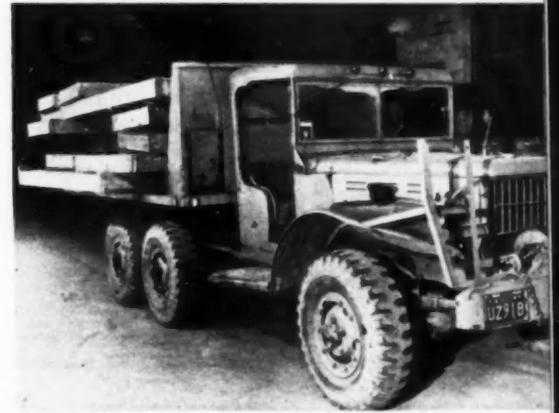
SEVEN 6-wheel drive trucks with winches are used to transport finished sections of houses from the plant to job site
