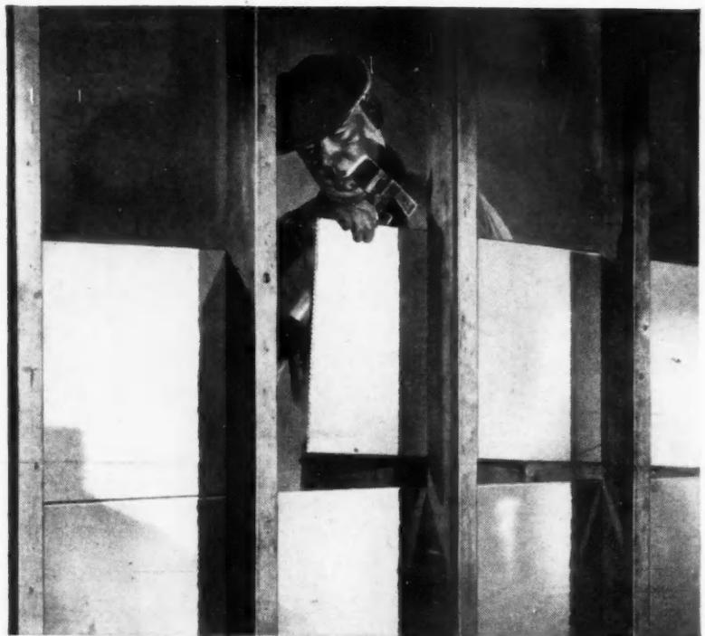
INSTALLING plain gypsum with a sheet of aluminum foil on back side making it resistant to vapor transmission and giving heat insulation equal to 1/2-inch fibre board
