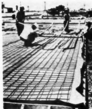
AB29165—Waterproof reinforced paper named Sisalkraft. The Sisalkraft Co., Chicago 6, Ill. Applied over fill in radiant heated floor job, as illustrated, it prevents small fingers of concrete from dropping down into the fill. These fingers carry moisture and cold up from ground into the concrete. Sisalkraft protects floor.
