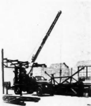
**AB2997 - Hydrocrane.** Bucyrus-Erie Co., South Milwaukee, Wis. Model H-3, 3 ton, 3/4-yard is fully hydraulic in operation. Boom telescopes and hoists hydraulically; load hoists hydraulically; deck revolves hydraulically; outriggers are set hydraulically; bucket digs hydraulically. Safe system. Simple to maintain and operate.
