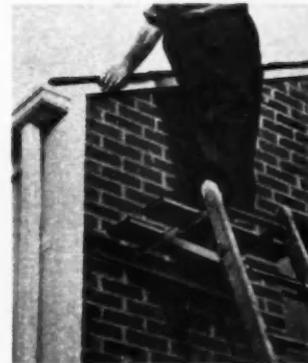
AB29369—Safety ladder stage. Juniata Co., Huntingdon, Pa. Designed for use with extension ladder. Provides a safe working area of 26 inches by 24 inches. Weighs less than 9 pounds, is completely portable, easy to handle. Footboards are of seasoned, waterproof wood, slotted for easy width adjustment.
