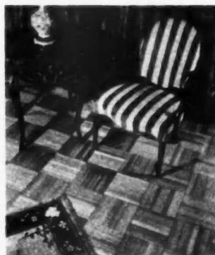
**AB29191—Hardwood flooring** made in squares that fasten to gum without nailing and create a parquet effect. Newcastle Industries, Inc., 300 West 54th St., New York 19, N.Y. Apply over concrete sub-floors or over radiant heating in concrete sub-floors or over old floors. A square foot can be laid each minute.
