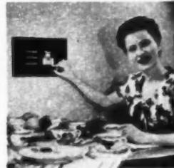
**AB29244**—Flush Wall radio. Flush Wall Radio Co., Newark, N. J. For kitchen, bathroom, playroom, bedroom. Wall becomes part of speaker-baffle. Five-tube, AC-DC. Adjustable slotted hinges attached. Steel box with single receptacle, 6½x9½x3½ inches.
