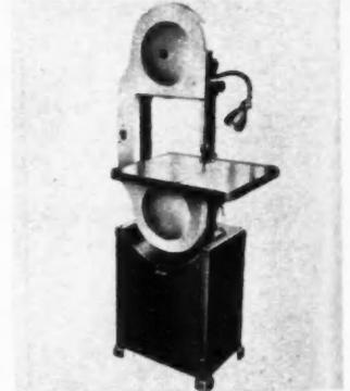
**AB29222**—H & A 14-inch band saw. Heston and Anderson, Fairfield, Iowa. Designed to permit operator 45 per cent more working area and 33 per cent more vertical clearance. Has 20x23-inch tilting table with 12 1/2 inch vertical and 13 3/4 inch horizontal clearance. Durable construction assures long life for band saws.
