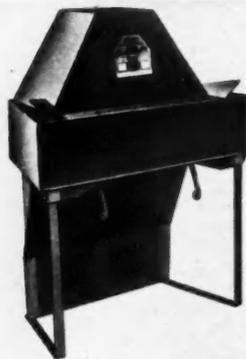
AB29112—Fresh-Aire fireplace unit. Bennett-Ireland, Inc., Norwich, N.Y. Unit is hidden within the masonry of conventional fireplace. Does not interfere with fireplace design. Fresh air from outdoors is heated and circulated throughout room. No loss of heat up the chimney. No cold floor drafts or smoke with the unit.
