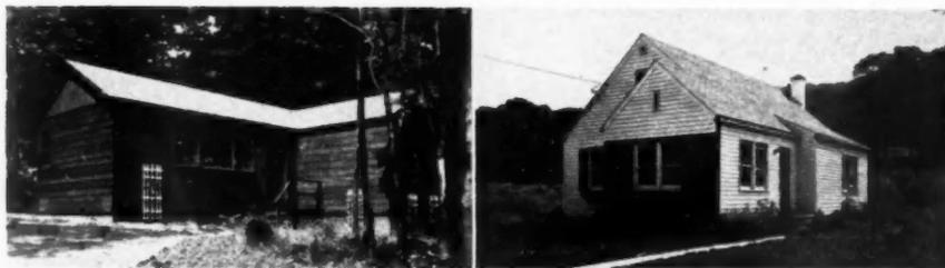
EXTERIORS are finished with stone veneer, wood siding, asbestos shingles and other materials. Space is available to add two extra bedrooms in the future. Heating ducts run to the attic and are capped so that heating can be conveniently connected. Interiors are dry wall construction. Prefinished oak or maple floors are used
