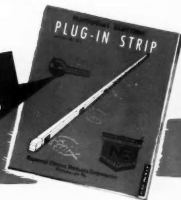
You'll like this revolutionary multi-outlet assembly too. It gives you a S-P-R-E-A-D of electrical outlets —spaced every 6" or 18" apart.
