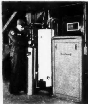
**AB29106—Culligan soft water service unit.** Culligan Zeolite Co., Northbrook, Ill. Soft water available on a service basis. Unit is installed to supply water in home. Exchanged by company service man at regular intervals for another unit of freshly regenerated zeolite. A monthly charge made for service.
