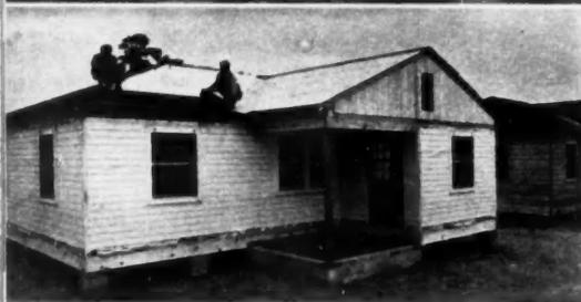
**AFTER** subfloor is laid, erection of various Crawford-Built house sections can be accomplished with few men in short time
