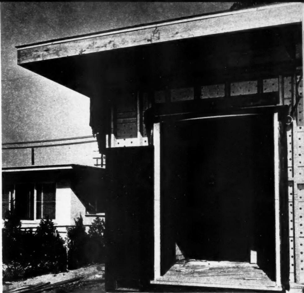
**SHEATHING** is rarely used on houses in California. Stucco is a popular exterior finish and is applied directly to studs over felt paper and chicken wire for reinforcing
