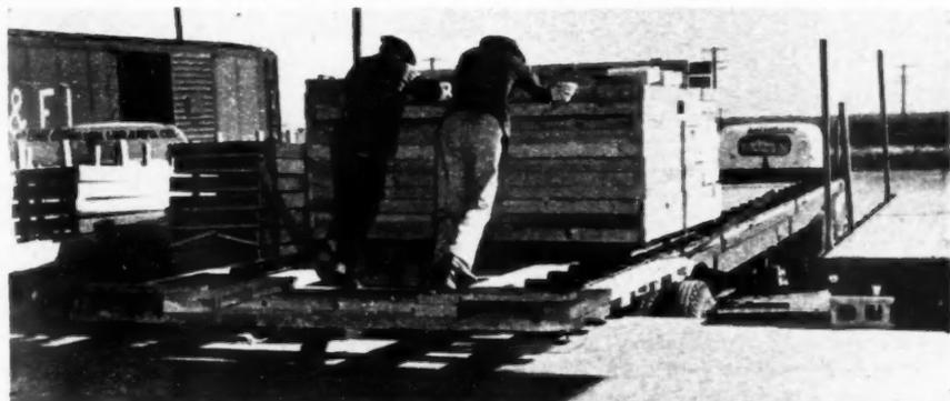
A SPECIAL roller conveyor arrangement makes it easy to load completed house sections from the fabricating plant to a truck with special roller-conveyor equipped bed
