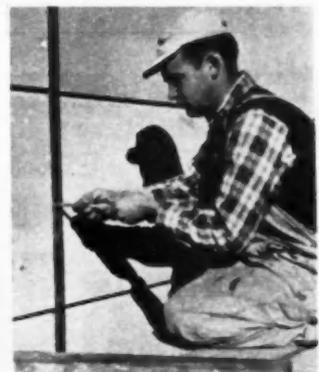
AB29118—Modular building units. Durisol, Inc., New York, N. Y. This material provides insulation, fireproofing, sound absorption and structural rigidity. It is a lightweight, precast concrete slab moulded in special shapes and sizes for sheathing and exterior veneer. Building time is cut through use of slabs.
