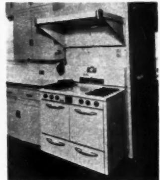
AB29161—New range ventilating hood for the modest home. Vent-A-Hood Co., Dallas 9, Texas. Hidden tube light across inside front provides indirect lighting of hood and range. Patented "magic lung" separates steam and grease before forcing heated air outside. Finish is baked enamel in white and colors.
