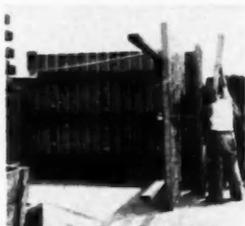
AB29359—Atlas Speed Forms. Irvington Form & Tank Corp., Irvington, N.Y. Concrete forms for foundation, four walls, inside and outside, may be picked up by crane when concrete is set and walked to next site, ready for next pour. Use 300 times.
