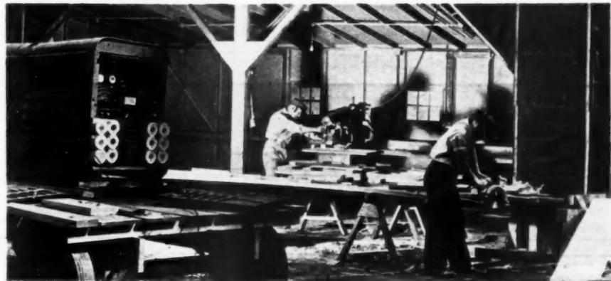
TWO LARGE portable generators on trucks were used to run total of 18 power saws. At this shop, centrally located in Sunset Park, precutting made greatest time-saving
