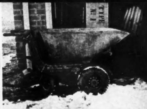
**POWER wheelbarrow is popular with laborers, bulider reports. Scoopmobile speeds handling of foundation excavation and loading of other earth material. Large concrete mixer, two jeeps also are used**
