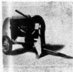
AB29294—Muller plaster mixer. Muller Machinery Co., Metuchen, N.J. Six cubic foot capacity. Driven by Briggs & Stratton engine through heavy roller chain drive. Equipped with bag shelf and bag splitter. Telescopic towing bail provided.
