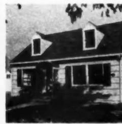
AB29255—P&H prefabricated houses. Harnischfeger Corp., Houses Div., Port Washington, Wis. One-story, 24x32 feet, two or three bedroom, with or without basement. Living room, 11 feet, 7 inches by 17 feet, 4 inches. Panelized and insulated throughout.
