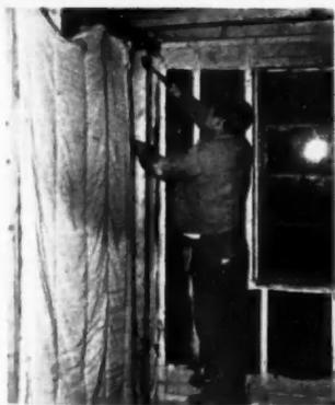
**AB29215**—Cellulite cotton insulation for soundproofing. The Gilman Brothers Co., Gilman, Conn. Produced in blankets for use as sound deadener. Installation simple. Blankets are hung by weaving in and out between studs. In a staggered-stud test wall, 3-inch Type E Cellulite cut passage of sound to whisper.
