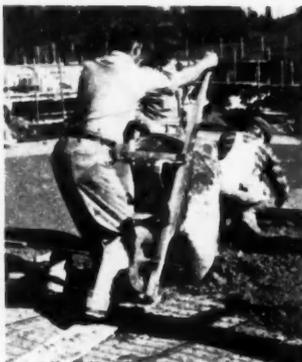
AB29196 — Pittsburgh Steeltex for floor lath. Pittsburgh Steel Products Co., Pittsburgh, Pa. Offers structural advantages and economies in light-slab concrete floor and roof construction. Gives maximum reinforcing value and facilitates proper curing of concrete through maintenance of water-cement ratio.
