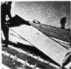
AB29265—Monel sheet for roofing. The International Nickel Co., Inc. New York, N. Y. May be cut, formed, joined and soldered into standard roofing parts with regular tools and methods. Nickel-Copper, .018-inch thick, corrosion-resistant.
