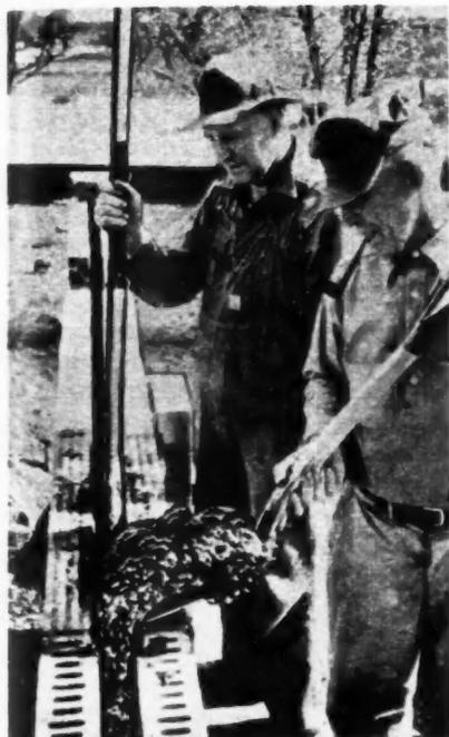
POURING and rodding vermiculite insulating concrete in a 10-inch tile cavity wall
