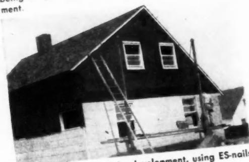
One of the houses in the development, using ES-nails to apply shingles to insulation sheathing.
