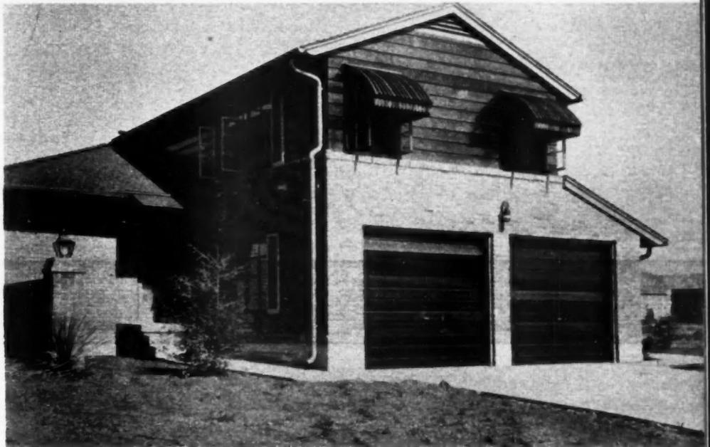
**UPWARD** acting garage doors, of redwood, were made on the site by Holaday workmen. Attic ventilation louvers are metal
