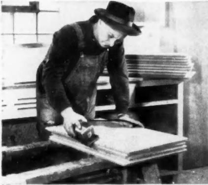
Chamfers and rounds must be thoroughly sanded when using plywood to give a smooth surface for the finish coat and to prevent strip-back of the outer veneer. For this operation a 120-grit aluminum oxide open coat cabinet paper is used. The Century should be held parallel with the edge to be sanded. Orbital motion of the pad will prevent chipping of the veneer.
