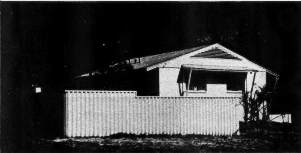
**CORRUGATED** asbestos-board fence (left) makes convoluted wall around back yard. Material is lightweight, easily installed and fireproof. Fence is not included in house cost. Section below shows construction details of roof trusses, walls and foundation. Placement of cabinets in relation to over-all planning of house is also indicated
