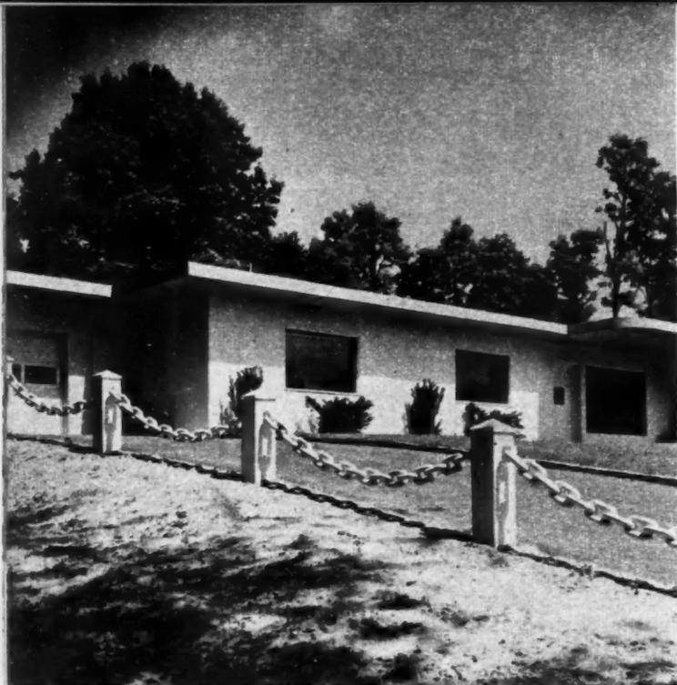
**LINKS** in decorative chain fence are of reinforced concrete. Process is patented by Charles Fontana, specialties manufacturer
