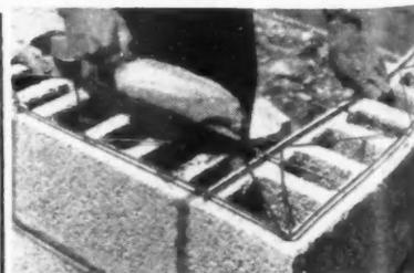
It's NEW . . . It's NEWS! Now you can have the protection of steel reinforcing in masonry walls economically. DUR-O-WAL prevents costly cracks . . . protects building investments. Available for the various wall thicknesses, DUR-O-WAL is designed for quick and easy laying in the mortar joints. Inquire about DUR-O-WAL today . . . be among the leaders who are building for the future. Write . . . wire or phone DUR-O-WAL Division, Cedar Rapids Block Co., 664 12th Ave. S.W., Cedar Rapids, Iowa.
