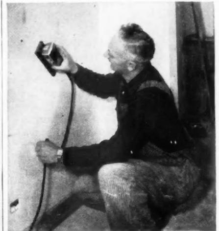
Dry wall taped joints and rough plaster are sanded smoothly and uniformly with the new Century. Ordinarily this type of work runs high in cost because of the time required for the necessarily smooth finish, but the Century, loaded with a 150-grit open coat paper, does it with speed, precision and economy.
