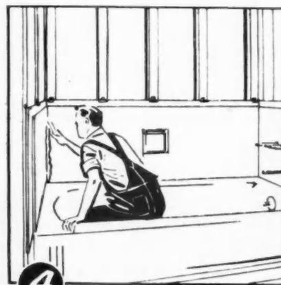
**4** Clean glass and fill joints carefully with the pointing compound supplied. This assures a thorough waterproofing installation.
