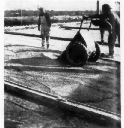
BY laying the insulating concrete in alternate panels, workers were enabled to work alongside the sections being poured
