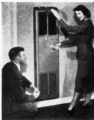
conserved and floor furnaces are impractical. Input rating, 25,000 B.T.U.'s, and warm air flow, 8,000 cubic feet per hour—enough to heat two average rooms. Front panel measures 14 inches wide by 61 5/8 inches high. Casing extends into room 3 1/2 inches. Meets all requirements of American Gas Association. The Coleman Co., Inc., Wichita 1, Kans.
