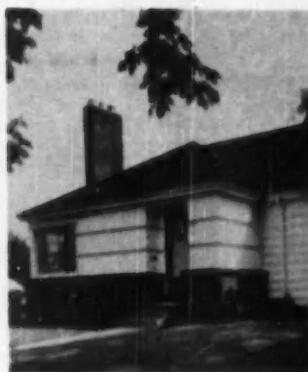
THREE wide horizontal strips of plywood above window-height stone resulted in this pleasing combination. Painted wood molding covers the horizontal plywood joints
