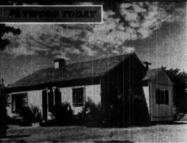
A MODERN prefabricated house with fir plywood as the basic material inside and out. Prefabricated housing was given tremendous momentum with the development of fir plywood, which made rigid panels possible
