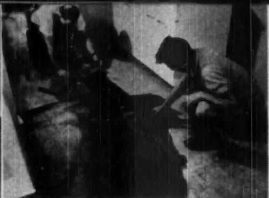
THICKNESS of plywood panels for subflooring varies with type of job. The  $\frac{1}{2}$ -inch panels meet all structural requirements
