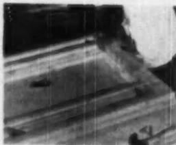
fittings and metal plates hold wires in permanent alignment. Face sheets of Maine birch veneer provide attractive appearance, while patented fibre core prevents waviness or ripple from showing through surface. If necessary, door can be adjusted to conform to misalignment that may occur in buildings after door is installed. Kenno-bac, Inc., Truss Door Div., Bingham, Maine.
