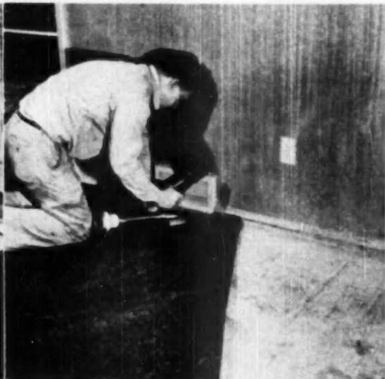
AS A BASE for linoleum or other floor coverings, the smooth, sanded Plypanel or Plybase grade plywood is used over Plyscord (unsanded) subfloor or a single layer of thicker Plypanel or Plybase is installed as a combination subfloor under-lay under linoleum or other coverings
