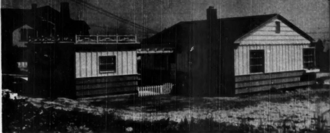
ABOVE the three courses of shakes here, the exterior is all plywood. To simulate plank siding, 1/2-inch molding was nailed at 12-inch intervals over the plywood panels. The gable ends are plywood with the same 1/2-inch molding applied horizontally
