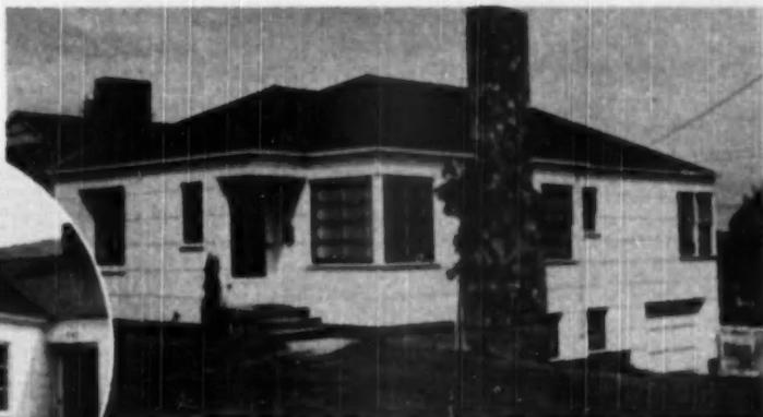
TYPICAL example of effective exterior that can be achieved when wide plywood lap siding is used on a small, low-priced house
