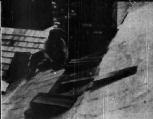
ROOF decking not only goes on faster when plywood sheets are used, but rafters may be spaced further apart for further saving
