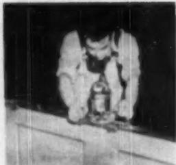
and firm's hinge assures good hanging doors because doors are held by the recess and not by the screws. Screws simply hold hinge leaf in place. Same templet, same setting and router are used in cutting recess in jamb. Threading on motor casing allows adjustment of 1/16-inch for each complete turn of the motor. Stanley Electric Tools, New Britain, Conn.
