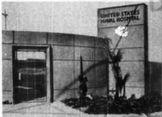
PLYWOOD forms used for curved fence with paneled effect
