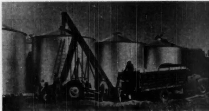
MORE than 8,000,000 bushels of capacity in all-plywood grain bins was purchased last fall by the Commodity Credit Corp. They were fabricated by more than a dozen firms in a variety of shapes and capacities. Those above are the large round type.
