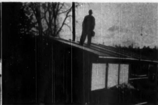
DRAFTINESS in farm buildings is held to a minimum when large panels are used because there are fewer wall joints
