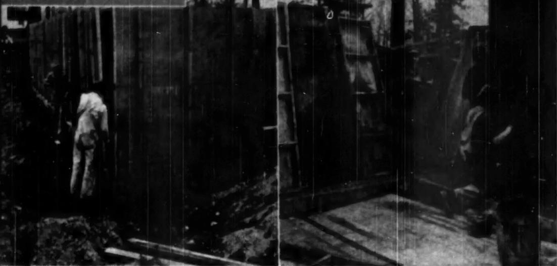
It is common practice for home builders to use the sheathing grade of plywood for forms and then re-use it in the structure
