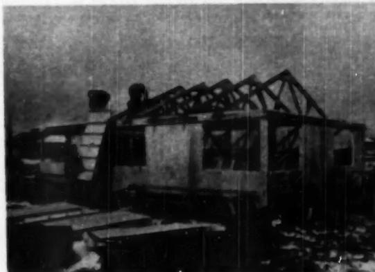
**PRECUTTING** and preassembly of house parts in on-site operations, made possible largely because of plywood, have been a tremendous factor in the huge volume of fully engineered houses produced by the industry
