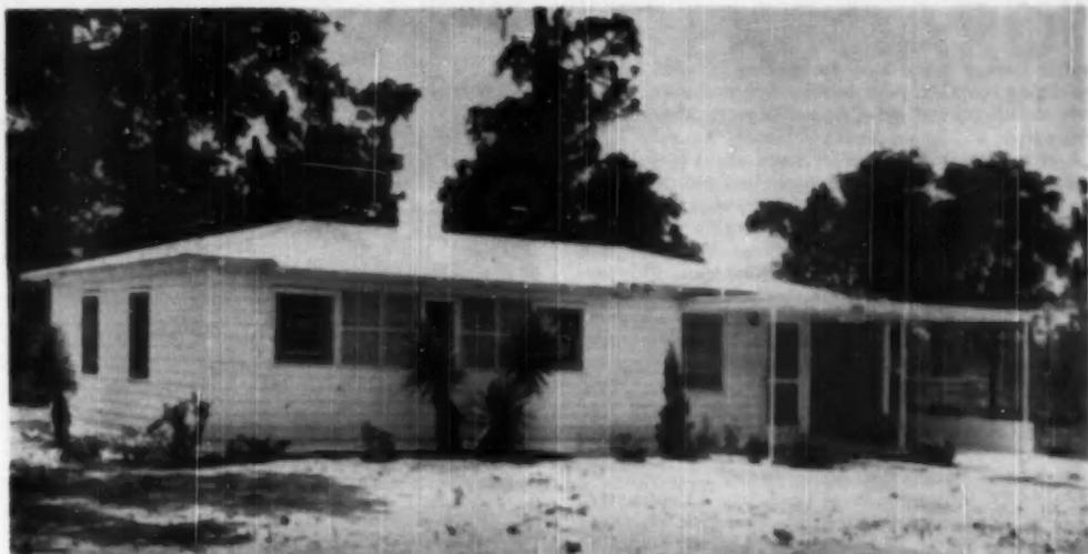
THE "Cabinet Wall" house introduces the free use of interior space by means of an exterior structural shell and roof trusses
