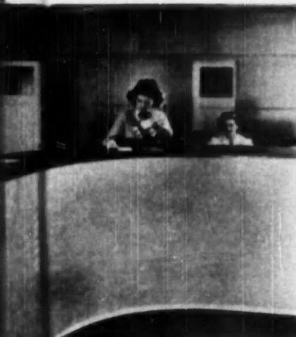
PANELING with plywood permits curved surfaces where desirable. In developing curved surfaces, the panel to be bent is usually fastened flat, and the flat surface then fitted to it. The use of continuous, rounded backing makes best job
