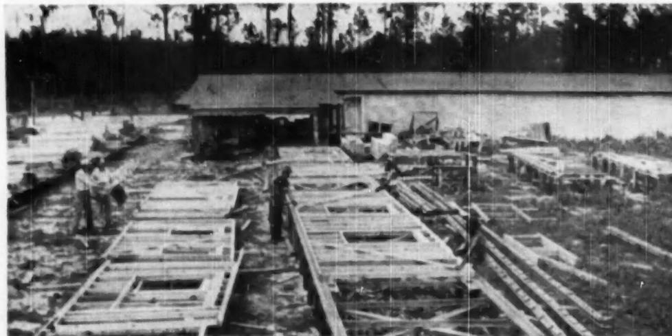
ASSEMBLY yard in back of warehouse and office showing jigs on which complete wall units are constructed ready for erection
