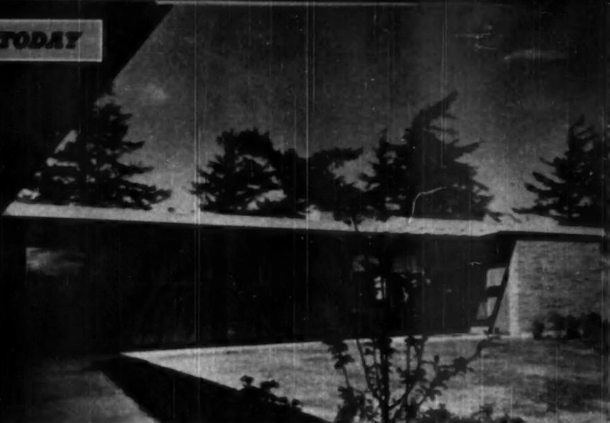
PLYWOOD has answered the requirements of designers wishing to achieve wide, smooth-underside overhangs on contemporary houses. Although this area is somewhat protected from the weather, only the exterior type of plywood should be used
