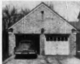
panels ¼-inch thick. Of dowel pin construction, with two ½/2-inch oak dowel pins to each joint. Door sections come in equal widths and are specially rabbeted so that rain and moisture will drain out instead of remaining in the joints. Doors are shipped in a crate with hardware and cable. Track and springs are packed in a second crate. Doors are toxic treated with a solution approved by the N.D.M.A. Installed, the doors offer finger-tip lifting. National Manufacturing Co., Sterling, Ill.
