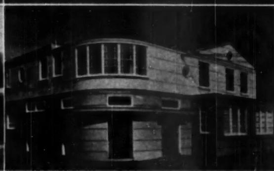
PLYWOOD has gained wide recognition as a versatile and permanent structure material for small commercial structures. Some examples are shown here. (1) All-plywood exterior in combination with glass block and large areas of plate glass. (2) Wood molding was used to em-
