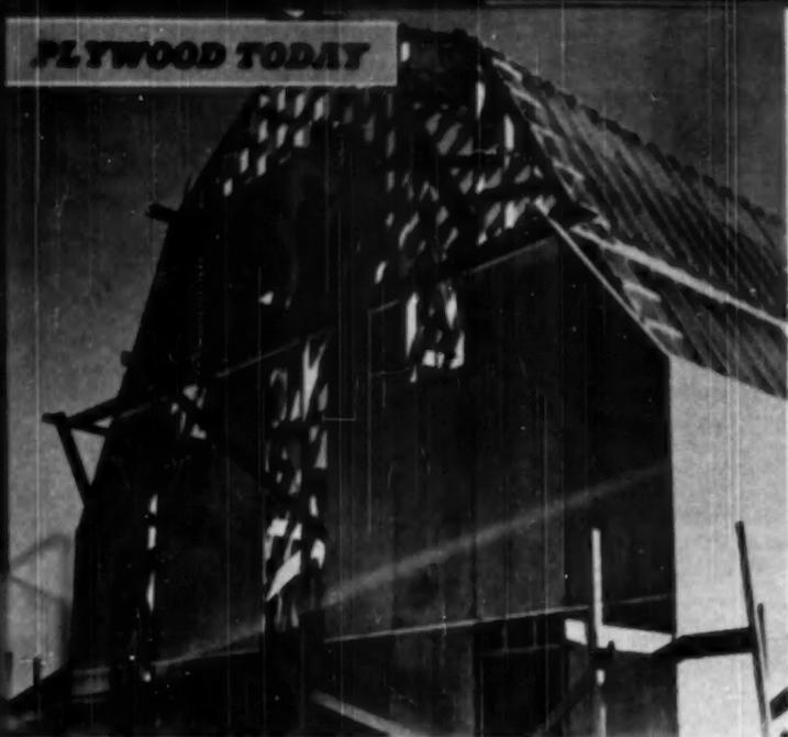
BECAUSE of high humidity conditions in farm buildings only the exterior types of fir plywood with waterproof adhesive bonds should be used
