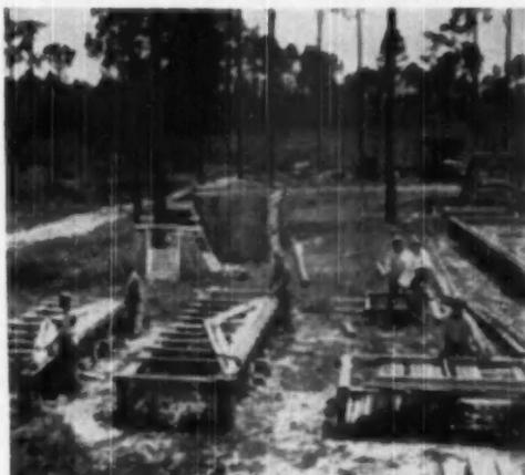
PORTION of assembly yard on building site where trusses are fabricated on jigs. Units are stored as shown until used on the job
