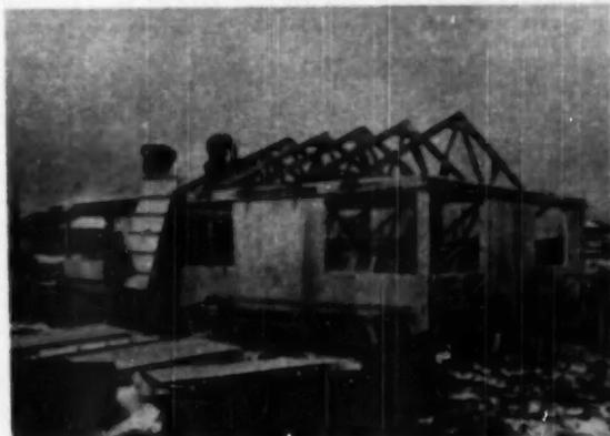
**PRECUTTING** and preassembly of house parts in on-site operations, made possible largely because of plywood, have been a tremendous factor in the huge volume of fully engineered houses produced by the industry
