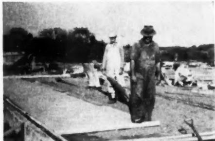
**VAPOR** resistant paper is placed over the leveled fill. Heavy rigid type insulation is placed around outer perimeter of slab
