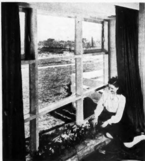
▲ **ANOTHER VERSION** of a window wall arrangement shown above with hinged units confined to upper tiers of lights. Brick planting area at sill of window on the exterior is repeated in the same position on the inside of living room, thus creating the illusion of planting box being continuous. Board valance at window head conceals the rod for draperies
