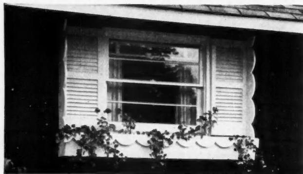
◀ **DESIGN FEATURE** particularly adaptable for kitchen windows that occur above counter or sink. The scroll treatment used as a crowning member for flower box is repeated in the vertical boards that enclose the extreme ends of wood blinds. This unit is used effectively where roof soffit is at top of casing
