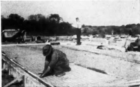
**REINFORCING** wire mesh is laid over the paper before the concrete is placed. Specialized crews handle all the concrete work
