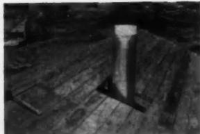
OPENING in roof larger than Vitroliner casing provides attic ventilation through flue housing and under chimney cap.
