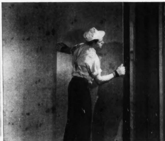
**BIG, STURDY PANELS** of Gold Bond Grain board can be nailed to wood framing or right over old material. They make the job go fast and help keep costs down!
