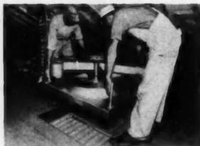
**Low-Cost Installation**—This photo shows how easy it is to install the automatic shutter models. Fan unit is simply placed over the ceiling opening . . . no fastenings needed. Shutter unit fastens to frame around ceiling opening.
