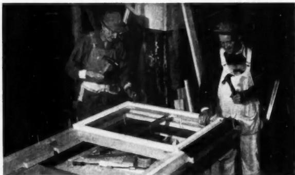
**A HANDY** jig in the Place mill is used to frame aluminum windows. Framing members become the finished jamb in Place homes resulting in cost economies
