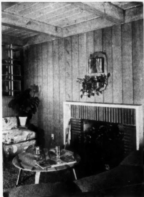
FLAT ROOFS permit exposed beams and boards in living room
