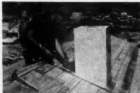
**RAIN CAP** is welded to housing top. New units have added welded-on baffle ring around cap
