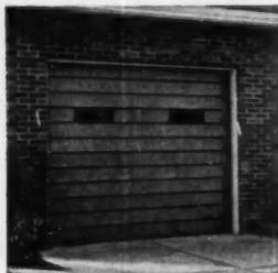
New 9x7-foot Morrison Roly-Door, a four-sectional steel, upward acting garage door, operates completely within the garage. Perfectly balanced in any position, it is quiet, safe and effortless, with no protruding obstructions to catch clothing or auto bumpers. New 9x7-foot door and the Standard 8x7-foot Roly Door are adaptable to a 6-foot 6-inch-high opening where ample headroom is available. Morrison Steel Products, Inc., Dept. AB, Buffalo, N. Y.
