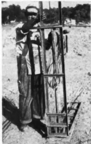
**BENDING** perfect 90-degree angles in reinforcing rods is easy with this device made by Place and Company men. The rods are used at corners of concrete slab floors
