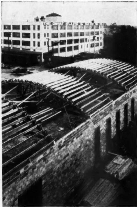
LAMINATED bowstring trusses form the roof of this warehouse
