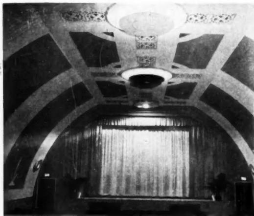
**ARCHES** form interior curved surface, covered with insulation board
