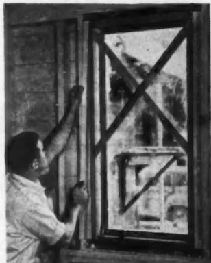
**3 ATTACH INSIDE PINS** — To complete the installation, apply the inside metal fins at head, sill and jambs. Fins fit under the lip of the steel frame and are nailed to the studs. This insures a tight weathertall all the way around the window.
