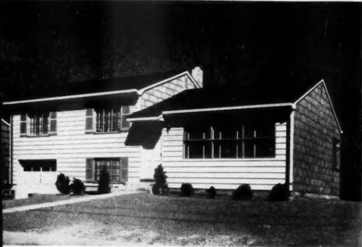
**SPLIT-LEVEL HOUSES** are particularly adaptable to sloping building sites where floor levels are made to conform to existing grades. Roof surfaces are varied in this type house
