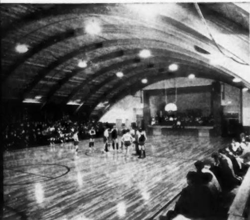
SCHOOL gymnasium with clear floor area 70x88 feet. Roof is constructed with wood laminated beam arches
