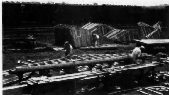
**GABLE** ends are completely assembled at the yards before they are hauled to the building site. All roof rafters are precut in shop and assembled at site
