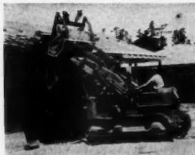
**ROOFING-SPEEDUP** on this 100-home project near North Bend, Ore., is achieved with Allis-Chalmers HD-5G Tractor-shovel. Special home-made fork designed by Bower-Edmonds Corp., Portland builders, enables tractor to hoist a half-load of 16-foot sheathings and a bucketful of asphalt shingles in one operation. Machine is also used to backfill basements, level yards and, with trench-hoe, dig sewer trenches
