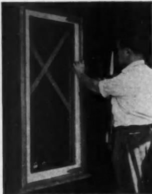
**2 ATTACH OUTSIDE PINS** — Next, attach metal fins at jambs. The grooved edge of the fin fits over the edge of the steel frame. The flat surface of the fin is nailed to the sheathing. Exterior trim can now be applied.
