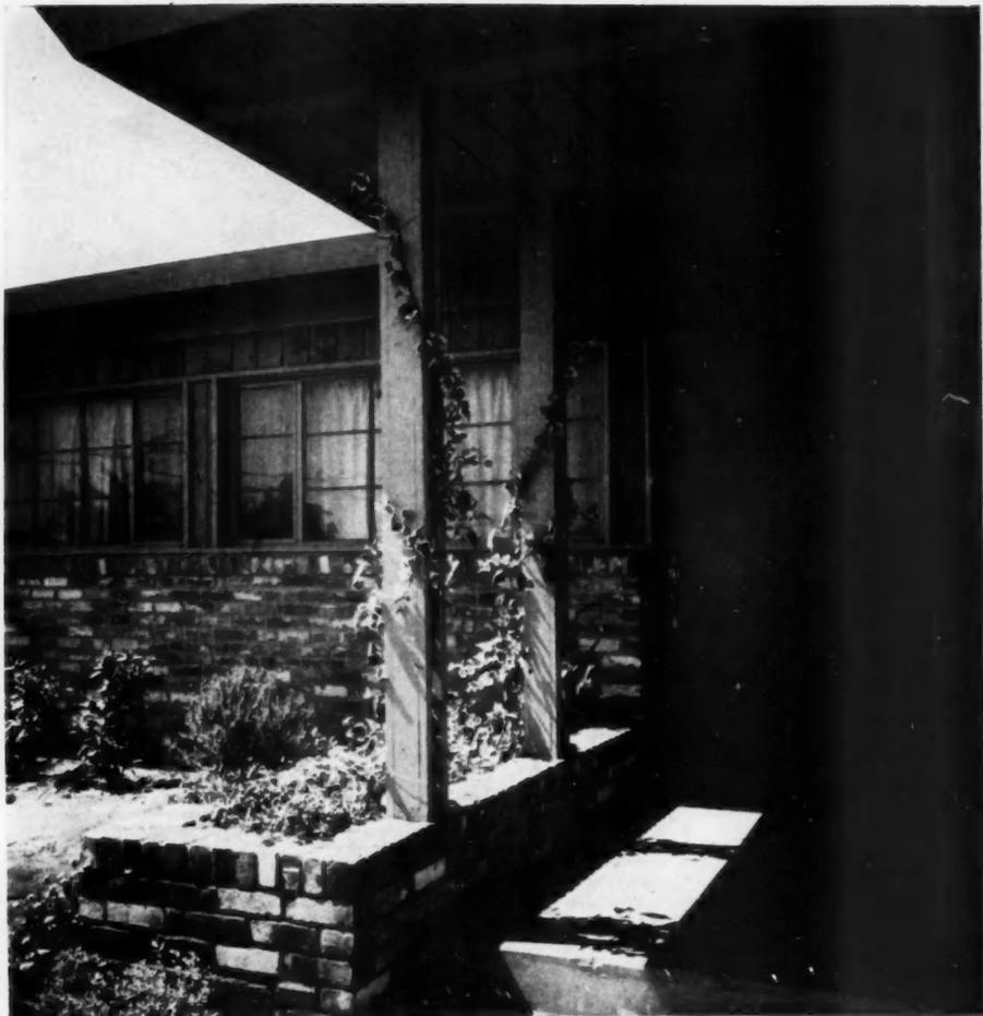
PARTICULAR emphasis is placed on entranceways by Jere Strizek. Note exposed boards and beams in overhang of flat roof
