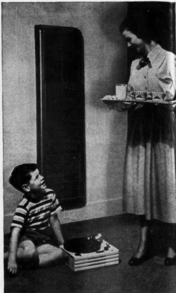
Today install the Heater of Tomorrow — Coleman's compact Wall Heater that's a natural for the low-cost small-home market. It's no problem to install these heaters because they fit right in the wall, extending out only 3 3/8 inches. The Single Wall Model illustrated above fits between standard studs.
