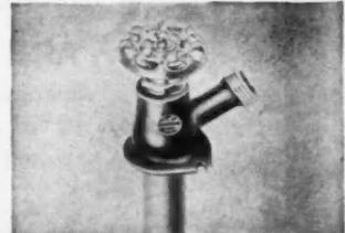
A non-freezing faucet which provides outside running water the year around despite freezing temperatures, is the J-K Non-Freezing Outside Wall Faucet made by the James Knights Co., Dept. AB, Sandwich, Ill. The faucet is operated by the handle turning off a valve inside the house. A notched flange on the faucet permits easy anchoring to frame buildings. Models are currently available of galvanized pipe as well as of all brass and copper construction.
