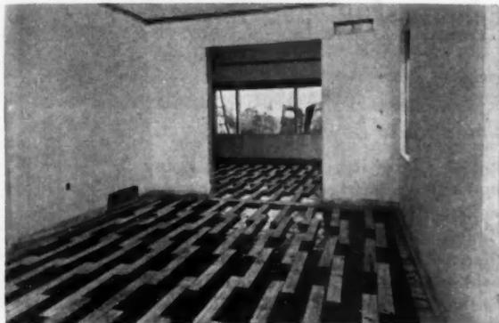
**SIMPLIFIED METHOD:** T & G strip hardwood flooring is applied to these staggered sleepers imbedded in mastic on slab and grooved strip hardwood flooring to sleepers imbedded in mastic on top the concrete slab.
