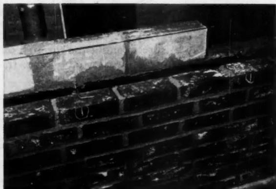
IN BUILDING this test wall the mason has taken the necessary precautions to smooth out the mortar squeezed out of the joints in the cavity
