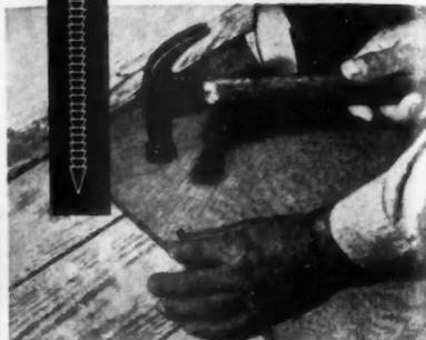
To make your linoleum underlays hold tightly and lay flat permanently, secure them with Hassall annular-threaded linoleum underlay drive screws. They are cement-coated for maximum gripping power. Heads are flat countersunk type. Size: 1/4 x #3 ga. State quantity when writing for prices to:
