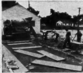
**CARPENTERS** build kitchen cabinets on the job in all Eclipse-sponsored units. Truck driver watches as crew spreads ready mixed concrete for slab floor
