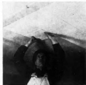
Tile is applied to ceiling, starting at center with temporary straight-edge nailed up for a guide
