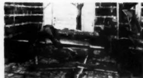
Concrete mix poured over membrane should be dry. Planking protects ducts when pouring
