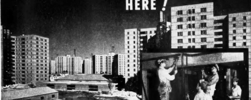
Many thousands of dollars were saved by the modern DRIVE-IT powder operated fastening method used on the Park LaBrea project in Los Angeles. Over 750,000 drive pins fastened metal lath to concrete ceilings and floors from which wall partitions were secured.
