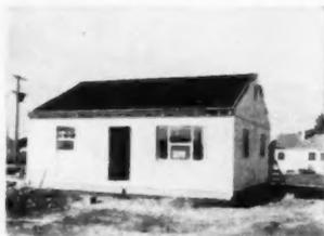
**RAISING THE ROOF.** Peak formed by two sections placed together. Gable ends are then hoisted into place
