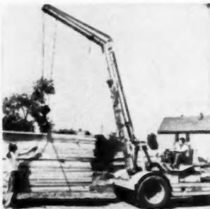
**LIGHT MOBILE CRANE** is versatile tool for loading and unloading, for erection of steel and panels
