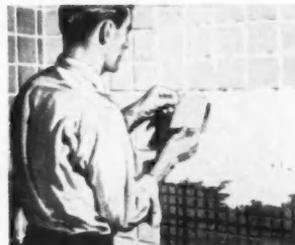
**FIG. 20**—Tiles are pressed into the grooves of the foundation board
