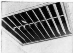
GRILLE or louvre for ceiling fan is a typical installation. Similar metal louvres are also popular in doors to control drafts and room ventilation
