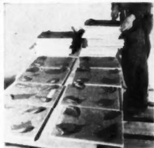
Application of cement to back of tile is first step in this method of applying tile to ceiling
