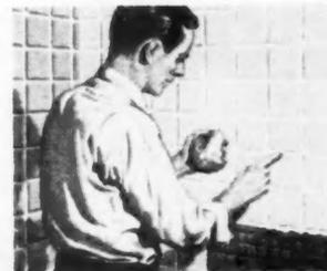
**FIG. 21**—Excess adhesive is removed and the joints are pointed with a finger. The tiles are then cleaned with a sponge dampened with water or mineral spirits
