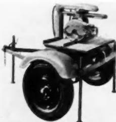
THE RADIAL SAW finds use in rafter notching, cutting joists and studding, making forms, and many other jobs. Trailer-mounted units are available for easy transport from job to job
