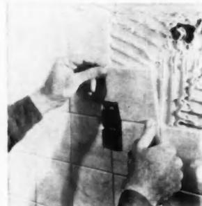
**FIG. 16**—How the tile is set around socket
