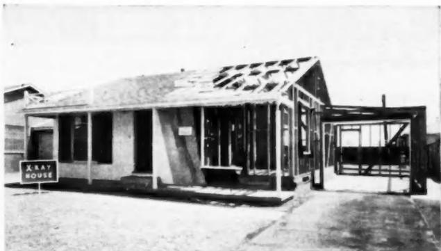
This builder uses what he calls an X-Ray house which has sides, sheathing, and other portions cut away to show details of construction, plumbing, heating and wiring installation and other features. Customers like to know what they are buying and appreciate this type of demonstration.
