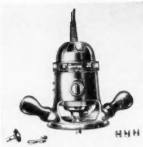
**HAND ROUTER** to rout for hinges, uses a special template. The use of templates assures a perfect fitting hinge
