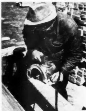
**CUTTING WITH HAND POWER SAW.** A portable electric generator supplies current for locations away from power lines
