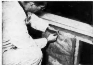
**BATTS OR BLANKETS** should always be worked carefully around pipes and conduits. Water pipes should be protected from freezing with insulation on the cold side but the vapor barrier retained on the warm side.
