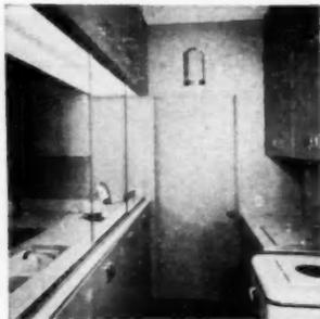
**HEAVY PLATE GLASS** is used for effective sliding panel treatment between kitchen and laundry
