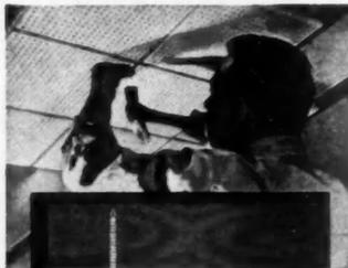
When installing acoustical tile choose a job-designed nail that combines ease of application with these special features: a head end which allows the nail to be driven home without damaging the tiles . . . a collar which holds the tiles firmly in place . . . annular threading which gives superior holding power. The nails are furnished with a plated finish to prevent rust streaks where moisture is present. Send for free samples and descriptive literature.
