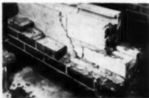
**PARGING** between brick and backing offers high resistance to water penetration
