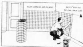
**FIG. 2**—Spread linoleum adhesive on wall area to be covered so that no plaster shows through. Keep below chalk line. Spread just sufficient paste to secure each piece as it is applied. Place first piece of material into position with top edge even with chalk line "A", and butt or fit to door frame or projection. After piece is in place, rub the entire surface thoroughly with a damp cloth to anchor the material into the paste and to remove air blisters.
