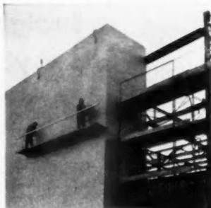
TWO TYPES OF SCAFFOLDING are shown: prefabricated steel units for mason and other construction operations, and hanging scaffold for cleaning and tuck pointing
