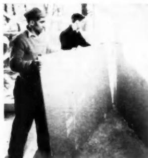
Second stage in double-wall construction with wallboard in horizontal application as finish layer
