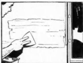
**3** Second coat of cement applied over tape and edges is feathered out evenly
