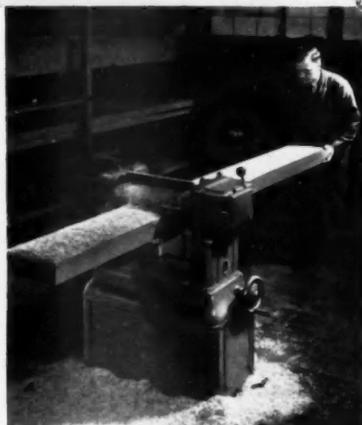
**PLANER** For converting rough lumber at high speed, the Delta 13" x 5" planer is an important money-saver. Rugged, safe, amply powered, it does a precision job on any stack from 13" x 5" boards to 6" pieces unbutted. No kick-back. Also available in 24" x 8" model.
