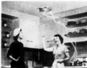
**OVERHEAD FAN** set in ceiling near range removes cooking odors, steam, smoke. Also contains concealed spotlight
