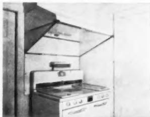
**VENTILATING HOOD OVER RANGE** is a popular feature. Hood is connected to chimney or vent pipe
