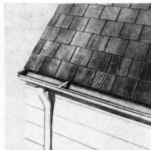
**ROOF GUTTERS** and downspouts are available of galvanized iron, stainless steel, copper and aluminum. Strength, durability, and tightly-sealed joints are important
