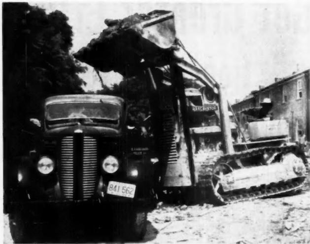
**CORRECTLY SIZED EQUIPMENT** for the job to which it is assigned is always important. It is costly to use a small unit for a heavy job or a heavy unit on a small job
