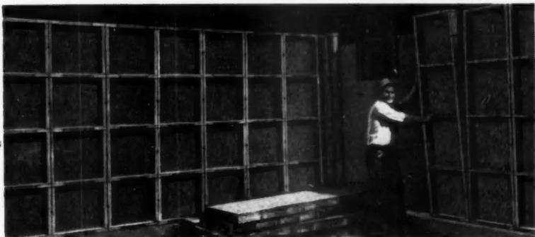
**3** Section showing inside and outside forms ready to pour. **4** To strip wall remove locking wedges and connecting bolts. Pull panels back easily. Break off tie loops with a ½ twist. Wall is smooth, strong and waterproof.
