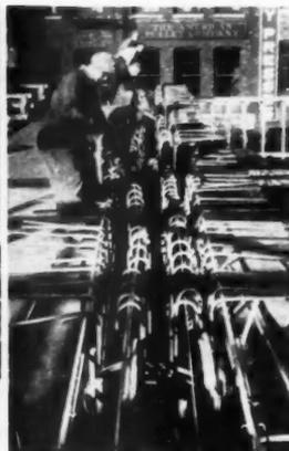
**STEEL RODS and bars used with concrete column and slab floor construction. Two types of bars are shown**
