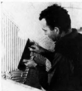
**FIG. 13**—Mastic is applied to the wall first in a vertical and then in diagonal pattern
