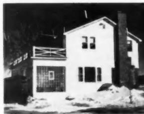
**PANELS OF GLASS BLOCK** used to replace windows on sun porch of a modern farm home. Glass blocks were also used in openings on each side of the chimney
