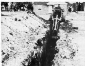
**Digs footings, trenches** with trench-hoe attachment. Cuts narrow, flat-bottom ditch to depth of eight feet. Does precision work on footings, any small excavations.
