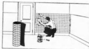
**FIG. 3**—Proceed in the same manner with each succeeding piece. Clean any smudges or excess paste from each piece immediately after it is installed. Wipe with a damp cloth.
