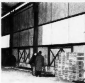
**WHITE CORRUGATED** plastic panels mesh with galvanized iron sheet siding, provide light with privacy
