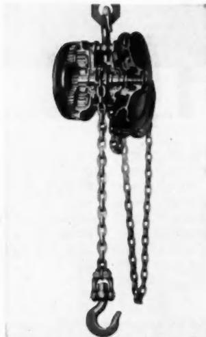
**CHAIN FALLS** makes light work of lifting heavy beams or pipe, provides safety by holding load at any point
