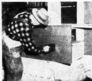
**INSULATING BOARD SHEATHING** is applied by nailing to intermediate studs first with the nails about six inches apart. Nails around the edges are then spaced three inches apart.
