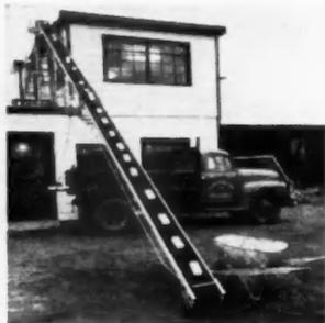
**CONVEYORS** provide an efficient method of lifting brick, tile, roofing materials to second or third-story level. Extensions are available to adjust the height of the conveyor to the level needed
