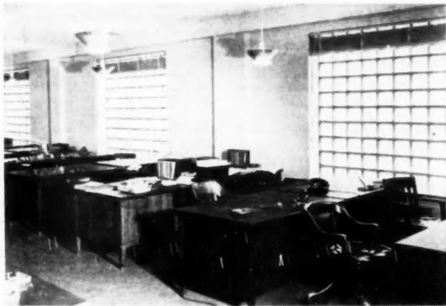
**PANELS OF GLASS BLOCK** admit flood of daylight that is softened and diffused throughout entire office
