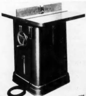
THE SPINDLE SHAPER enables the contractor to save by making his own mouldings and trim. The unit shown above has two speeds, 7000 and 11,000 r.p.m. for different size cutters, and a vertical adjustment range of three inches THIS JOINER is mounted on a stand and powered by electric motor
