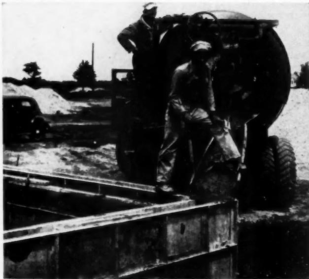
Prefabricated forms save the builder time and money. The units shown above are of rigidly braced metal panels
