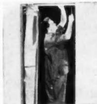
**Step 1.** Slide head track onto trolleys, raise door to standing position, fasten it in place.
