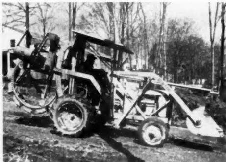
**COMBINATION TRENCHER** and front end loader. This machine is used for digging foundation walls, footings, sewer, water lines
