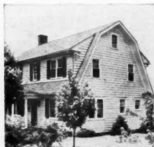
fumes are a problem. Both houses were painted at the same time, No. 1 with a first-quality white lead and oil base paint, No. 2 with a lead-free paint. The houses are shown after 14 months of exposure.
