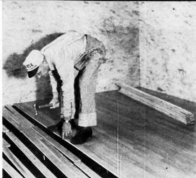
WHEN FINISH FLOORING 1/2 by 2-inch or 1/2 by 1 1/2-inch is used, 6d bright wire casing nails are best—one nail every 10 inches. Flooring 3/4-inch thick takes 4d nails spaced 8 inches apart.
