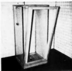
**PREFABRICATED SHOWER STALL** and receptor units may be shipped cheaply in knocked-down form and easily assembled on the job
