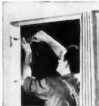
**Step 2.** Attach jamb clips, screws jamb post to them. No planing or fitting necessary.
