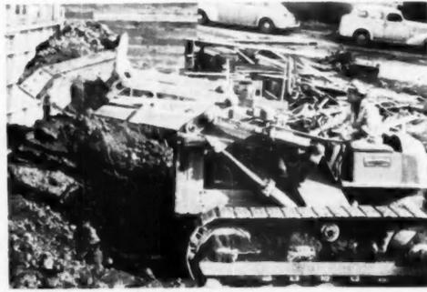
**THE CRAWLER TRACTOR AND FRONT-LOADING ATTACHMENT** are a versatile combination for digging, earth-moving, and many jobs of handling materials on the job
