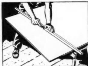
Gypsum board can be cut easily without sawing. Score with sharp knife against
