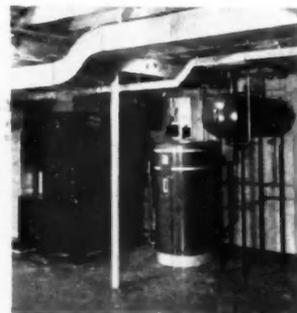
**FLAT**, square, and small-diameter tube shapes are popular for heating ducts in modern installations
