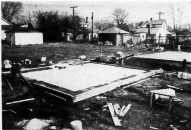
**THE SLAB FLOOR FOUNDATION** is the prevailing type for prefabricated houses in the lower price brackets, but full basements are often used. The builder prepares the foundation in advance of delivery of the packaged house from the factory
