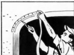
**8** Outside angles of curves are taped with tape cut as shown to allow for bend. Board is scored on back to follow curve
