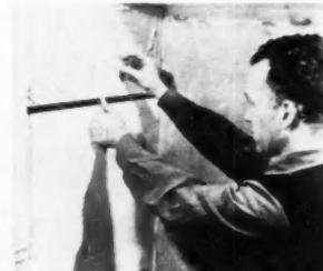
**FIG. 17**—When all of the tile is interlocked in position, feature strip is then applied
