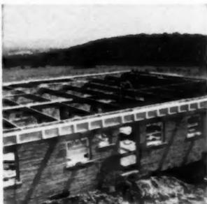
**LIGHTWEIGHT** steel beams form sunshields and porch in this modern design. At right, workman bolts roof purlin to larger structural beam running length of house
