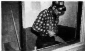
(2) APPLY MORTAR joints 1/4-inch thick
