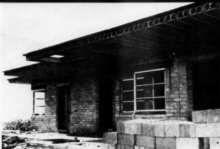
Slabs of prestressed concrete make the 8-foot overhang of the eaves possible here
