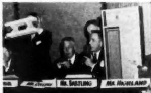
V-SLOT CONCRETE BLOCK offered by Martin J. Bartling Jr., Knoxville, Tenn., who estimates its use can save about 200 linear feet of wire per house. Exterior is designed to look like shingle siding. Next to Bartling (at mike) is scale model of his storage wall closet, built of wood to effect savings on shelving, flooring, hardware and trim
