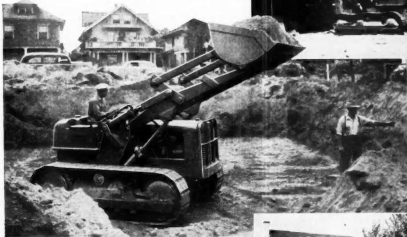
HD-5G Tractor has 40 hp., weighs 16,200 lb. with 1-yd. standard bucket. There are three other models of A-C tractors with 2-, 3-, and 4-yd. standard buckets for doing more work — faster.
