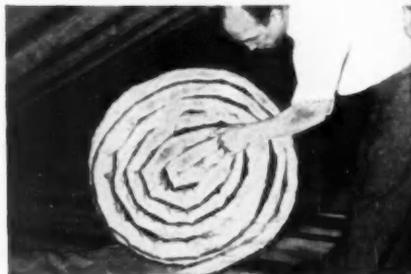
BLANKET INSULATION wrapped in paper with vapor barrier on side
