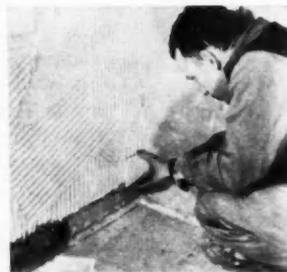
**FIG. 14**—Noting level line, first tile is laid
