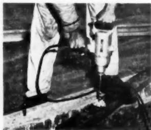
**HAND POWER DRILLS** are versatile tools finding constant use. At left, holes are being bored in mudsills. Right, two models of power drills
