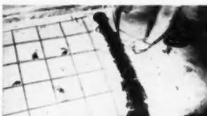
All joints of waterproof membrane should be lapped and sealed with waterproof sealer
