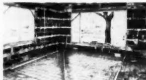
Reinforcing mesh in slab and over ducts adds strength to thin part of slab
