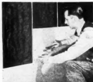
**INSULATING BOARD LATH** is applied with the long edges at right angles to framing or furring. When small areas are to be filled out insulating lath must be used; not wood.
