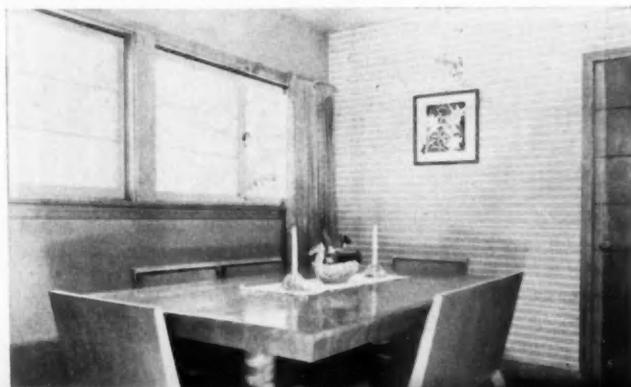
Most awning units, either wood or metal, are delivered to the site as complete packages, ready for installation. Installation is the same in most cases as for other types of window units, the same precaution for metal units being necessary as for metal casement or double-hung types. Weather stripping and interior storm sash and screens make them feasible for use in any climate.
