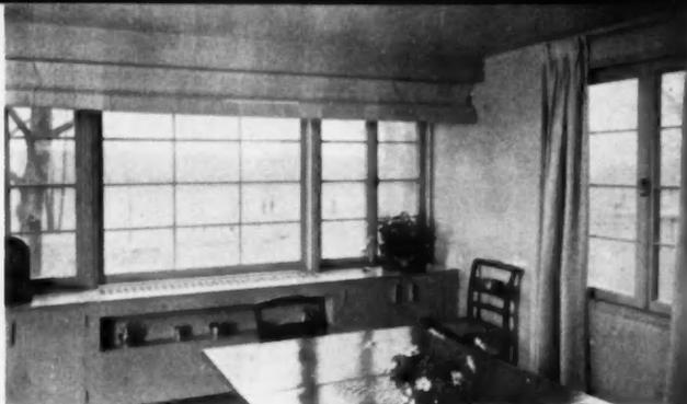
**WOOD CASEMENTS** are easy to install and to make weather-tight. Double-paned glass may be used, and screens and storm sash may be constructed as a part of the sash
