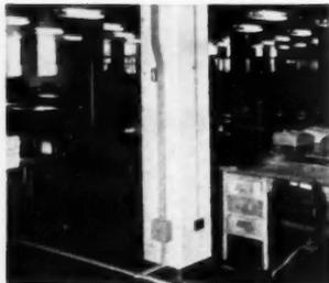
METAL conduit used for surface raceways for telephone lines is easy to install in remodeling operations
