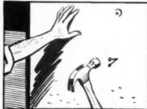
**9** Each board must be tight against furring before concealing nail heads. Care must be taken to avoid breaking surface of board when nailing or dimpling
