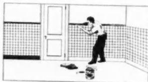
**FIG. 4**—If a cap strip is desired, paste the strip after the lower area of the wall has been finished. Apply to upper wall above finished portion. Baseboard may be applied at the same time.
