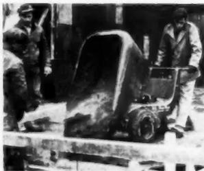
**POWER-OPERATED CONCRETE BUGGY** has large capacity, speeds production, cuts material-handling costs
