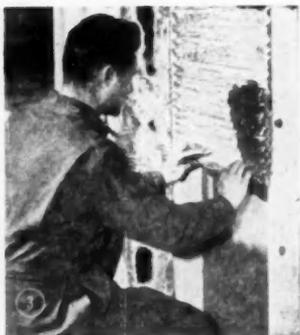
(3) Multiple layers of treated wood fibers attached to heavy creped paper with a reflective aluminum foil cover on one side
