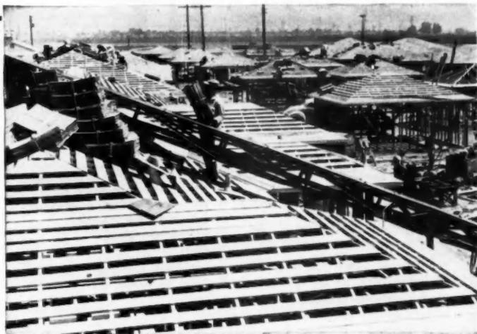
You may be paying more than you think, for "inexpensive" roofing. Don't fail to figure the cost of sheathing when estimating roofing expense. Certi-grade cedar shingles, because of their great strength and rigidity, require only half the sheathing that you must use on ordinary roofing.
