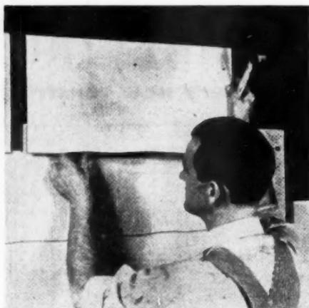
PHOTO ABOVE illustrates the approved method of applying asbestos-cement siding shingles. First, the sheathing or old siding is covered with a felt underlayment. Shingles are then aligned and nailed in position, using non-corrosive nails, with a felt backer strip at each joint. Strips lap lower courses. At least one nail penetrates each strip
