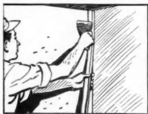
**6** Corner joints are finished similarly to flat-wall joints. Tape is creased down the middle before applying
