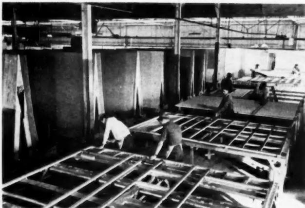
**JIG AND FLOW LINE** for interior wall partitions. "Starting" jig is in foreground, and subsequent stations complete the panel assembly
