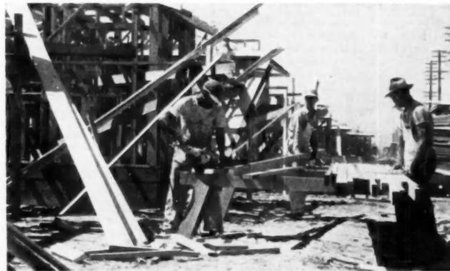
**THE POWER HAND SAW** is one of the most useful tools. Workman is shown making angle cuts on rafters at the job site
