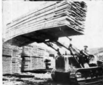
**Handles lumber, pipe, etc.** — lifts, loads, stacks or skids materials with lift fork. Works anywhere, including muddy or rough ground.
