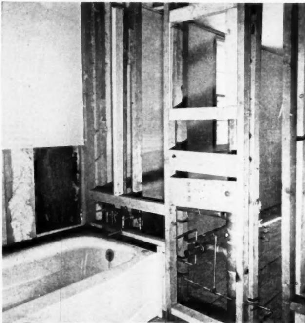
**WATER SUPPLY PIPING** for tub and shower, lavatory, and closet are shown "roughed in" in the partition. Copper tubing is used for water supply, waste and vent lines
