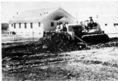
**CRAWLER TRACTOR WITH BULLDOZER BLADE** and cleared treads is efficient for heavy scraping and grading, can also dig shallow excavations
