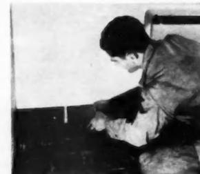
**FIG. 18**—Final step is the applying of Cove base
