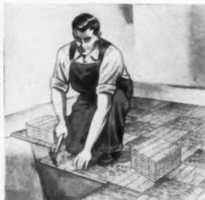
**PARQUET FLOORING** may be nailed to a wood subfloor or an old finish floor in the same manner as strip flooring. Proper construction of the subfloor is essential. Floor joists must be on 16-inch centers and covered solid with 25/32 by 4-inch or 6-inch subflooring thoroughly dried and nailed securely. The surface must be even-bearing.
