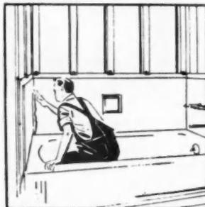
**FIG. 25**—Clean glass and fill joints carefully with compound. This assures a waterproof installation
