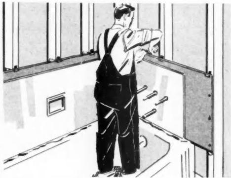
**FOR TUB SURROUNDS.** Prefabricated Carrara units are available for use in bathroom recesses. Panels are shipped to your job ready to install with all cut-outs made and holes drilled to your specifications. No cutting is necessary on the job. You have a variety of colors and a choice of 24- or 28-inch panels.
