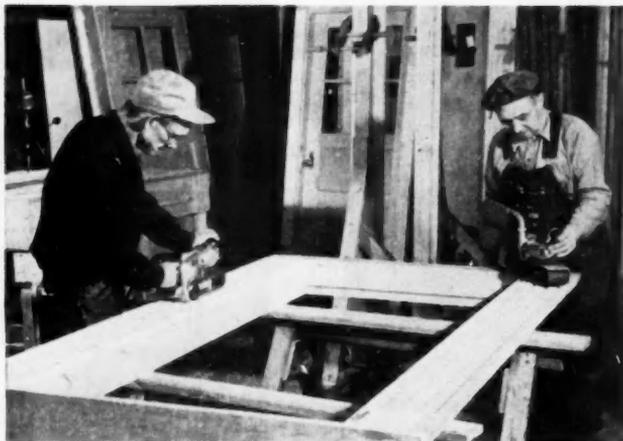
**WORKMEN USING POWER SANDERS** to finish doors. Power drill press with auxiliary oversize table is shown in the background
