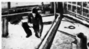
Perimeter system with loop distribution. Feeder duct runs to "T" connection
