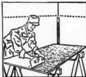
**FIG. 9**—Cover the entire back of the board with cement, spreading it generously with a toothed trowel. Start applying the board in one corner at wainscot level and continue around the room to door opening. Then proceed from the same corner, in opposite direction, to the same door opening. Press the board firmly to the wall, using a few  $\frac{1}{4}$ -inch brads to hold it in place until the cement sets
