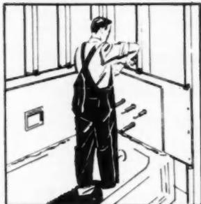
**FIG. 24**—Do the same with the end panels. Let plasterboard extend beyond tub to next stud. If wainscot is 48 inches high, follow the same sequence in setting around second course.
