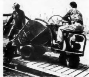
POWEROPERATED BUGGIES speed handling of concrete and other materials. The unit shown above has a capacity of 2000 pounds, and can operate at 16 m.p.h. Low center of gravity and short wheelbase provide excellent maneuverability
