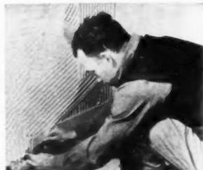
**FIG. 15**—First course sets line for rest of wall
