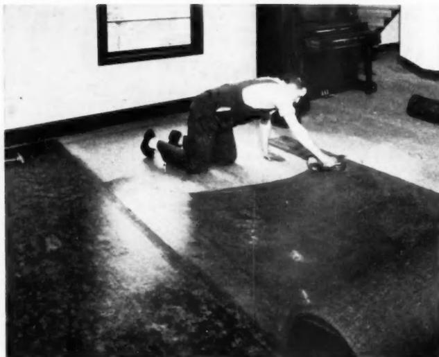
**LAYING LINOLEUM ON A PLYWOOD SUBFLOOR.** The plywood subfloor saves time and labor in this operation, since each panel covers 32 square feet. Large size means minimum linear footage of joints, producing superior base for wood finish flooring as well as for tile or linoleum
