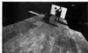
On the basis of recent tests and experience data, Federal Housing Administration now accepts plywood 3/8"-thick as roof decking over rafters spaced 24" on centers, according to a letter from Curt Mack, assistant commissioner of the FHA underwriting office, to Douglas Fir Plywood Association.
