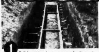
**1** Build cast-in-place concrete footings at least 16" wide and 8" thick. Make sure they are carried to firm soil below the frost line.
