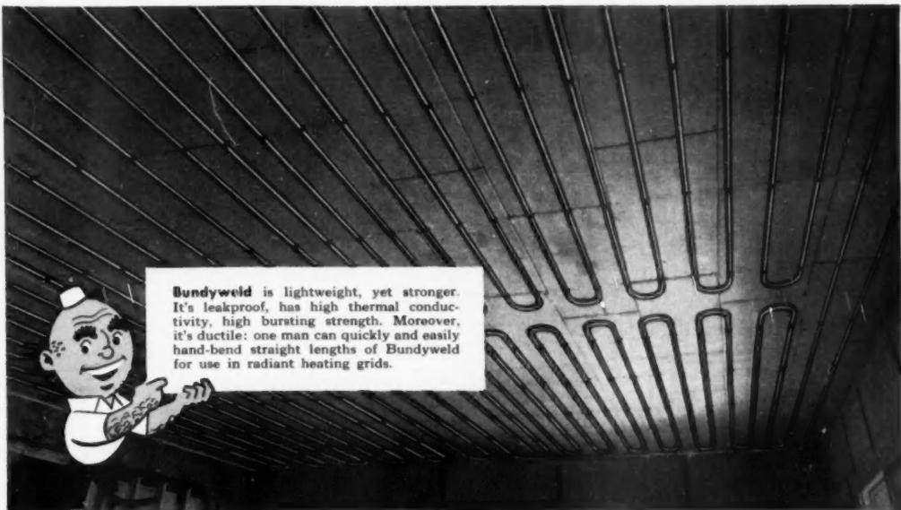
**Bundyweld** is lightweight, yet stronger. It's leakproof, has high thermal conductivity, high bursting strength. Moreover, it's ductile: one man can quickly and easily hand-bend straight lengths of Bundyweld for use in radiant heating grids.
