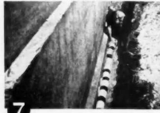
**7** Except in dry climate or well-drained soil lay drain tile around outside of footing and cover with 12" to 18" of coarse gravel.
