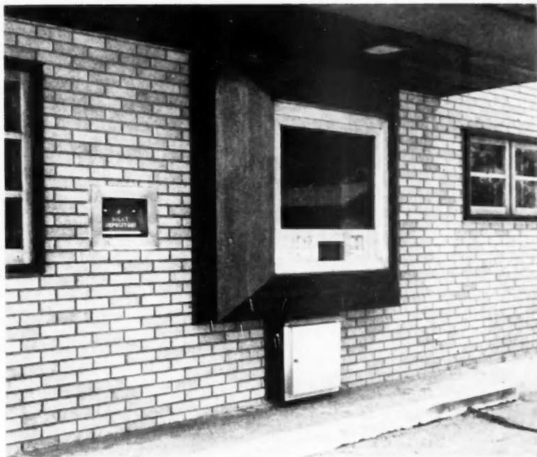
Projecting teller's window for drive-in customers allows banking transactions from cars
