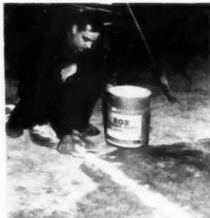
Applying powdered packing compound in widened cracks
