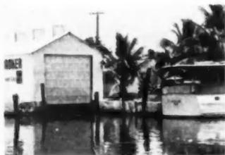
**4** The easy opening mechanism of the upward acting garage door is a safety factor in boat house construction. Large door accommodates cabin cruiser while two section door gives plenty of head-room for runabouts. Mesh below the large door stops wave action
