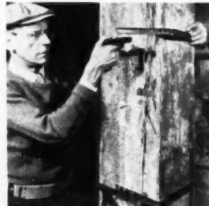
When diamond mesh metal lath is used instead of self-furring lath, column is wrapped at approximately 2-foot intervals with 3/4-inch cold-rolled channels, furring lath a distance of 7/16-inch
