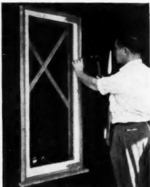
**2 ATTACH OUTSIDE FINS** — Next, attach metal fins at jambs. The grooved edge of the fin fits over the edge of the steel frame. The flat surface of the fin is nailed to the sheathing. Exterior trim can now be applied.
