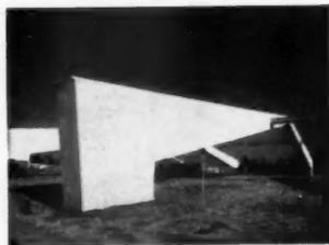
Plywood-formed concrete frames were used to replace conventional posts and roof trusses to achieve an unusual degree of interior flexibility in the Fred Meyers Burlingame Shopping Center Building, Portland, Oregon. Photo shows frames viewed from roof; vertical haunches project down through the roof to ground. Trussed wood joists are suspended from tie-beams secured to the frames. Because the frames are a definite architectural feature, concrete had to be smooth, fin-free. According to Leslie E.
