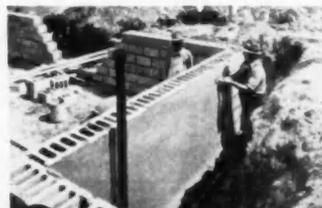
**8** Apply two 1/4" coats of portland cement plaster to earth side of wall from 6" above finished ground line down to the footing.
