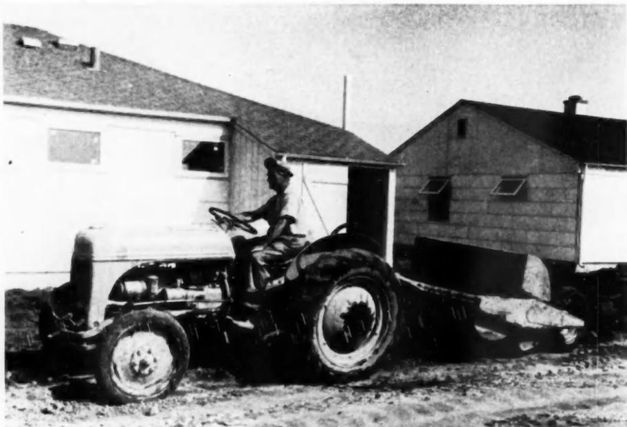
Smaller amounts of top soil are strategically spread with this scraper-loader. All attachments are powered with Ford tractors
