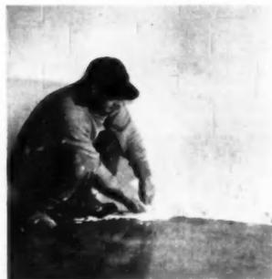
Weep holes are plugged with the powder in dry form
