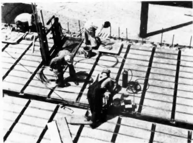
Journeymen laying copper tubing on top of steel box joists (dark lines in photo). 80 per cent of the heat is directed downward from the ceiling, and 20 per cent upward from the floor. Installation is used on the roof, which employs the same general construction
