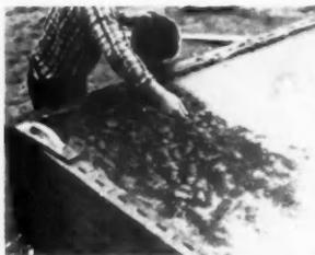
After subfloor has been screeded to proper elevation, colored dust-on mixture can be applied by hand uniformly over floor surface. Proportion should be not less than 125 pounds per 100 square feet
