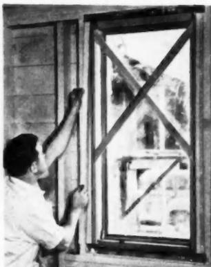
**3 ATTACH INSIDE FINS** — To complete the installation, apply the inside metal fins at head, sill and jambs. Fins fit under the lip of the steel frame and are nailed to the studding. This insures a tight weathertight seal all the way around the window.
