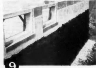
**9** Brush 2 coats of hot bituminous material over plaster. Brace wall with first floor and connect drain tile to outlet before backfilling.
