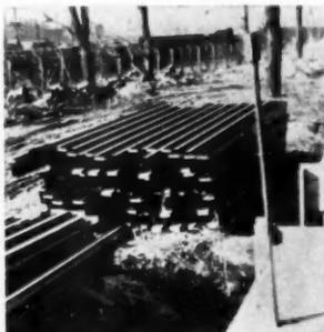
Floor construction starts with steel joint boxes, open at the top, which are set with one end in the rowlock wall and the other on U-shaped steel soffit pan girders
