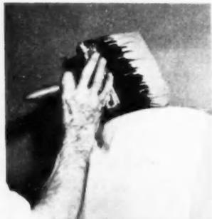
Easy brushing is a characteristic of both the silicon-base stipple texture material and the paint to which the silicon mix has been added. Here a fine sand-textured finish is being applied to a treated wall
