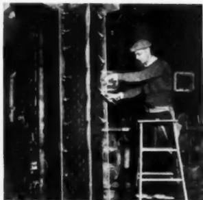
"Tricks of the Trade" are employed by this lather to extend the reach of the corner bead for a four-hour rating. By cutting the flange diagonally and bending it, he forms "ears" which are tied to the metal lath around the column
