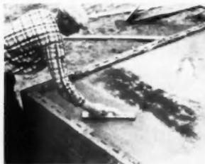
Color mixture is floated and worked into the topping. Discontinue floating as soon as the surface becomes wet
