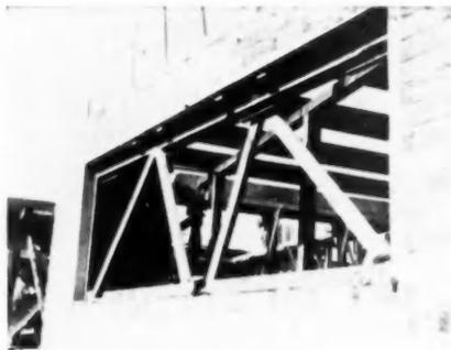
Brick work goes up easily around the precast concrete window trim, held in place by a temporary wood template. Reinforced brickwork over the window does not require lintel steel.
