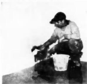
Where masonry was disintegrating, the paint, mixed with two parts silica sand, is trowel-applied
