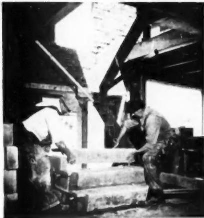
Placing precast concrete stair tread and risers. At one end, support is provided by a steel plate stringer; at the other end by the masonry wall of the stairwell.
