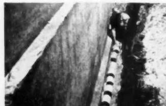
**7** Except in dry climate or well-drained soil lay drain tile around outside of footing and cover with 12" to 18" of coarse gravel.
