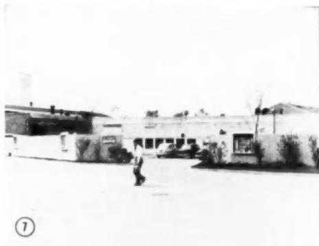
Receiving compounds are big enough to accommodate trailer trucks. They are screened by corrugated Transite board. Shadow boxes, mounted on these walls, give eye-appeal with displays of merchants' notices
