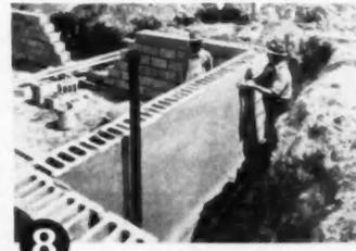
**8** Apply two 1/4" coats of portland cement plaster to earth side of wall from 6" above finished ground line down to the footing.
