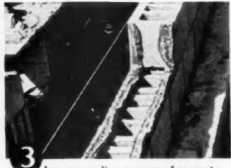
**3** Lay succeeding courses of concrete block plumb and level, using horizontal and vertical face shell bedding as pictured above.
