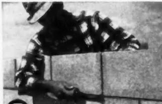
**5** Since the wall is only as strong and as watertight as the mortar joints be sure to compact all mortar joints with a jointing tool.
