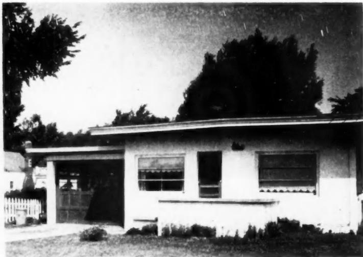
**3** Carport was transformed into a garage by the addition of two garage doors. Owner placed storm sash above the stucco wainscoting of the carport. Doors at both ends make a large open passageway so owner can drive through to the front of his narrow lot
