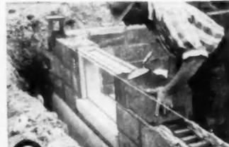
**6** Use a solid top concrete block or fill the cores with concrete in the last course in the wall that will support the floor slab or joists.
