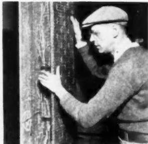
First step in new method of column fireproofing is bending the sheet of self-furring metal lath. Lath is placed so "dimples" are against column flange, furring out about 3/4-inch to provide space for plaster to key
