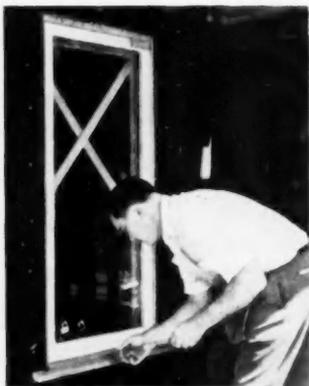
**1 ANCHOR WINDOW** — Pella Windows are completely assembled when they arrive. Just set the unit in the opening and anchor it firmly at the head and sill. Flange screws are furnished for this purpose.
