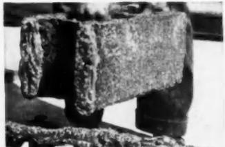
**4** Apply mortar to vertical face shells of one end of next block to be laid in the wall and then press the block firmly into position.
