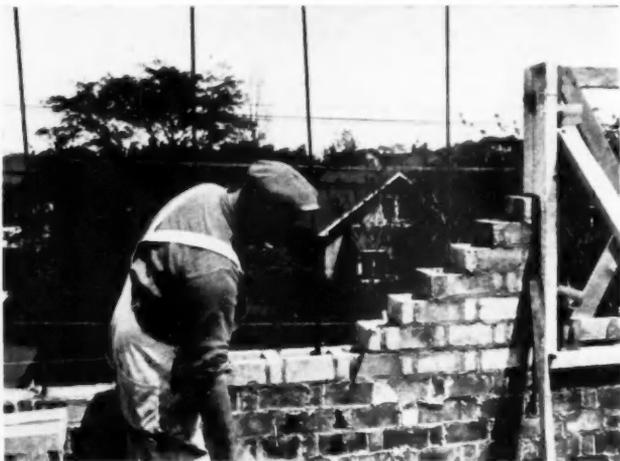
Rowlock reinforced brickwork forms a 3 1/2-inch cavity into which vertical steel rods are placed and concrete poured for reinforcement. Grout is poured every three rows as the brickwork goes up. Horizontal reinforcement is provided by 3/8-inch rods every third course
