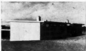
"We've been using plywood for four years," says James Hopkins, assistant superintendent of schools in charge of construction. The portable schoolrooms are fully as well built as the average house and we expect them to be good for 50 years. Plywood construction is lighter and gives maximum bracing strength—a must in movable buildings."
