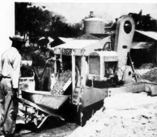
**Pug-mill mix your plaster or mortar with a multi-blade Jaeger Power Hoe**
