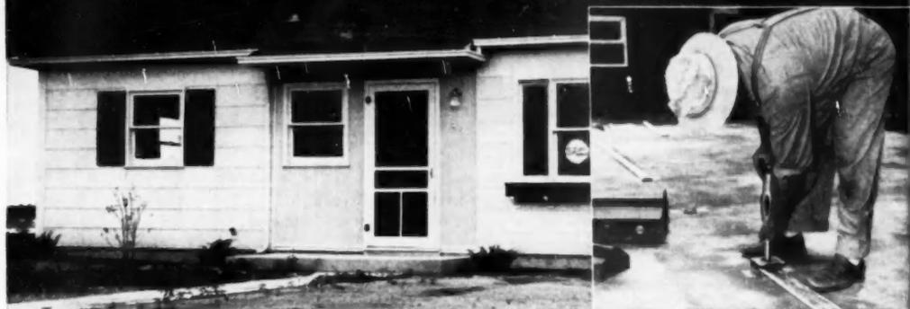
Home builders have taken a cue from heavy construction using Drive-It powder power fastening tools. They find Drive-It is money, time and effort saving when fastening to concrete or steel. Sleepers are anchored by driving hardened steel pins into the concrete slab. This is only one of the many fastening jobs Drive-It does efficiently and economically.
