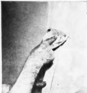
After joints are filled with the new silicon filler, joint tape is immediately worked into the filler and smoothed with a broad knife. When first application is dry, a top coat of filler is applied and feathered out to insure a uniformly flat surface.
