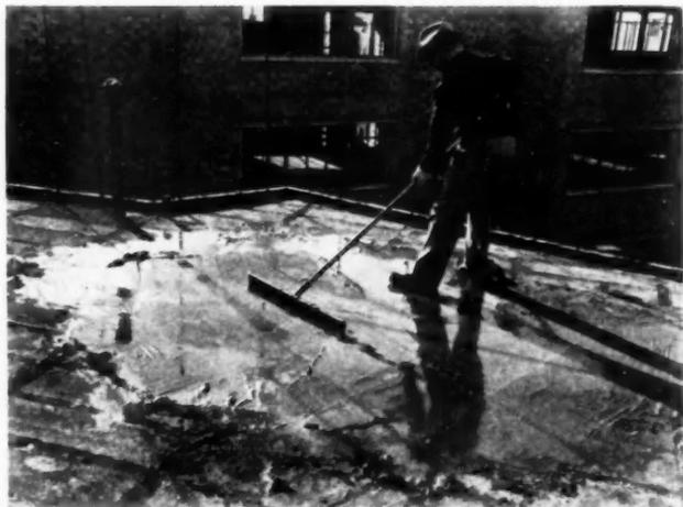
After the copper tubing is in place, structural concrete is poured over the entire floor, dropping down into the hollow girders, joint boxes and V-joints between the slabs. The floor is then finished with a thin coat of concrete spread with a squeegee.
