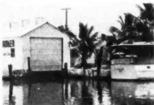
**4** The easy opening mechanism of the upward acting garage door is a safety factor in boat house construction. Large door accommodates cabin cruiser while two section door gives plenty of headroom for runabouts. Mesh below the large door stops wave action
