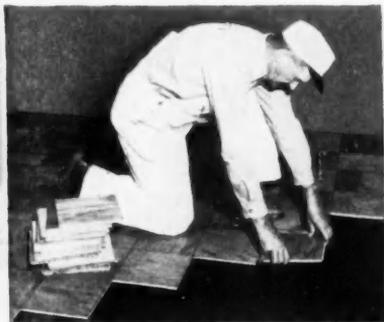
**Looks easy . . . and is easy!** Blocks, with interlocking tongues and grooves, are installed over concrete slab in an adhesive (Everbond Mastic). No membrane-waterproofing required except where hydrostatic pressure may exist. No expansion joints or spaces needed.
