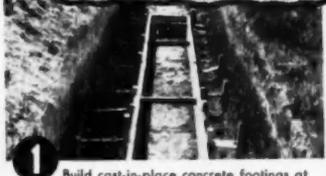
**1** Build cast-in-place concrete footings at least 16" wide and 8" thick. Make sure they are carried to firm soil below the frost line.
