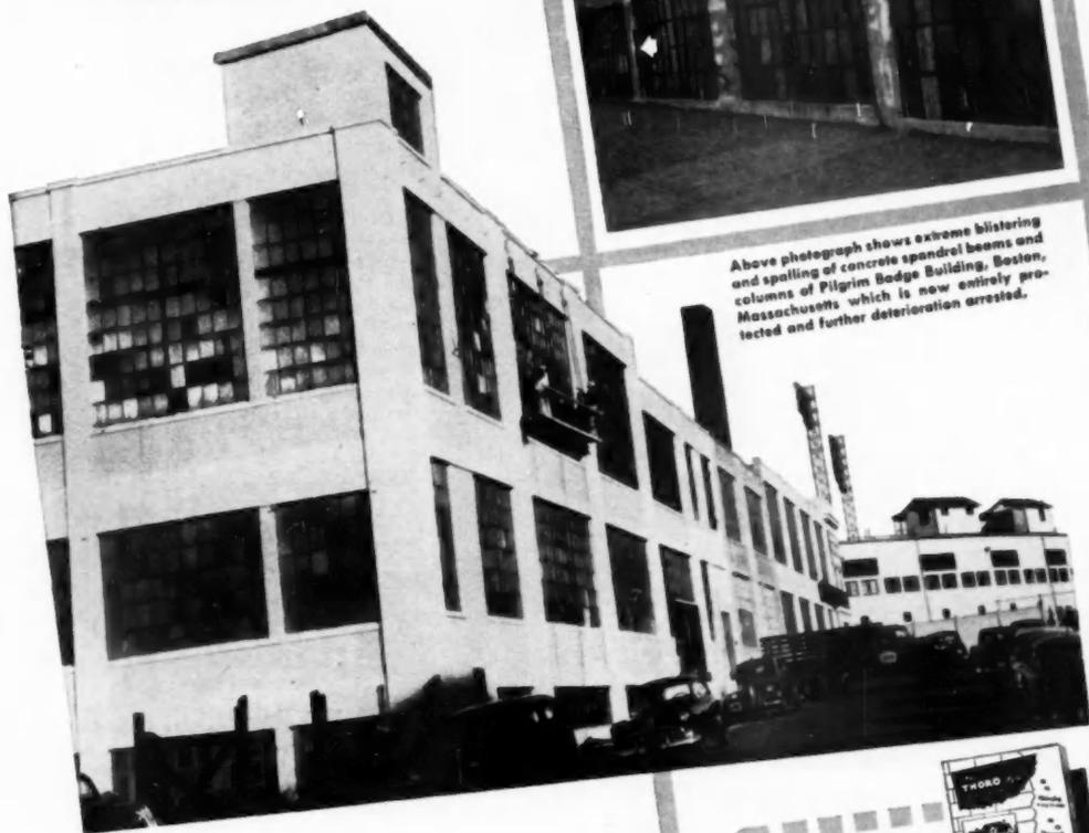
Restoration of concrete spandrel beams and other structural concrete work done by contractor Henry Gironi, Allston, Massachusetts. THORITE Patching Mortar used to seal rods and patch blistered concrete and THOROSEAL to protect surface and patched areas.
