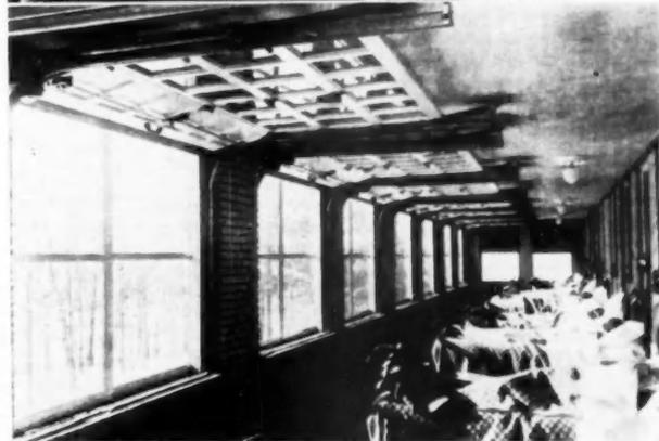
**6** Deluxe breezeway installation has hidden tracks. The glass paneled door slides upward into a false ceiling. Screen cloth has been placed on the exterior for family comfort
