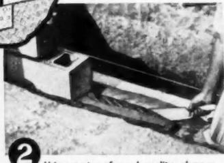
**2** Using mortar of good quality, place a full bed on the center of the footing prior to laying the first course of concrete block.
