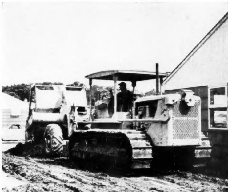
Caterpillar D-7 strips top soil prior to construction and piles it to the rear of lot. Slab and stoops are poured, house is built, and sidewalks and drives are laid. The D-7 returns the top soil to the lot after rough grading
