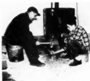
Cracks in the floor were chiseled out so that the cement paint could penetrate to the source of the trouble
