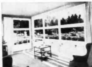
A picture window corner installation. Most of the units have fixed sash. Lower row opens for hopper-type ventilation
