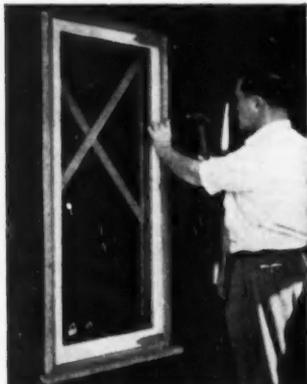
**2 ATTACH OUTSIDE FINIS** — Next, attach metal fins at jambs. The grooved edge of the fin fits over the edge of the steel frame. The flat surface of the fin is nailed to the sheathing. Exterior trim can now be applied.
