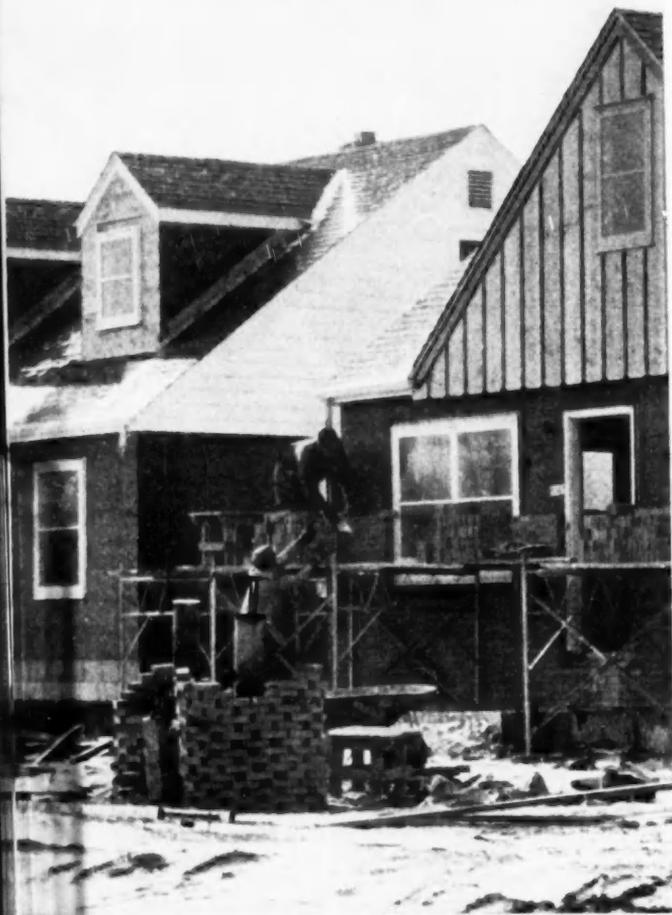
Salamander heats brick that surrounds it. Heated brick is a must when temperature is near zero. Masons in the Milwaukee area are reluctant to start house jobs when the thermometer nears 20 degrees
