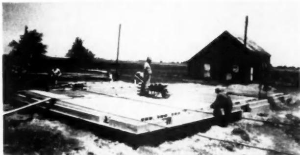
Workmen are setting keyed blocks in place for the first floor deck. Joists rest on foundation wall and eight-inch W. F. beam
