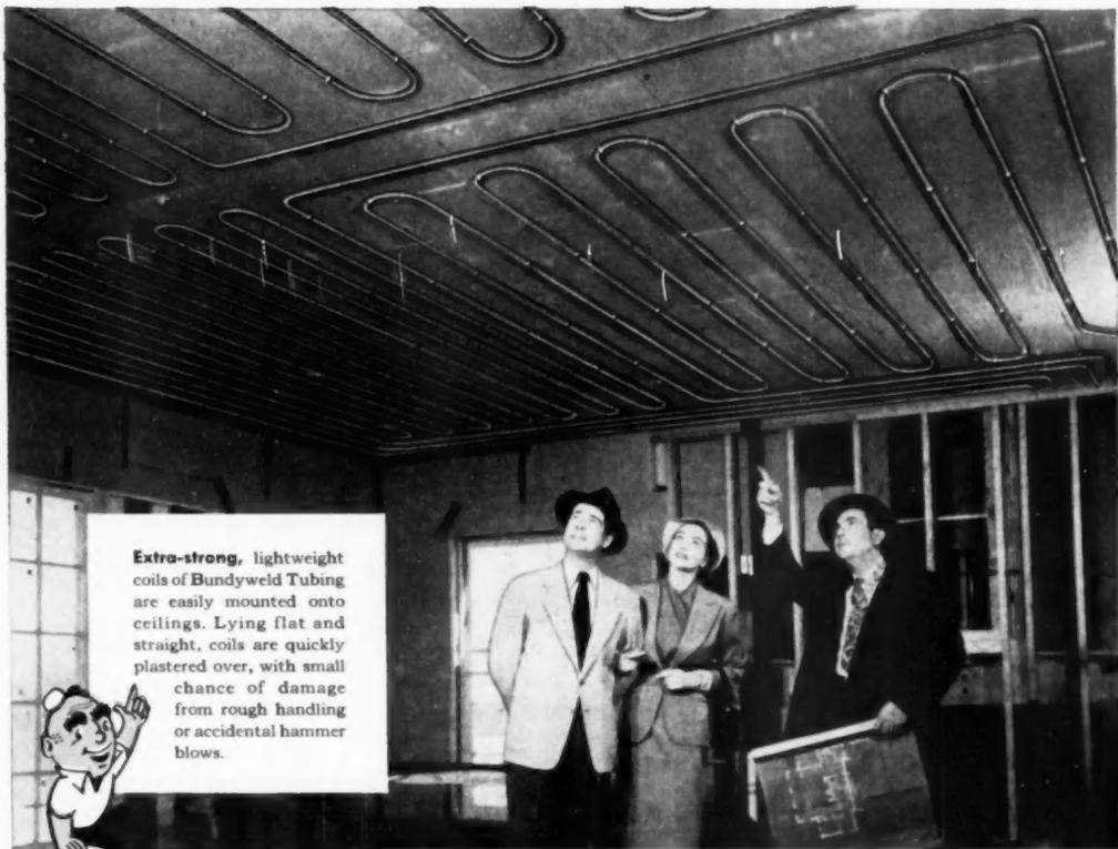
**Extra-strong, lightweight coils of Bundyweld Tubing** are easily mounted onto ceilings. Lying flat and straight, coils are quickly plastered over, with small chance of damage from rough handling or accidental hammer blows.
