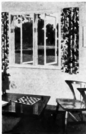
Flexivent units installed on end in casement position. Double glazing panel fits on outside of sash
