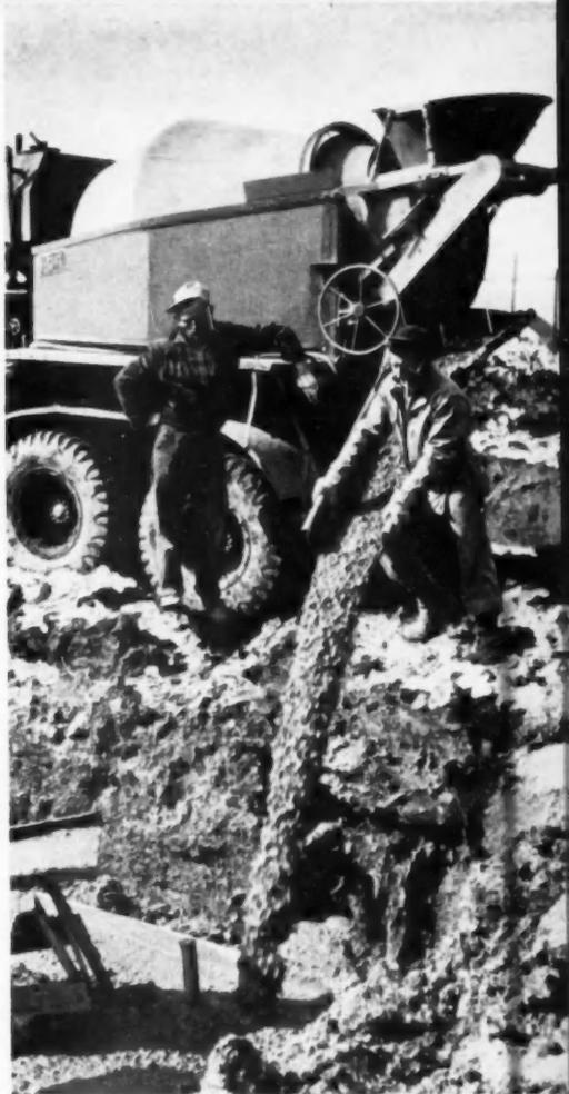
Operators deliver the mix warm and add calcium chloride if the builder requests it. After the footing is poured, straw will be placed over the concrete to protect it from freezing.
