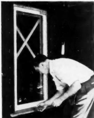
**1 ANCHOR WINDOW** — Pella Windows are completely assembled when they arrive. Just set the unit in the opening and anchor it firmly at the head and sill. Flange screws are furnished for this purpose.
