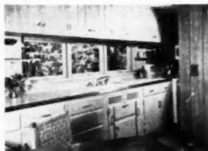
The ribbon arrangement provides excellent light for kitchen counter work space. Sash open outwards, in awning position
