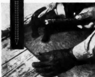
To make your linoleum underlays hold tightly and lie flat permanently, secure them with Hassall annular-threaded linoleum underlay drive screws. They are cement-coated for maximum gripping power. Heads are flat countersunk type. Size: 1 1/4" x #3 gauge. State quantity when writing for prices to:
