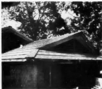
**Hot air is exhausted** through these louvers. Cool fresh outside air is pulled in through open windows. Result: temperature in house drops 10 to 20°.
