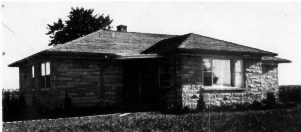
Bedford stone veneer and asbestos roofing are combined. Sunlight enters the projected living room through the east and west windows. The kitchen at the rear right of the house overlooks the driveway and other farm buildings
