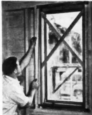
**3 ATTACH INSIDE FINIS** — To complete the installation, apply the inside metal fins at head, sill and jambs. Fins fit under the lip of the steel frame and are nailed to the studding. This insures a tight weathereal all the way around the window.
