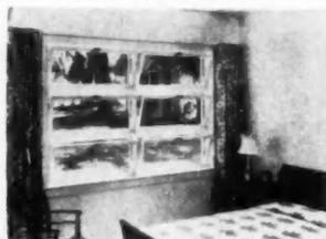
These units are installed well out in the wall, permitting bedroom ventilation without opening sash past the drapery line. They occupy the space of two double-hung windows.
