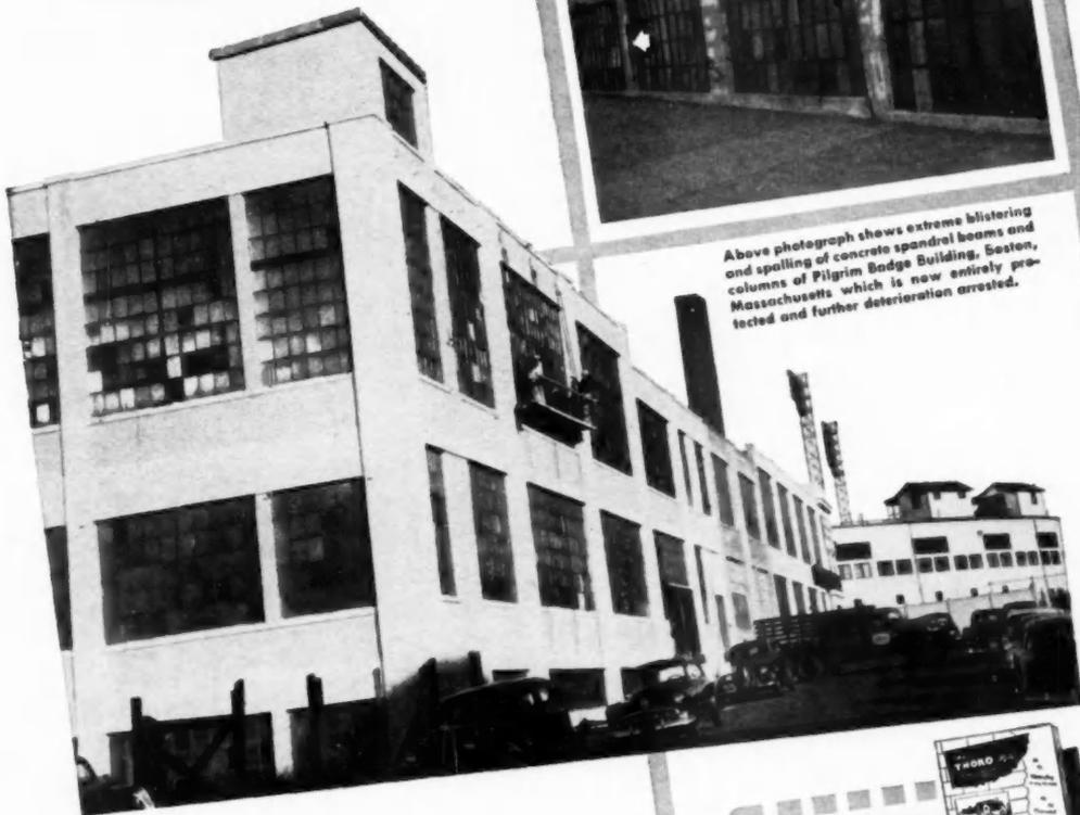
Restoration of concrete spandrel beams and other structural concrete work done by contractor Henry Gironi, Allston, Massachusetts. THORITE Patching Mortar used to seal rods and patch blistered concrete and THOROSEAL to protect surface and patched areas.
