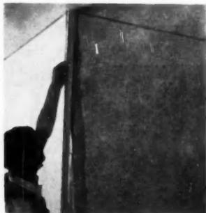
Cement is spread on each side of the corner and Perf-A-Bead is placed in position by holding one end near the top of the corner and pulling the bottom end slightly away from the corner.
