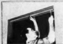
**Step 1.** Cut drilled track to door opening width. Mark and drill holes in header. Average tested time for this operation, four minutes.
