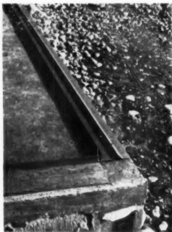
Metal channel, fastened to the foundation, aligns the panels. A similar channel is also at the top of the panels
