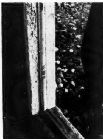
Tubular spline between the panels eliminates shear stresses
