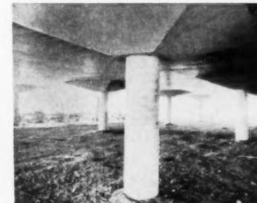
**AB13020—BOOTH NO. 246—FIBRE CONCRETE FORMS**—Sonoco Products Co., Dept. AB, South St., Hartsville, S.C. "Sonotube" concrete forms made of laminated fibre provide a fast, economical method of constructing concrete columns, cylindrical voids. They are furnished in 19 standard inside diameters from 3 to 24 inches. The forms can also be used for upright piping by pouring concrete between two tubes of different diameters. Two coatings are available, for clean finish or form on column.
