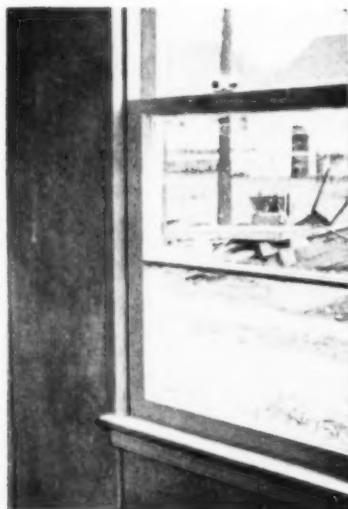
Interior photograph of the window shows that frames are eliminated. Wood sill and window stop are the only trim items. Stop covers pressure type sash balance
