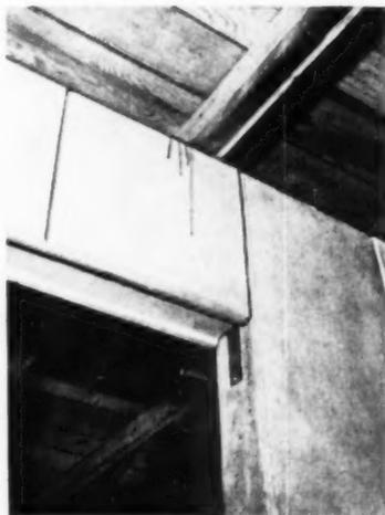
Header is cast with V-joints to match panels. Special hangers are nailed to a full size panel and support the header. The header has the necessary steel reinforcing cast into it
