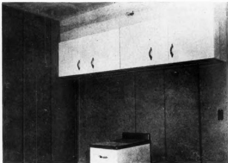
The kitchen soffit has a frame skeleton and is covered with plaster board. The metal cabinets are fastened to the panels as in standard framing
