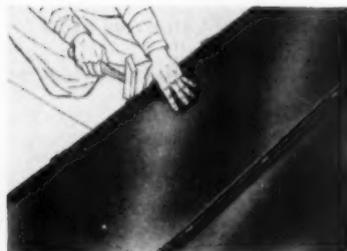
**4.** The second strip is installed with its one inch flange adjacent to the half-inch flange of the initial strip, and cleated down to the roof deck along its half-inch flanged edge
