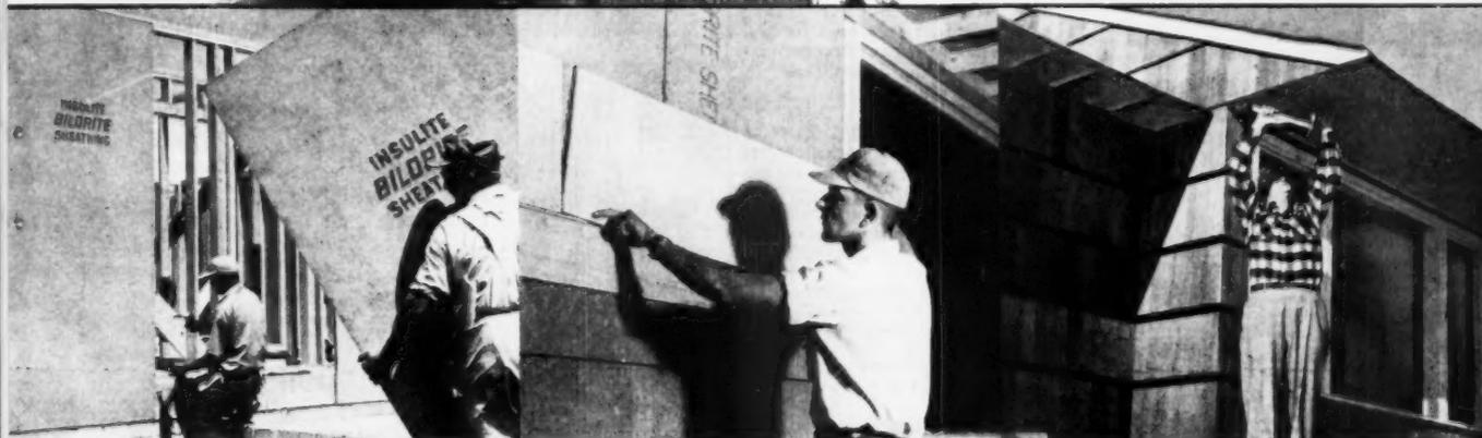
**First, apply Bildrite Sheathing—cut sheathing time as much as 43%.** One carpenter can sheath 1,000 sq. ft. in 8 hours or less. Saves corner-bracing (4-foot Bildrite was the first insulating sheathing to be accepted by F.H.A. for use without corner-bracing). No building paper needed . . . Bildrite is waterproofed throughout. Saves material—no matching loss or waste.
