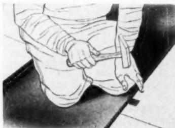
**2.** The initial strip is laid on the roof and attached by cleats hooked on the half-inch flange of the initial strip, each cleat being fastened to the roof deck with two nails side-by-side on the width of each cleat
