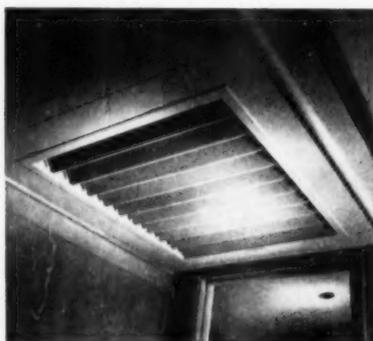
**Automatic Shutter** harmonizes with modern interior of Pace Setter House. Easily installed by screw-fastening metal trim to edges of ceiling opening.
