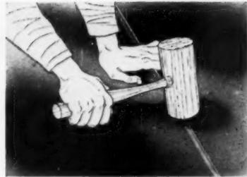
**9.** This type of seam is malleted down flat against the roof, producing a flat locked seam of the same type as shown in the first six steps. The preferred method of seams is to cut the terne into strips as long as can be handled in a brake to make the bends shown in step one
