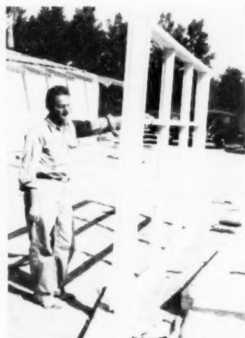
A COMBINATION JAMB, casing and stop unit is milled from one piece of lumber
