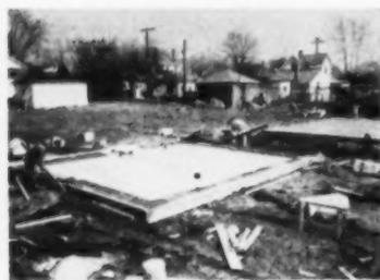
4 Fiberglass insulation is laid around rim. Entire surface is covered with wire mesh, and concrete is poured. Slab is insulated and vapor-sealed
