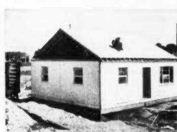
**17** All roof sections are now in position and being nailed down. Pre-assembled gable ends will be moved into position next to complete roof structure
