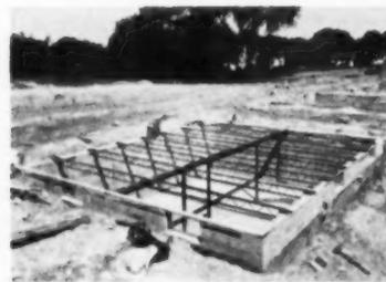
7 Second stage for home with basement is installation of either wood or steel posts, girders, and beams to give firm base for floor and walls
