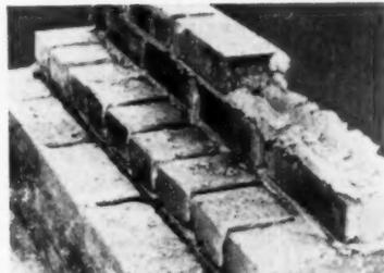
**POOR WORKMANSHIP**—likely to leak. Deeply furrowed bed joints and only partly filled head joints with no mortar in vertical or collar joints allows water to seep in and damage structure
