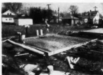
2 Concrete foundation wall must extend below frost line. Depth varies with climate of location. Inside area is filled with 4 inches of pea gravel
