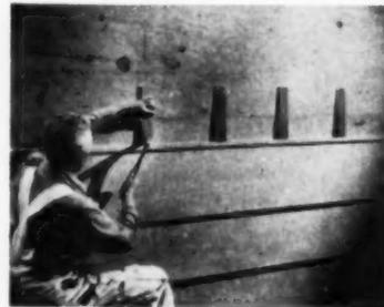
Place shingles over studs where the ends of panels will butt
