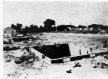
6 First step in erection of home with basement is installation of foundation walls with openings for basement windows in place
