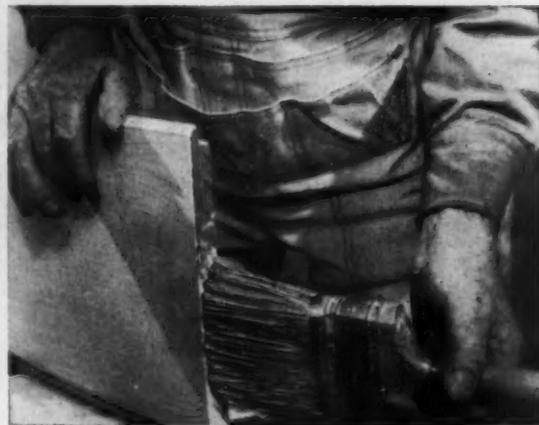
No. 2 is proper sealing of all cut ends with priming material, plus caulking and sealing all joints which might give moisture a foothold
