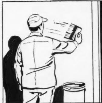
To obtain full, uniform coat, size should be brushed on with semi-circular stroke. Primer and/or sealer give bonding surface for paint
