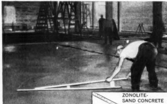
Screeding Zonolite Sand Concrete, grade-level floor. United States Tobacco Co., Chicago, Ill. Ideal concrete for one-pour floors on grade, or for lightweight upper story floors.
