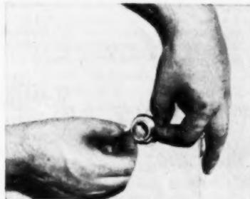
Apply outside knob assembly, tightening up threaded collars with spanner wrench provided. Bedroom and bathroom locks are locked by pressing button on inside knob, unlocked by turning inside knob
