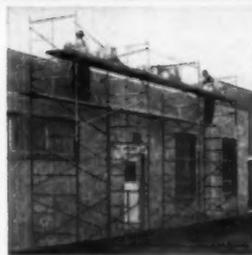
No wonder builders like balanced Safway steel scaffolding! It's engineered for structural stamina. Easy-to-assemble units speed erection of scaffolding and make dismantling simple. Pictured here is the lowest cost steel scaffold on the market for loads up to 50 lb. per sq. ft. with heights up to 40 ft.
