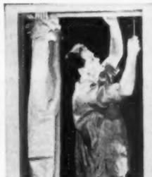
**Step 1.** Slide head track onto trolleys, raise door to standing position, fasten it in place.
