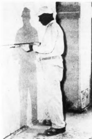
The partition is now ready for plastering. A scratch coat is applied to both sides. After the scratch coat sets, a brown coat is applied to the unbraced side. When the brown coat sets, the temporary channel braces are removed, and a brown coat is applied to the side formerly held by the braces. Wooden runner serves as ground or screed strip for the brown coats. Any standard plaster finish may be used
