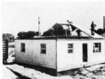
**16** With roof peak formed by two sections, roof moves rapidly towards completion. A total of only 3 or 4 hours puts the house under roof!
