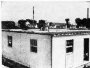
**13** With all walls and ceiling sections in place, work begins on roof. Men are installing ceiling purlins. Note notched rafters at right
