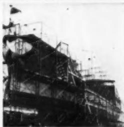
Standard Safway equipment is easily assembled to fit the curved bow and sloping sides of this vessel at the U. S. Navy yards. Only a few basic types of interchangeable members are needed to assemble scaffolds of any required shape and height.
