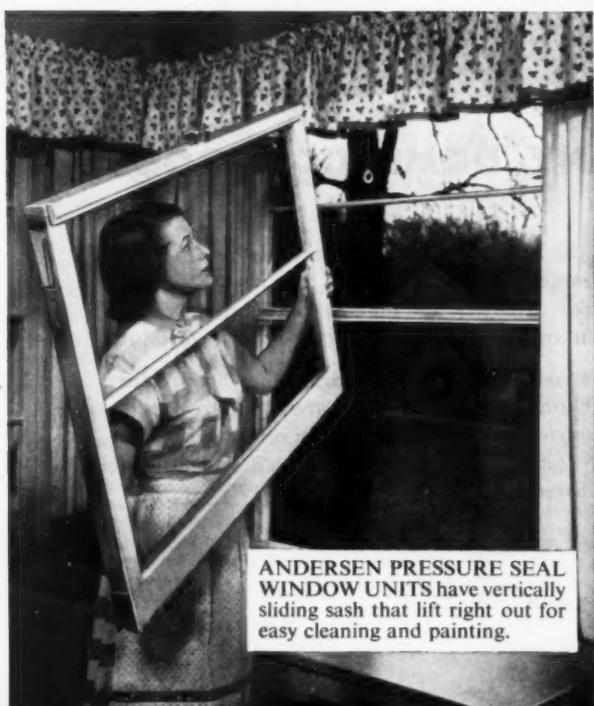
**ANDERSEN PRESSURE SEAL WINDOW UNITS** have vertically sliding sash that lift right out for easy cleaning and painting.
