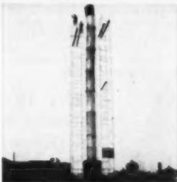
Workmen safely reach into the sky 75 feet high. They're using Safway scaffolding to dismantle a heavy steel stack in Minneapolis. Safway carbon steel frames are solidly joined with wing nuts to tubular steel cross braces for strength. All welds are made by master welders.
