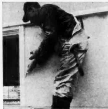
CAULKING COMPOUND being applied around outside of window frame to insure weather-tightness
