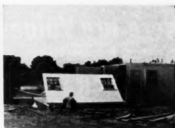
**12** Men here are raising exterior panel that will complete the rear wall of this home with full basement. Quality control in factory insures "fit" on the site
