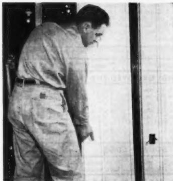
Plank is 16 inches wide to cover one stud space, has t&g joint for concealed fastening. Scoring is to resemble 6 and 10-inch alternating planks. Application here is a basement amusement room.
