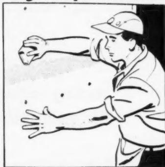
Joints, treated nailhead depressions and other surface irregularities should be lightly sanded to insure smooth receiving wall
