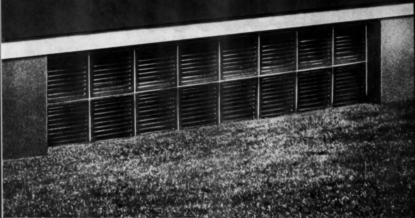
Installed in place of sash, Insulux Glass Block hides outside views and makes a sound, weather-tight, insulating wall.
