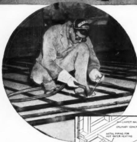
Zonolite Insulating Concrete under radiant heat pipes promotes efficient operation of heating system, better temperature control, saves fuel.
