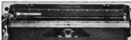
— The Office-riter's 11-inch paper capacity is large enough for all general office typing, and the writing line is the longest of any 11-inch carriage machine now manufactured. The Office-riter easily takes paper, carbon packs or forms up to 11 inches wide.
