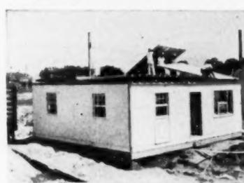
**15** With first roof section in place, second section goes up to meet it. Factory equipment such as large tenon saw makes 23 notches in rafter at one time
