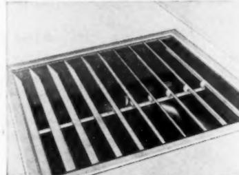
**GRILLE or louvre** for ceiling fan is a typical installation. Similar metal louvres are also popular in doors to control drafts and room ventilation
