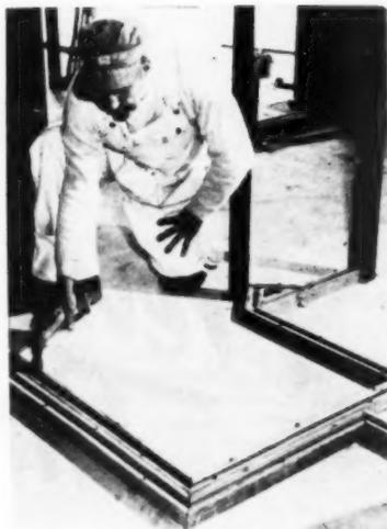
The first step in the installation of a two-inch solid gypsum partition is to secure a grooved wooden runner or 3/4 inch steel channel to the floor according to the partition layout with nails or adhesive
