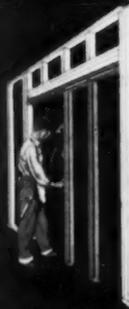
**SERIES 800** Prefabricated warp-proof, all-metal frame for closed pocket installations. Series 400-A track already installed.
