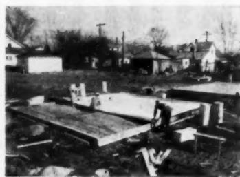
3 Continuous water-repellent blanket of sisalkraft paper is laid over gravel and foundation to give vapor seal, keep cold and damp from slab
