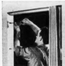
**Step 2.** Screw in jamb clips, attach jamb post to them. No planing or fitting necessary.
