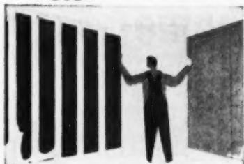
First step: Nailing the 3/8-inch panels to studs and joists
