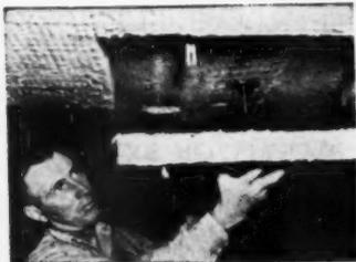
3. FIBERGLAS Insulation Type PF-613, 2" thick — bonded to concrete ceiling using MIRACLE PRONGED ANCHORS at Radio City Studio 6B, New York, N. Y. CONTRACTOR, William J. Scully, Inc., New York, N. Y.
