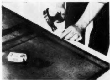
First step in attaching plastic saran screening is to start at top corners to hold material in place. Nail tacks or staples about 1½" apart
