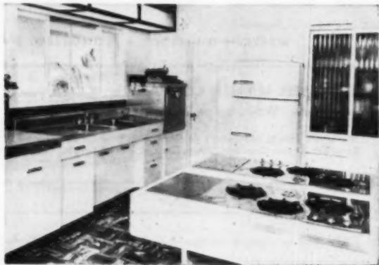
Drop-in cooking top and in-a-wall oven are features of this kitchen plan for No. 2 ranch type home. The convenience of peninsula snack bar to cooking top highlights the flexibility of arrangements possible with these fixtures for decentralized cooking. Heavy insulation built into the oven is the basis of "retained heat" cooking which makes for fuel economy. Drop-in cooking top fits into a waist-high counter top, where wide work surface increases efficiency
