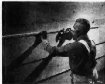
For deep shadow line, nail strip of plywood or 3/8-inch furring strip along top edge of each course and (below):
