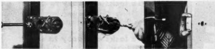
Mark door, set jig and drill two 7/8" holes for latch and spindle
