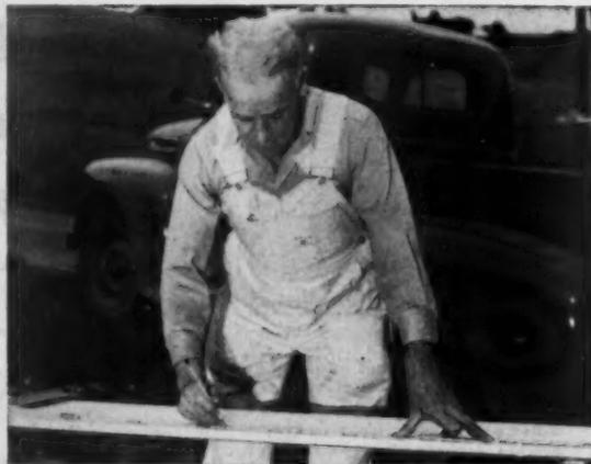
In applying siding and trim two things help keep moisture out. No. 1 is accurate cutting for tight-fitting joints
