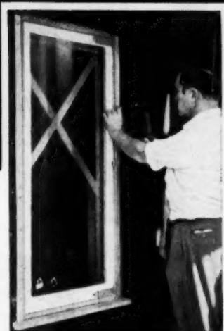
**HERE'S WHY PELLA WOOD CASEMENTS ARE EASY TO INSTALL . . .** When received on the job, they are simply set into rough wall openings, caulked and secured in place by steel interlocking fins. Pella Wood Casements are completely assembled and prefitted at the factory—cut installation costs to a minimum. Stock-size units can be combined into hundreds of custom-like effects.
