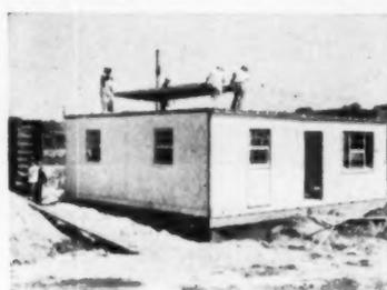
**14** Carrying first roof section to its position. Notched rafters have been prepared to receive roof sections and speed erection
