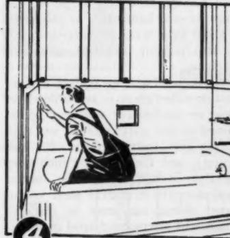
**4** Clean glass and fill joints carefully with the pointing compound supplied. This assures a thorough waterproofing installation.
