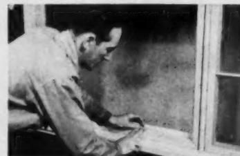
Third, place wood setting blocks  $\frac{1}{4}$ " thick, 1" wide and 3" long in position shown. For 36" sash, setting blocks are in 9" from each end.
