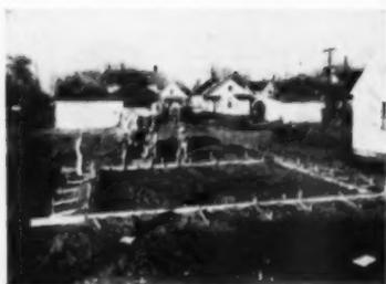
1 First step in erection of prefabricated basementless home. Crew stakes out ground area for slab. Pipes and conduits are put into position
