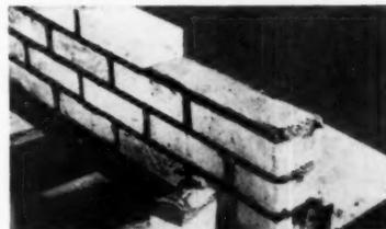
**HERE** is good workmanship. Bed joint is spread to uniform thickness. Mortar is only slightly furrowed. Head joints are completely filled by buttering end of brick before shoving into place. Slushing partly filled head joints does not do the job!
