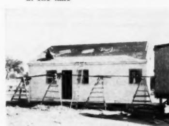
**18** Shingling starts 3 to 4 hours after first panel is unloaded. Interior finishing, wiring, plumbing, landscaping, will require 10 days to two weeks
