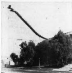
Weather and corrosion won't hurt the Safway scaffolding used in this 185 foot ski slide in Los Angeles. It's corrosion and rust resistant. Special phosphate bath converts surface of Safway steel scaffolding to non-metallic oxide. Baked-on weather resistant paint gives extra protection.
