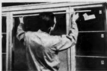
First step is to check window against size of window opening. Opening should be  $\frac{1}{4}$ " larger on all sides than the double glazed unit
