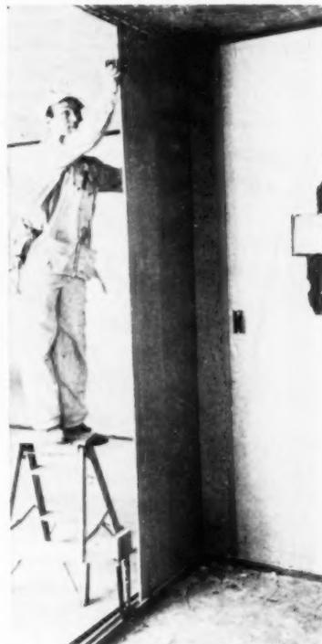
One-half inch, long length gypsum lath with grooved or square edges is set into the floor runner, and tie-wired or clipped to the ceiling runner. Adjacent laths must be butted tightly
