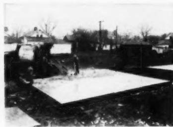
5 Finish coat of concrete is applied to entire area of floor slab. A smooth surface is provided to insure smooth floor when laid on slab
