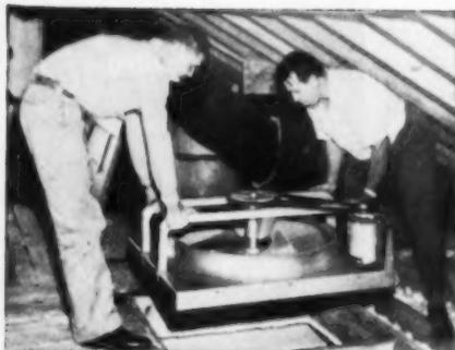
*Installation is easy and inexpensive. Fan rests on attic floor—no suction box or other extras. Automatic ceiling shutter screw-fastens over ceiling opening—no replastering or repainting.*
