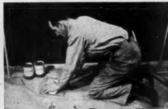
Next, use a good glazing compound, adequately worked. Never use putty, as it hardens, and unit no longer "floats" in the opening. Use elastic glazing compound.
