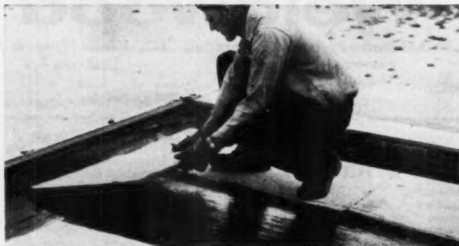
After flashing, the felt is mopped in place. Hot roofing asphalt is applied to the roof deck upon which the insulation board is set. This asphalt coating acts as a vapor barrier. Under conditions of excessive humidity within the building, the Insulation Board Institute recommends the addition of two plies of 15-pound felt mopped together with asphalt coatings. Insulation consists of panels of one-inch rigid insulation board abutting each other and against the edge of cant strip.
