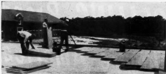
Closeup view of installation shows the ease of handling the insulation board panels. After panels are secured to deck with hot asphalt, they are sufficiently strong to support the weight of mechanics and equipment
