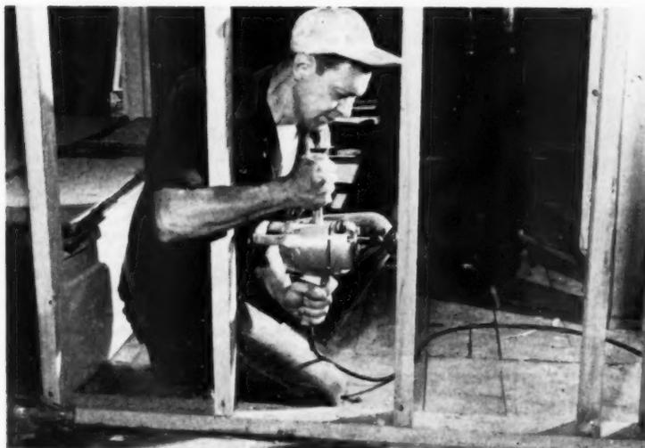
This short, "stubby" drill will allow work in restricted areas, such as between studs. With a  $\frac{1}{2}$ -inch (steel) capacity, this close-coupled tool permits the attachment of 2-inch special auger to spindle after chuck is removed. Drill pictured is only 11 $\frac{1}{2}$  inches in over-all length and is only 3 $\frac{1}{2}$  inches wide
