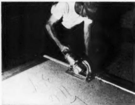
Precutting interior and exterior drywall on modular cutting table. Quick setting gives exact dimension, taking into account the offset of the saw, thus, one worker does this usual two-man job
