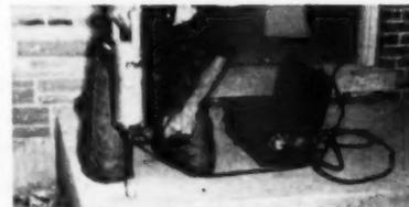
Portable electric hammer speeds boring of holes in concrete porch for installation of ornamental railing. Equipped with turning wrench and handling drills from 1/4 inch to 1 1/2 inch, tool is plugged into rectifier box which changes AC current to DC for magnetic-type hammer. It strikes 3,600 blows a minute
