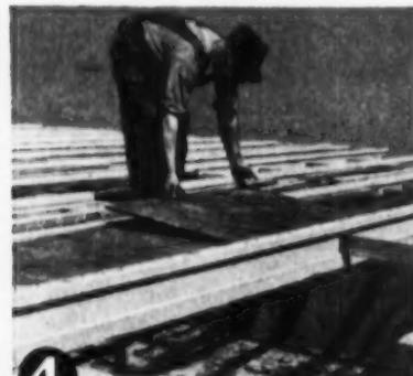
**4** Lay sheathing or plywood forms over spreaders. Allow for expansion if the wood is dry. Place conduits for plumbing, heating and wiring and then thoroughly oil the forms.
