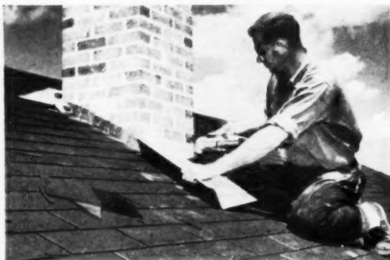
Portable electric shear speeds up work on metal chimney flashing. Shear is used for straight and contour cutting, and cuts on radius as small as one inch. It cuts metals up to 16-gauge
