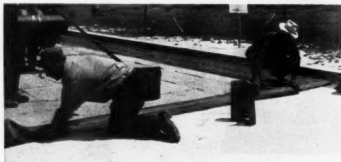
When the felt-strip water-stop has been applied at the end of first section of insulation board application, roofers then cover this area with hot asphalt and roofing felt. A good deal of care is used to have felt adhere snugly to roof at seams. Creasing or buckling invites air pockets which destroy the efficient performance of the roof
