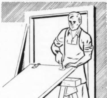
**2** Use template to position carriers, attach with single screw. Mount guide-strip on bottom rear. (2 minutes)
