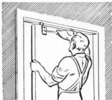
**4** Bottom clearance should be  $\frac{1}{8}$ ". Loosen screw, raise or lower door, tighten. Insert other screw. (100 secs)
