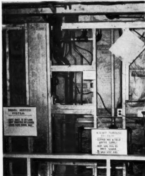
The kitchen wall with the entire plumbing, wiring, heating and insulation visible
