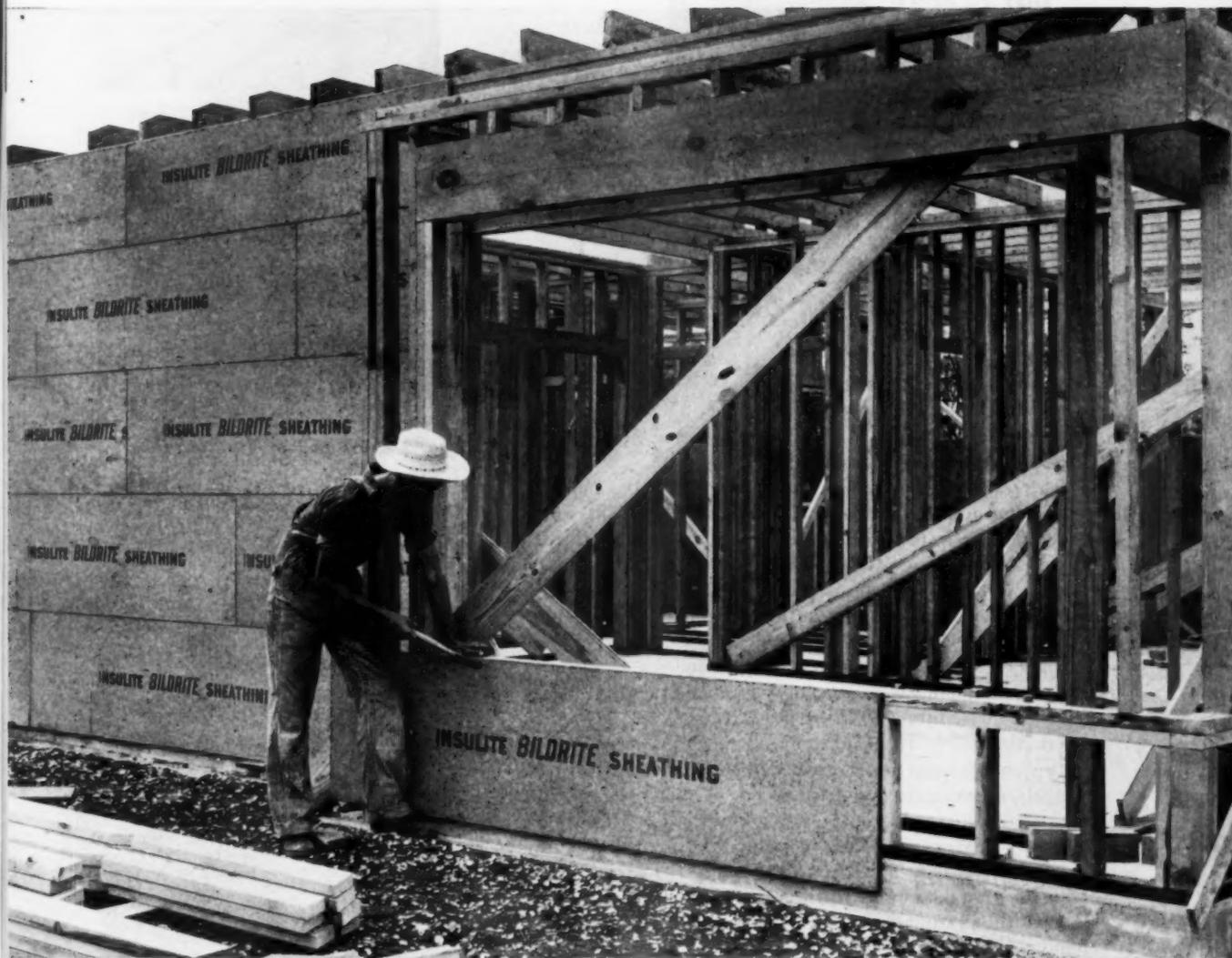
**4. Bildrite goes up faster, easier.** One carpenter can sheath 1,000 sq. ft. in 8 hours or less with Bildrite. Cuts application time as much as 43% compared with wood. Has tremendous bracing strength. 4' Bildrite eliminates need for corner-bracing (F.H.A. accepted)!
