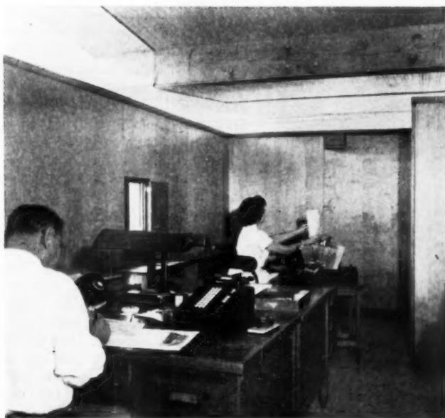
Fitch-plate beam and steel support can be seen in the payroll-bookkeeping department. Note how roof at beam does not bear on the side wall. Outside window facilitates paying employees
