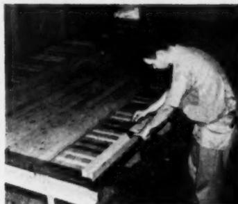
**Marking the plate on the universal jig table with the aid of a four-inch hard-board marker** (see chapter 9, Sept., 1952)
