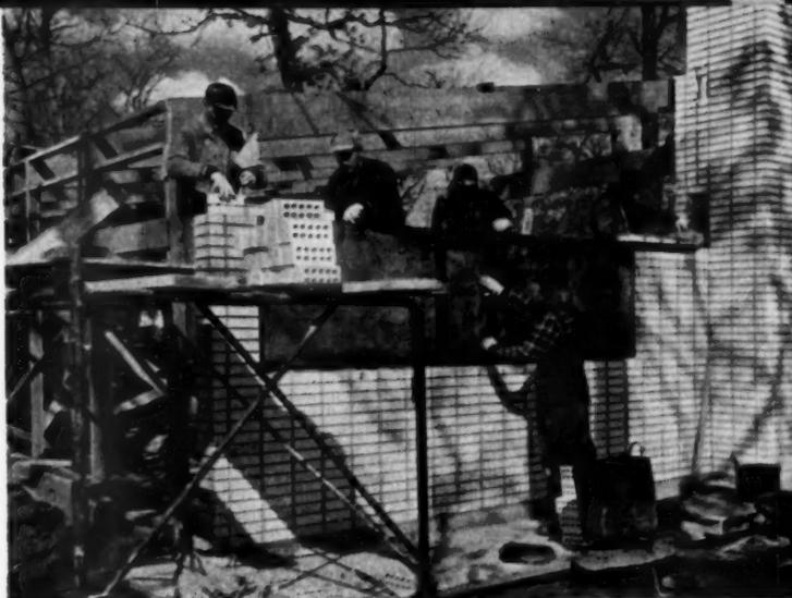
Laying up cavity wall with face brick, both sides. One-inch rigid insulation fills the void between the two wythes
