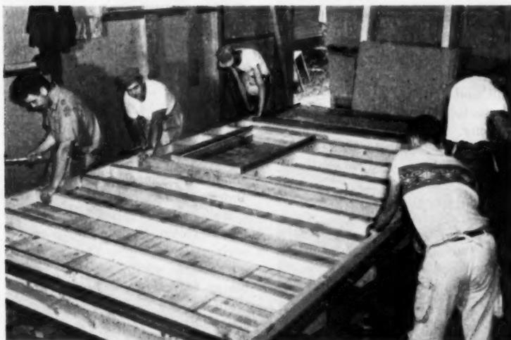
**Framing assembly of wall sections on the modular jig**
