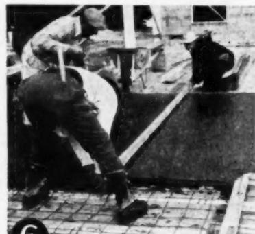
**6** Place properly proportioned and mixed concrete. Spade or vibrate the mix, compact it with wood float, finish with steel trowel. Moist-cure thoroughly, then remove forms.
