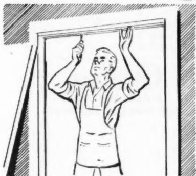
**1** Mount track to header, keeping face of track flush with opening. (35 seconds)
