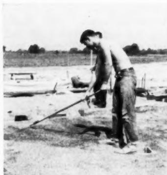
Applying loose fill around the heating ducts and pier forms
