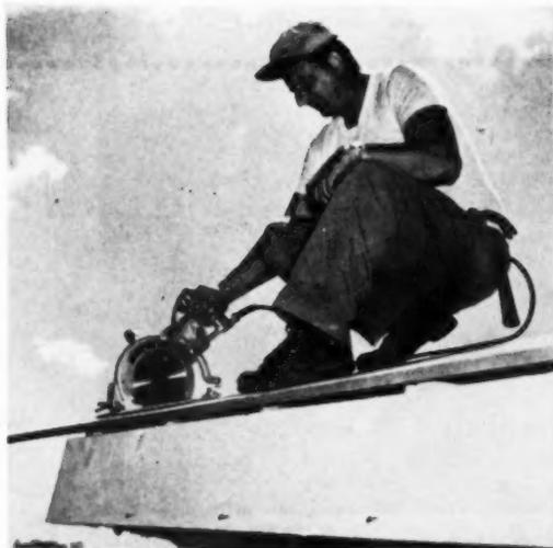
Carpenter is using power saw to trim roof sheathing, reducing operation time from hours to minutes. The same saw, with its straight cut depth of 2 $\frac{3}{8}$  inches and 2 $\frac{1}{2}$ -inch depth cut at 45 degrees, is powered to cut masonry, metal, all types of composition material
