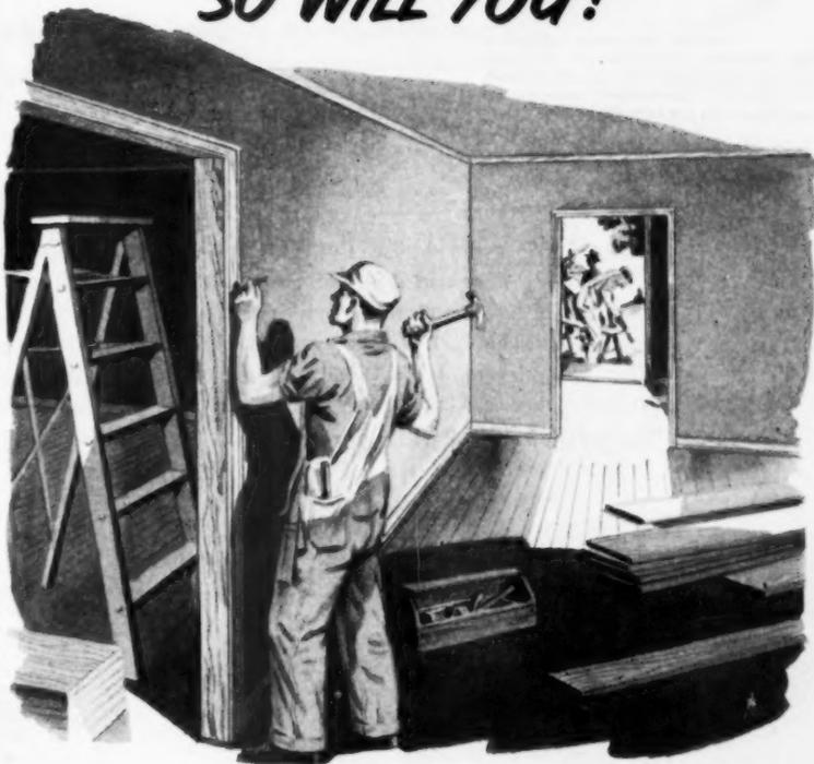
Because its fine grain, soft texture, light weight and freedom from pitch work easily. The wood cuts clean, matches accurately at mitres. Properly dried to specified moisture content, it doesn't shrink, swell or split. It absorbs primers evenly, holds paint, stains or transparent finishes, free from bleeding or raised grain.
