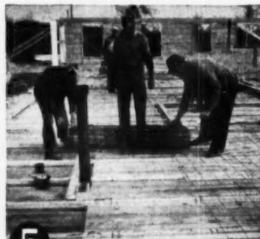
**5** Set insulation around outside edge of floor and then install reinforcement consisting of either (1) wire fabric or (2) steel bars placed at right angles to the precast joists.
