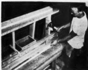
**Making a subassembly.** The subassembly makes it possible to cut all horizontal plates for all wall sections in modular dimensions (see chapter 8, Aug., 1952)
