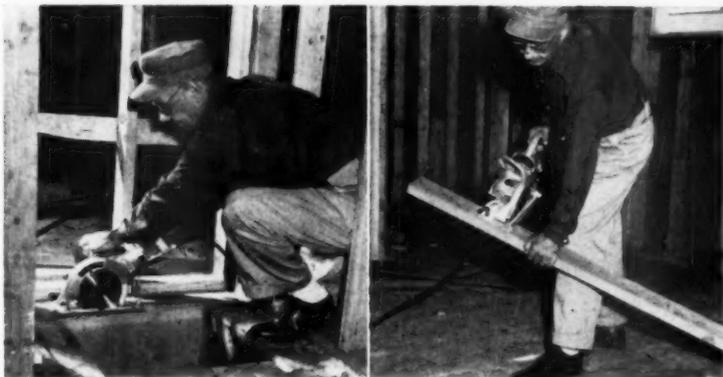
Portable power saw is also a handy tool for making quick and accurate pocket cuts in flooring for chimney, heating, ventilation or plumbing ducts
