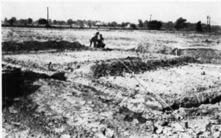
Checking the diagonals for the slab—only  $\frac{1}{8}$ -inch tolerance is allowed. Trenching for concrete footings and for plumbing is shown
