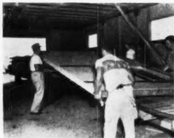
Loading wall sections on a lightweight trailer which will carry them directly from jig table to job site for erection
