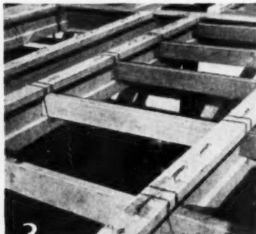
**3** Insert spreaders on about 30-in. centers to support forms. Spreaders usually are hung with wire hangers. After the forms are removed cut ends of wire hangers off flush.
