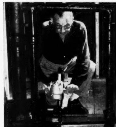
All-purpose, close-coupled drill, driving long, 1 $\frac{1}{2}$ -inch diameter auger bit, bores holes for plumbing and electrical installations
