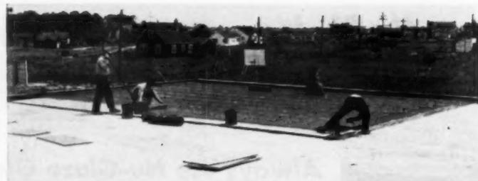
Final step in the application of the first section of insulation-board panels over a large section, is the placement of a water-stop at the fourth side of the section. Roofers go over entire area to make sure that felt adheres snugly at all seams. After this section is completed, work then proceeds on other sections of the roof deck
