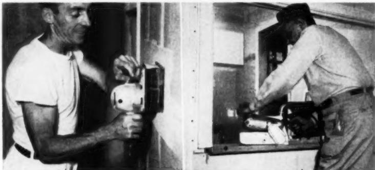
Oscillating sander is being used here to smooth taped gypsum wallboard joints. This tool is also used in wood finishing operations, and, equipped with a felt pad, speeds rubbing, polishing
