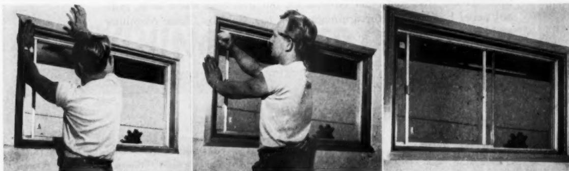
**Marking dimensions for application of newly designed metal head trim (top). Note kerf in wood surround for the snap-on application. Vertical trim is applied in kerf (center), which has a five-degree angle for tension grip. Installation is completed (right) in a matter of minutes**
