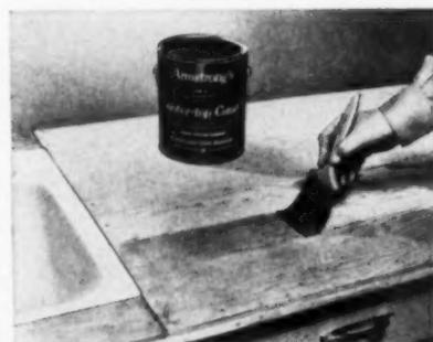
3. Spread cement on counter top and back of laminate
