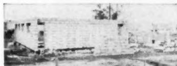
Openings for doors and windows are left in block walls. Aluminum doors and windows go in without trim. Grooves in the blocks receive flanges on the windows. Mastic is applied for waterproofing. Sash have sills attached
