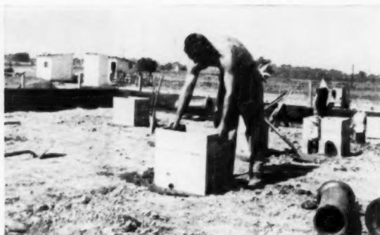
Forms for supporting piers are placed in position before the loose fill for subgrade is added
