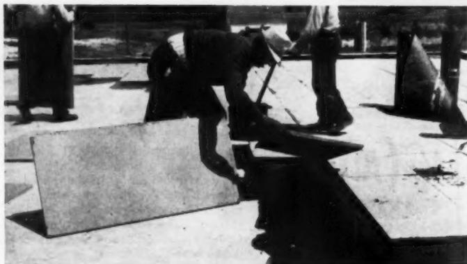
If mechanics are unable to complete the application of insulation board in a fixed working period, they then seal off the end of incompleting portions with strips of roofing felt. This serves as a water-stop and protects the installation against possible damage by a sudden rainfall
