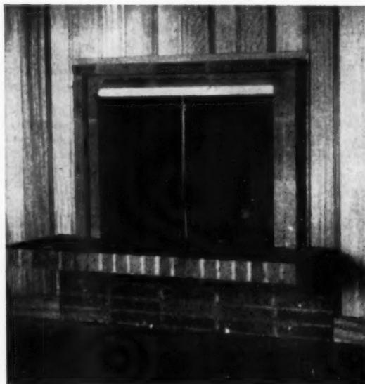
**I**N this fireplace the hearth slab is 50 inches deep and protrudes beyond the plane of the wall 20 inches. The steel goes the entire depth of the hearth slab and also crosswise between ends of the brick. The weight of the brick and steel supports the cantilevered portion, so that three or four persons could jump on it without damaging it.
