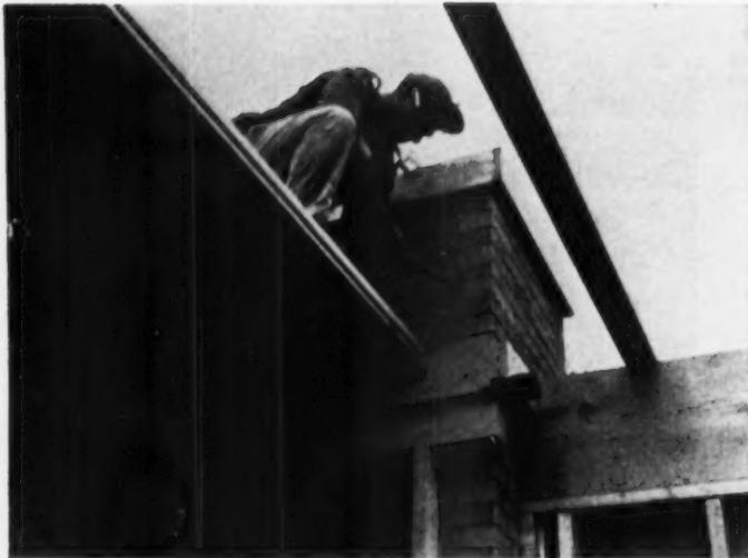
Construction of the "Readers' Choice" house parallels the advanced design of the structure. Basically it is post and beam framed on 10-foot centers. The beams are 4x16 and rest on 4x4 posts set at the exterior walls. Roof decking for the large span is 3x6 t&g industrial flooring nailed to the supporting beams.
