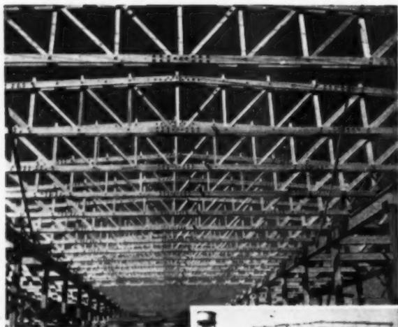
Photographs show how engineered timber construction is used in Crossett's new mill building.
