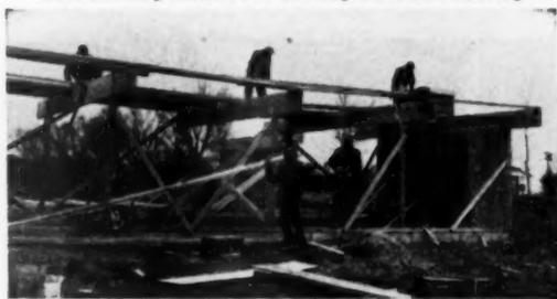
Heavyweight decking was used due to the long span between supporting beams
