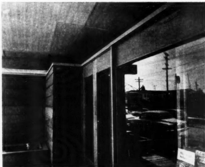
Glass between top plate of sidewall and roof can be seen in this photograph. Glass edges are lapped rather than set in wood stops. Glass line is unbroken around perimeter of building
