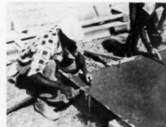
Locating the anchor bolts in finished slab (see chapter 6, June, 1952)
