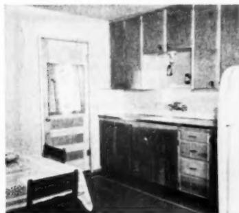
Kitchen has low-cost plywood cabinets. Its 12x12-foot over-all area provides space for dining. Cabinets and appliances align along two walls
