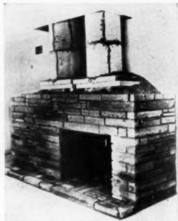
In Atkinson's houses, the pipe insulation flues are self-supporting and rise from the top of prefabricated metal fireplaces about 11½ feet to the chimney. Chimneys are wood with a fireproof stucco lining
