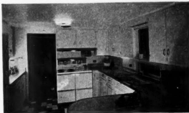
Cabinets on walls of kitchen are placed against a one-inch furring strip which forms a recess at ceiling line
