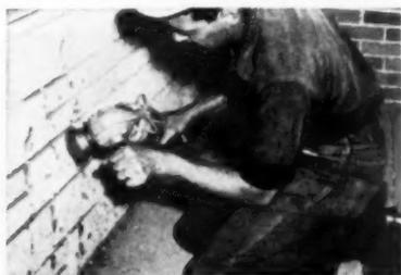
Equipped with a wire cup brush, the powered disc sander makes short work of mortar splashes and other dirt or debris
