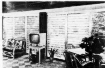
equipped with plastic weatherstripping at the head and sill where the top and bottom glass louvers compress it to a complete seal when vanes are tightly closed. Precision adjustment and exact balance assure easy operation, with free action of up to 30 louvers on a single control. Recessed inside screens of aluminum frames and mesh are held in place by easily-turned clips. All Weather Jalousies, Inc., Dept. AB, State Highway 46, Teterboro, N.J.
