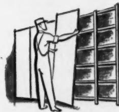
**EASIER TO ERECT.** It's less brittle, easier to nail because the Fiberglas reinforcements help hold the gypsum core together. Cut-outs come clean, edges don't crumble. Board's more resilient, too, withstands handling better, minimizes losses.
