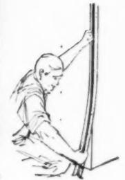
**PERF-A-BEAD**—Applied and finished with PERF-A-TAPE Cement. Metal bead provides low-cost outside corner reinforcement. Standard 8' lengths; 125-piece jumbo or 25-piece junior cartons.
