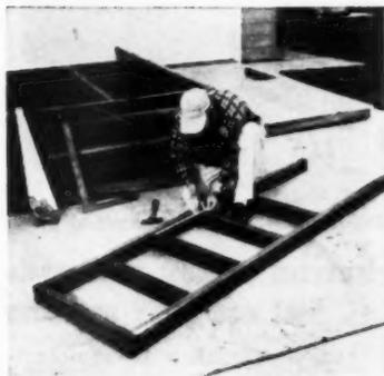
Constructing narrow frame. Width is 27 $\frac{3}{4}$  inches. Height is 64 inches
