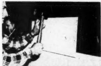
Mechanic installs shingle using "hook nail," a recent development of The Flintkote Company
