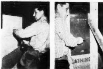
Photo above shows installation of insulating siding over fiber board or gypsum board sheathing. Black painted galvanized or electro-plated copper twist nails are used to secure vertical joints between studs. Nails must be twist clinched (see photo right) on back side of sheathing before inside wall is finished. Use 2 1/4-inch 11 1/2 gauge black painted siding nails or aluminum nails (etched or plain) at studs only.
