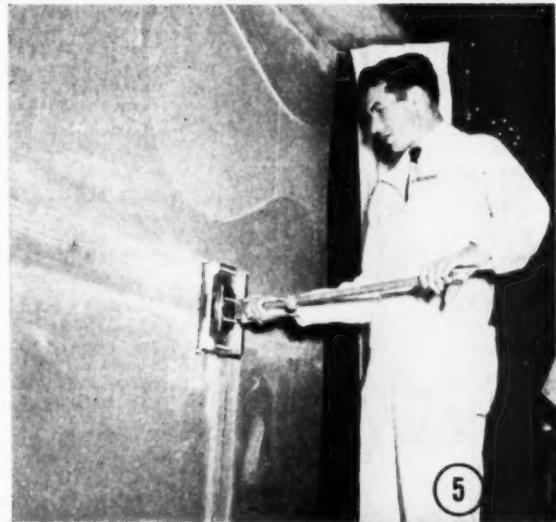
5. Mechanic finishes horizontal wallboard joint with 12-inch hand finisher.
