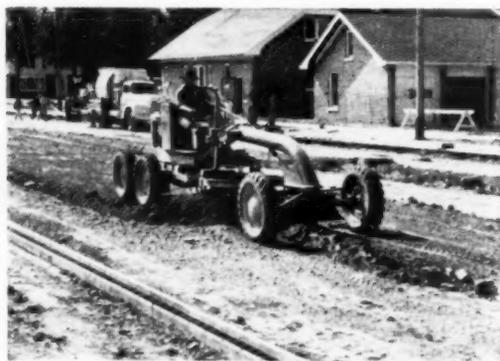
**ROUGH GRADES** for curbs, gutters; finish grades shoulders, sidewalks, between forms; cuts and cleans drainage ditches; removes weeds and brush.
