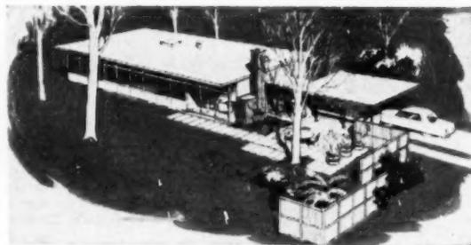
Roof slab is supported by columns independent of the exterior walls. This permits continuous window fenestration in the wall. The cantilevered roof slab makes possible wide overhangs
