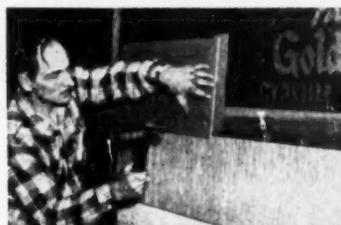
Here workman demonstrates "horsefeather" method for applying asbestos cement siding shingles
