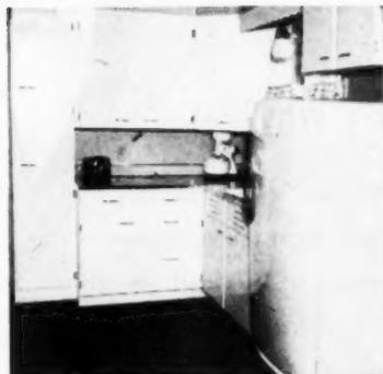
Kitchen cabinet corner has recessed fluorescent light over sink top, with steel casement window in back
