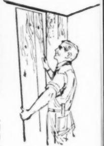
**USG METAL TRIM**—Nail on for narrow line effect. Provides enduring edge protection; ideal for door and window trim or molding at ceiling and wall line. 7' and 10' lengths fit  $\frac{3}{8}$ ",  $\frac{1}{2}$ ", and  $\frac{3}{4}$ " thickness. Also  $\frac{3}{8}$ " pre-decorated type to harmonize with Striated or Knotty Pine finish boards.
