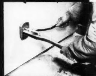
Insert cutter—SQUEEZE HANDLES TOGETHER
