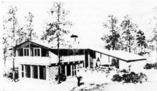
This split-level house takes full advantage of a sloping lot, featuring a patio on the lower grade, front entrance at the intermediate level, and a kitchen "housewife supervisory" area on the top level. Structural steel frame of basic house is exposed along side walls
