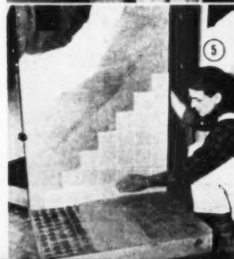
1. Shown are two of three basic types of clay tile. Three types are: (a) 4 1/4 x 4 1/4 inch glazed, square; (b) ceramic mosaic; (c) quarry.
