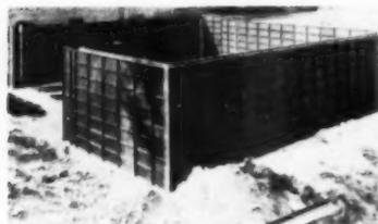
steel frame is only 2½ inches, as compared with 4¾ inches for wood frame forms. The manufacturer has developed a simple, easy-to-follow procedure that enables a contractor to build his own concrete forms in the field, using the frame and purchasing his plywood panels locally. Symons Clamp & Mfg. Co., Dept. AB, 4249 Diversey Ave., Chicago 39, Ill.
