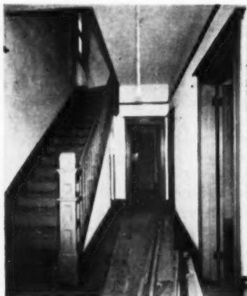
This is the typical foyer of houses built in the late 19th century. The builder was able to make separate entrances to the duplex apartments by putting a partition next to the stair
