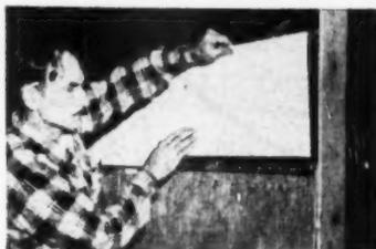
Channel strips fit over head edge of under-course shingles; are held in place with "hook-headed" nails
