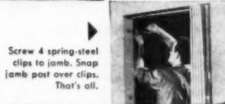
Screw 4 spring-steel clips to jamb. Snap jamb post over clips. That's all.
