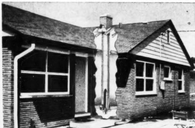
SECTIONAL CONSTRUCTION saves 30% to 50% on time and material over brick chimney cost. The Van-Packer may be placed directly over furnace in center of house as easily and inexpensively as against a wall.
