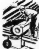
3 Cement remaining sections in place until desired height is reached.
