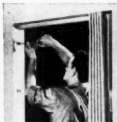
**Step 2.** Screw in jamb clips, attach jamb post to them. No planing or fitting necessary.
