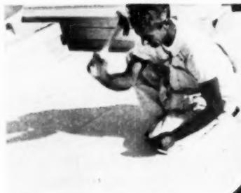
Large-headed galvanized nails, long enough to penetrate the framing members at least 1 1/2-inch, are used to apply the 2x8-foot roof deck sheets
