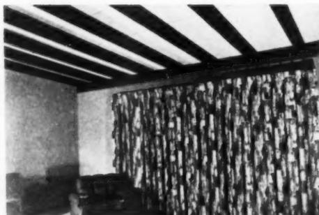
The living room ceiling in this home is the finished surface of the underside of the roof panels. These panels combine three functions in one—roof decking, roof insulation, and a prefinished interior ceiling
