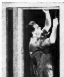
**Step 1.** Slide head track onto trolleys, raise door to standing position, fasten it in place.
