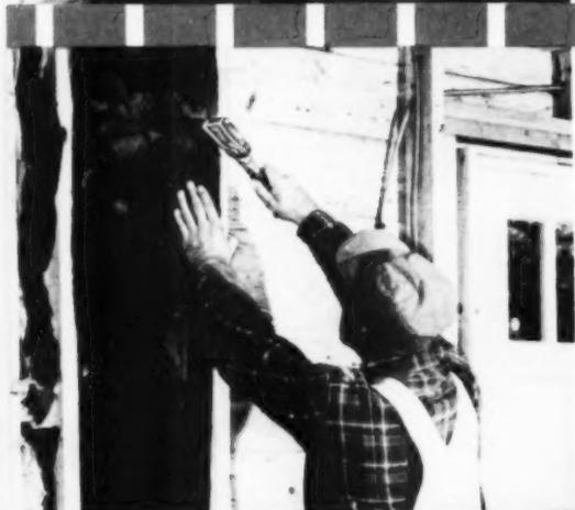
**FASTER FOR** installing batt, blanket and reflective insulation . . . applying cornerite and metal lath . . . applying wooden undercourse shingles on outside walls (H2B-1/2) . . . applying felt and waterproof paper to outside walls prior to siding.
