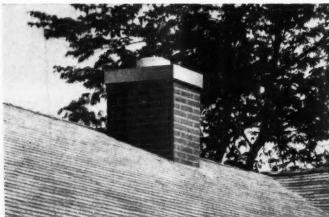
BRICK-PANEL Van-Packer Chimney Housing has "buyer acceptance" of a conventional brick housing. Brick-red cement asbestos panels have deep embossed brick texture and natural color mortar lines.
