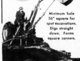
Minimum hole 36" square for spot excavations. Digs straight down. Forms square corners.
