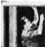
Cut drilled track to opening width. Mark and drill holes in header. Slide track onto door and lift into opening.
