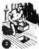
2 Nail chimney support in place. Cement first 24" chimney section in support.
