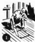
1 Cut holes in floor, ceiling and roof. No clearance to wood members necessary.
