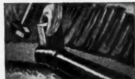
1/2 Bend connected to Orangeburg Pipe making a 45° turn. The famous Orangeburg Taperweld Joints are leak-proof and root-proof.
