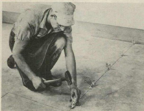
Attach base clips to floor every 12 or 16 inches, centering them on a single line. Slotted hole in floor permits adjustment of clip
