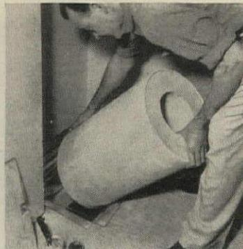
Flue sections made of  $\frac{5}{8}$ " fire clay tile inner lining, 3" vermiculite-concrete insulating wall, and cement-asbestos outer jacket. Here first 2' section is installed in support.
