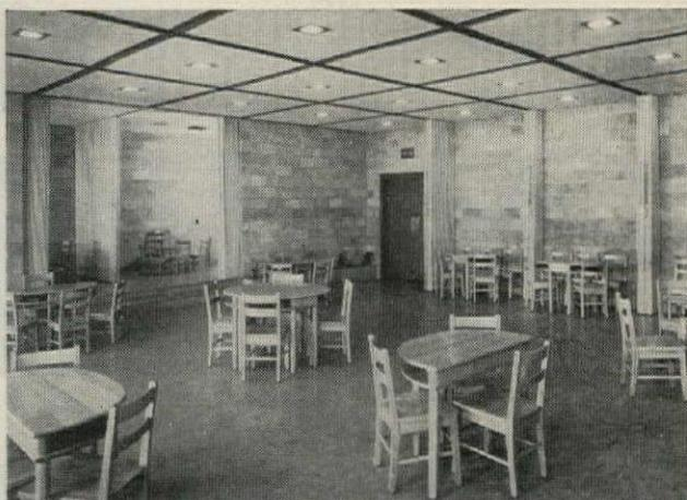
Classroom presents great flexibility of space arrangement. Ceiling grillework is made of tracks upon which folding doors slide to divide room into rooms of almost any shape or size desired.
