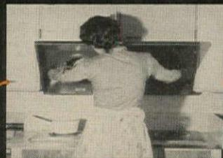
To clean, merely turn two fasteners and tilt
