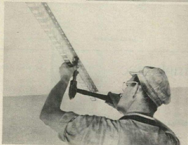
Attach runner to ceiling, using ½-inch stub nails. Web is perforated with two rows of 9/16-inch holes to permit keying of plaster
