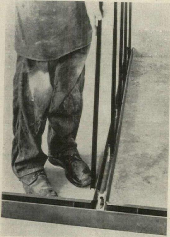
Insert channel studs in base clips, raising channel up to ceiling and placing bottom end of channel onto prong in base clip, which holds it in place. Can be removed in same manner
