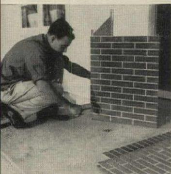
Brick-red cement-asbestos panels are cut to roof pitch, then assembled with corner angle irons and sheet metal screws provided.
