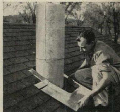
Aluminum flashing is installed on the roof. Van-Packer's "Brick-Panel" Housing over its aluminum flashing gives chimney a weathertight seal.
