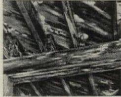
**CUT COSTS 70%?** You can . . . with new Shakertown GLUMAC Units! Such savings are not exceptional with these deep-grooved, factory-stained shakes which are electronically bonded to a tapered, asphalt-impregnated backer board. In big, easy-to-handle 16" x 46<sup>3</sup>/<sub>4</sub>" panels, GLUMACS complete a "double-coursed" shake sidewall up to
