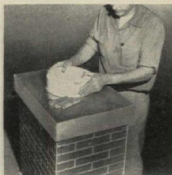
Aluminum housing cap, chimney pot and refractory rain cap are added to complete installation. Van-Packer develops 34% more draft than standard code brick chimneys.
