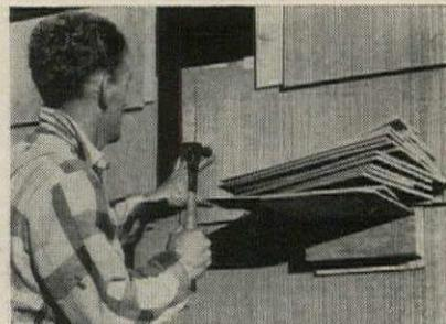
Platform in place, showing how top of platform face fits under 1/2-inch projection of top shingle course
