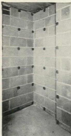
*Gemco Anchor Nails* firmly installed on concrete block wall with waterproof *Tuff-Bond Adhesive*.
