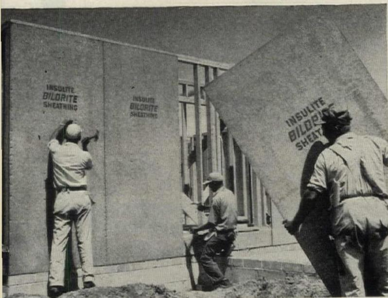
**Bildrite saves \$106 per 1,000 sq. ft.** on Mr. Bacchus' 700-home Sunrise Park project. With Bildrite, one man can sheath 1,000 square feet in 8 hours or less. Cuts application time as much as 43%. Four-foot wide Bildrite eliminates the need for corner-bracing (F.H.A. accepted). Since Bildrite is waterproofed throughout with asphalt, there's no need for building paper; can be exposed to weather indefinitely.
