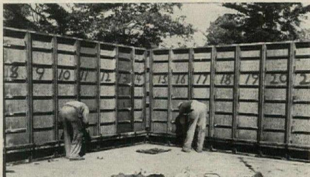
Fast form erection gains new importance when home builder concentrates on all-concrete houses. Careful numbering of forms speeds the operation
