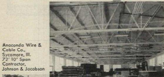
Anaconda Wire & Cable Co., Sycamore, Ill. 72' 10" Span Contractor, Johnson & Jacobson
