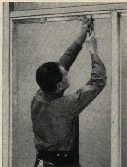
**1. Mount track to header.** (Grant 7000 Sliding Door Hardware Sets feature extruded aluminum track, cut to size, properly drilled for mounting. All parts contained in dust free tube. There's a style and size for every need.)
