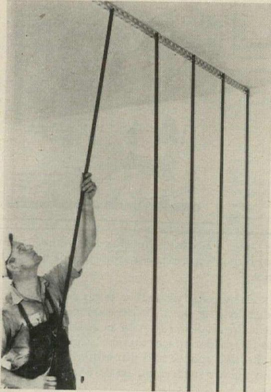
Insert channel studs in  $\frac{7}{8}$ -inch slot in ceiling-runner at intervals corresponding to position of base clips on floor. Channels fit snugly, yet vertical movement compensates for variations in ceiling height up to two inches
