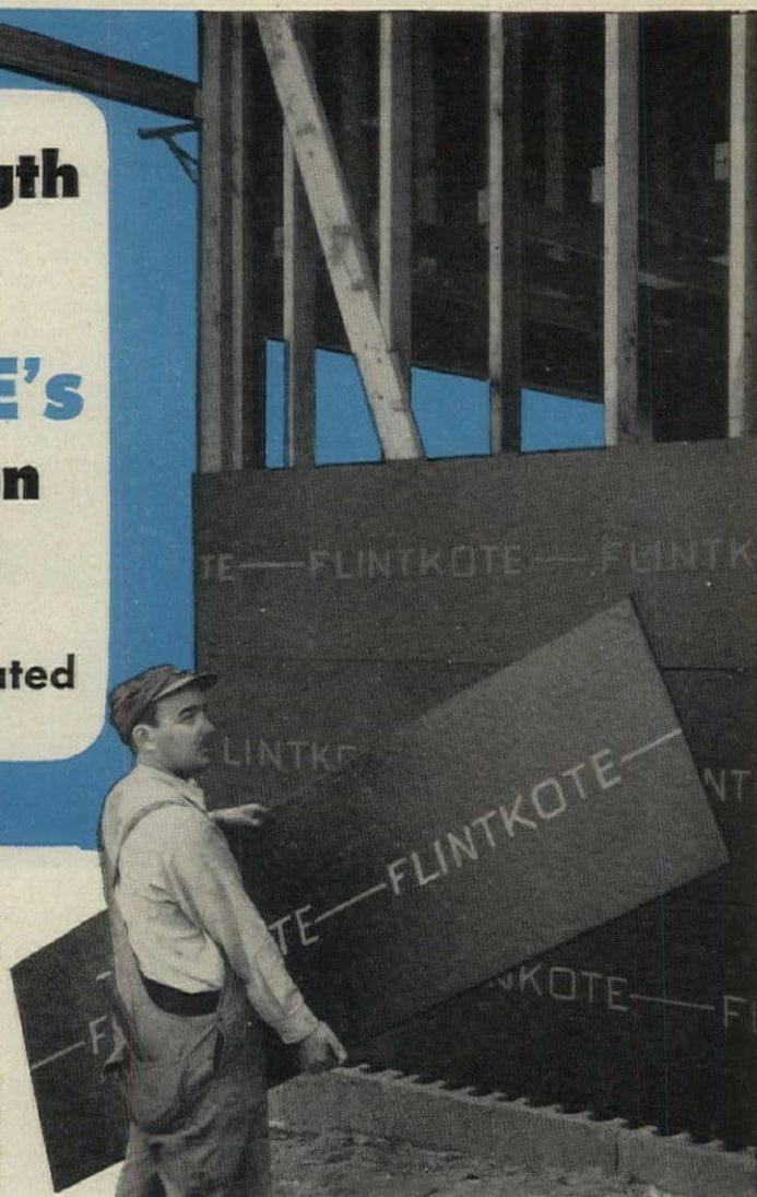
To protect insulation sheathing board from rain and moisture—in transit or on the job site, prior to and during application—it is desirable to have both the core impregnated and the surface coated with asphalt.
