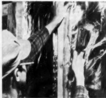
Here is a stapling hammer being used to secure multiple accordion insulation to wood studs. Space between studs allows enough room for hammering movement with this stapler
