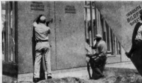
**First, apply Bildrite—cut sheathing time as much as 43%.** One carpenter can sheath 1,000 sq. ft. in 8 hours or less. 4' Bildrite has more than twice the bracing strength of horizontal wood sheathing, thus eliminates need for corner-bracing. No building paper required since Bildrite is waterproofed throughout with asphalt.
