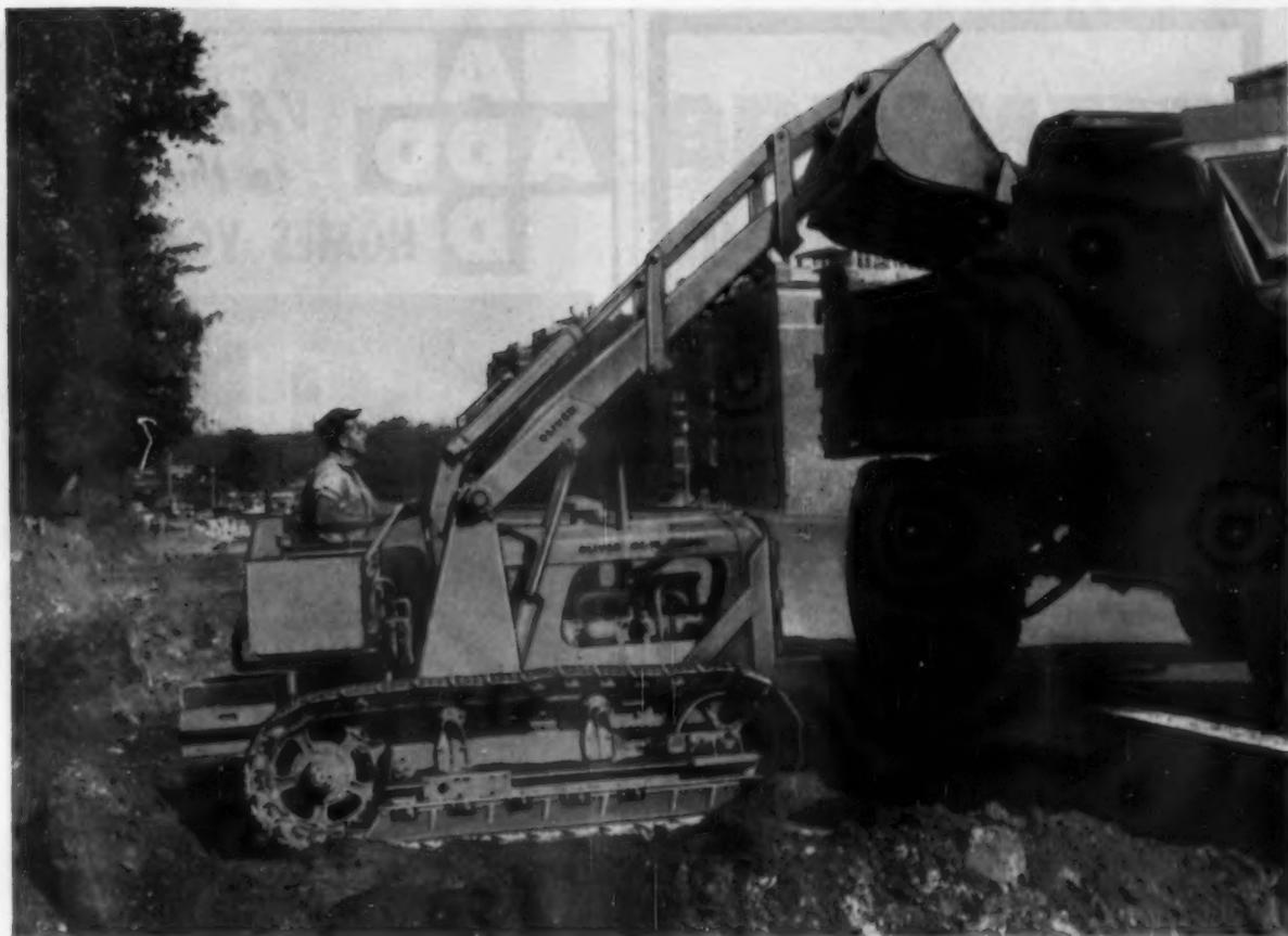
Oliver "OC-12" with hydraulic 1-yd. loader. This model has the long track frame for added stability. Loader has exceptional bucket rotation and 10' 4" loading height.
