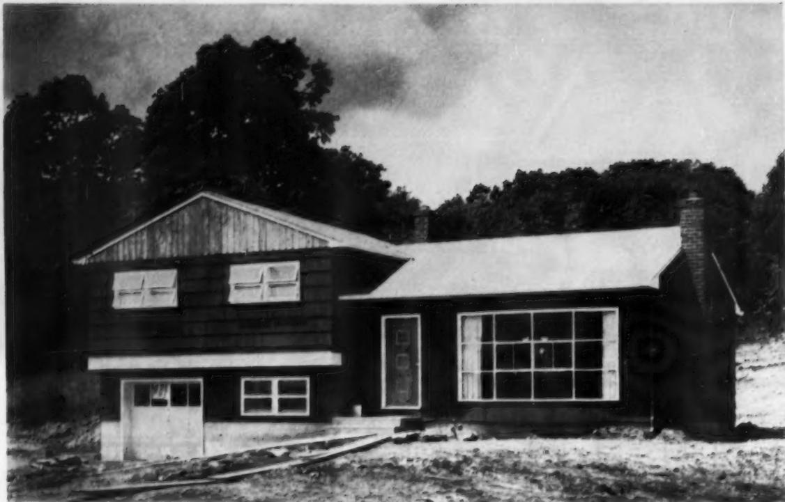
Split level models such as this helped Bogdanoff adapt houses to hilly sites. In some cases garage was dropped four feet to accommodate steep slopes. Variety was achieved by reversing plan, altering roof lines
