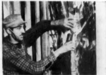
In extra-wide stud spaces where the panels of accordion insulation must be joined together to close up a space, a stapling plier is used for fastening the flange surfaces together
