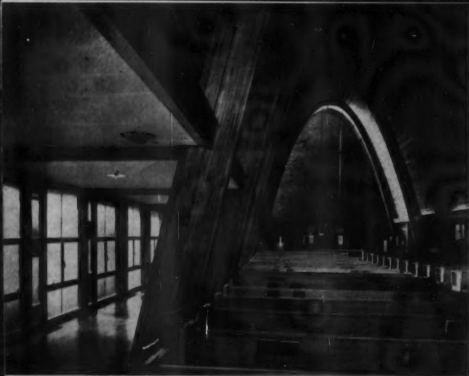
Parabolic in shape, laminated rafters form the skeleton and shape of interior. Two-inch depression in brick wall over altar is to receive future ceramic mosaic
