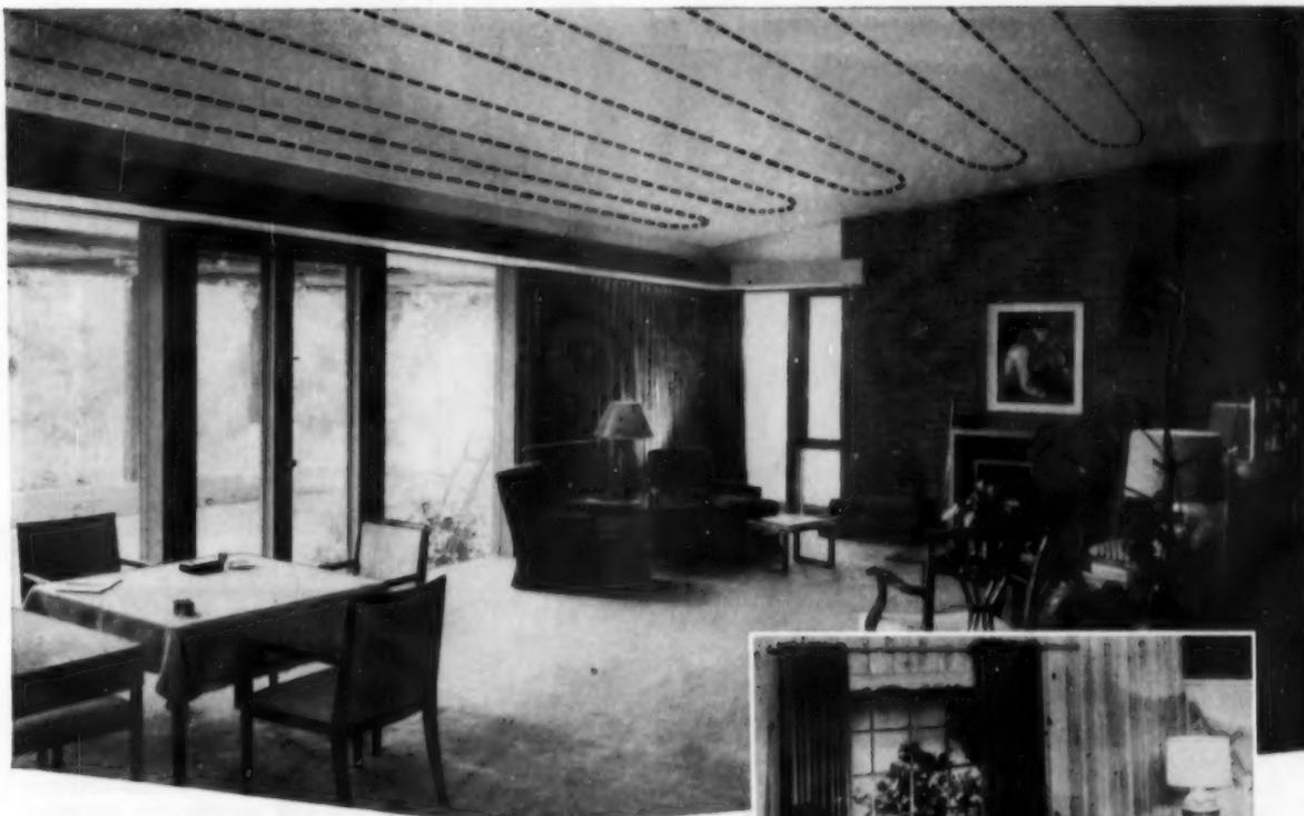
Invisible coils in ceiling or floor.
