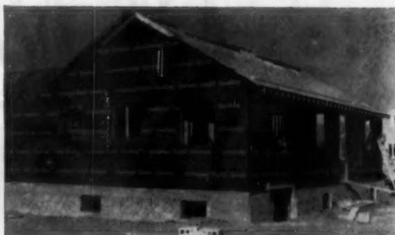
**No costly delays from rain.** Rainstorms will never knock a big hole in your construction schedule when you use Temlok. The new Rain-Shield® coating, plus asphalt impregnation, completely seals every square inch of Temlok against water. When storms are over, work can be resumed almost immediately. Temlok is clean to handle . . . leaves no gummy coating on carpenters' hands and saws. \* Trade-Mark
