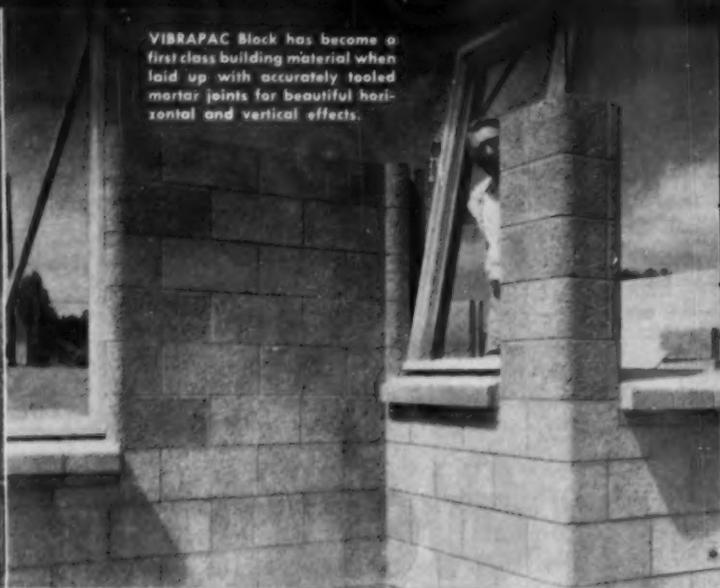
With VIBRAPAC Block, it's so easy to build small closet space and interesting patterns of short walls, using stacked bond coursing.
