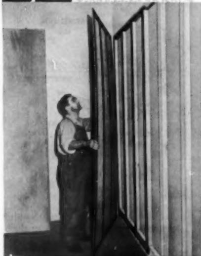
**Important Building Economies** — Now, the world's largest plywood organization brings you a revolutionary new concept in building construction. With Weldwood Contact Cement you can put up plywood paneling entirely without nails! Ends nail-setting, puttying and finishing unsightly nail holes. No change in plans needed! No special construction needed. Install plywood panels directly to studs or furring strips.
