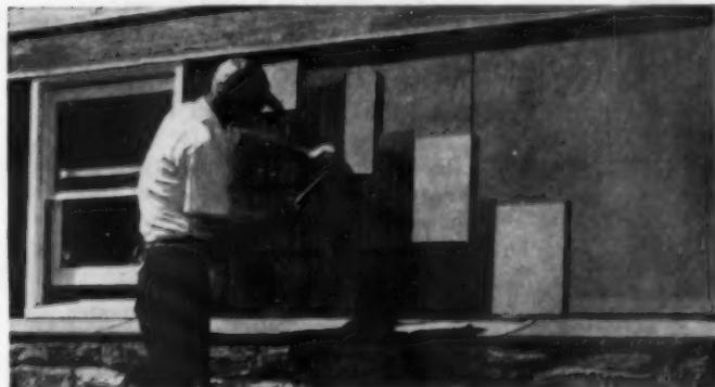
**Next, apply Shingle-Backer in half the time** required for wood under-course shingles. Handy 4' panel produces deep, modern shadow-line. Practically eliminates waste. Adds extra insulation value to sidewall. Can be used or stored anywhere in any weather—it's waterproofed throughout with asphalt.
