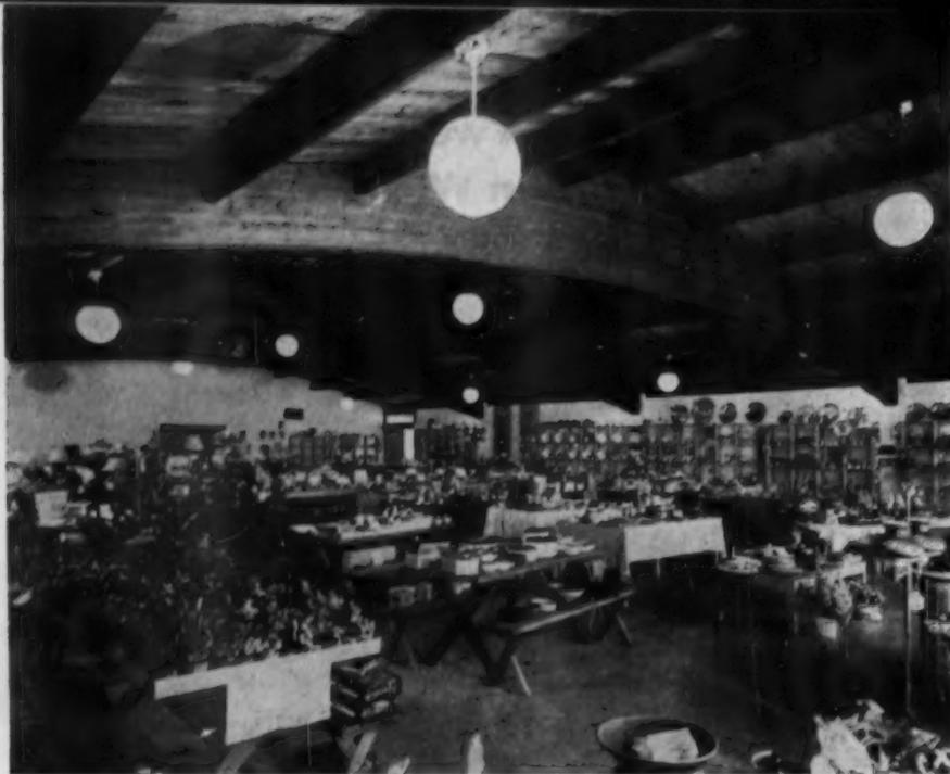
◀ Arch of glued, laminated beams creates a feeling of space, allows for better vision into the large sales floor, and avoids the effect of too-low ceiling. Exposed decking is warm, attractive enough so that intermediary ceiling between sales floor and roof framework is unnecessary
