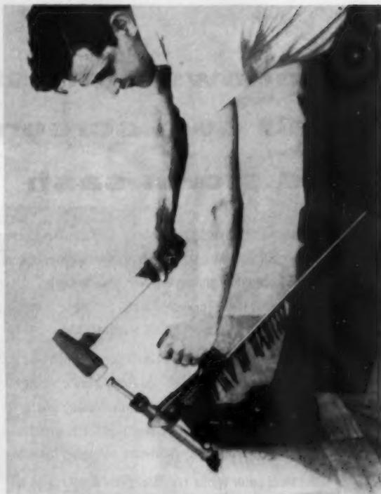
The Screw-tite floor nailing machine makes it possible to lay T & G floors better with a saving in time and labor and without banged up edges or mashed tongues. The machine feeds the nail at the proper angle, drives and sets nail and drives flooring snugly into place
