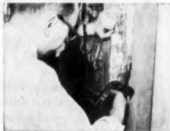
A spring-driven stapling tacker is used to fasten accordion aluminum insulation to wood studs where there is not much more than several inches of space in between the studs to be covered
