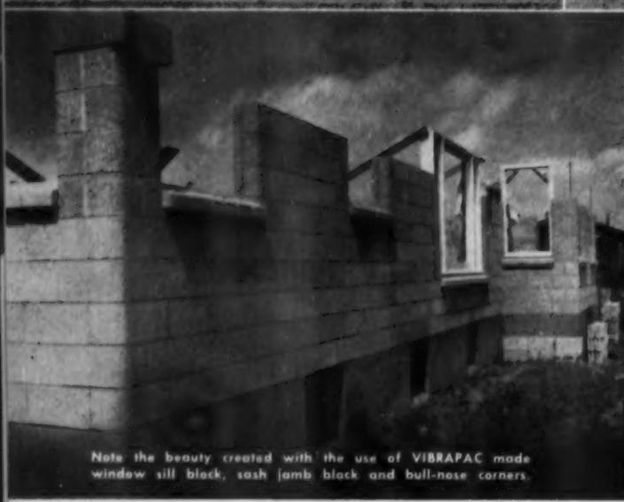
Note the beauty created with the use of VIBRAPAC made window sill block, sash jamb block and bull-nose corners.
