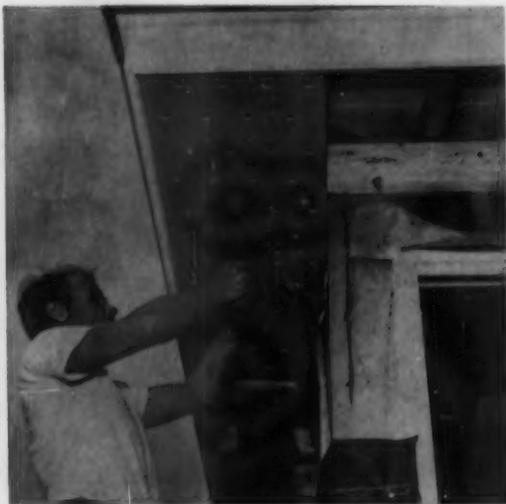
**FIRST STEP** in eave plastering, after installing 2x6 ribbons, blocking and vents (Fig. 2, upper right), is to apply rocklath. Knuckle-bustin' job of notching lath around rafters in open-end eaves is eliminated.
