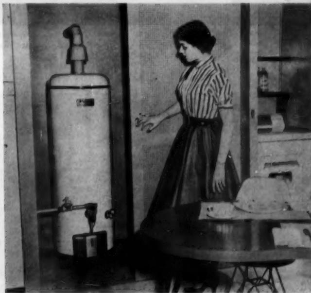
**DIALED TEMPERATURE**, long life and fast supply are points stressed by Ruud-Alcoa Alloy heater. Solid aluminum alloy tank resists corrosion and is free from rust formation. Heater automatically provides water at the dialed setting.
