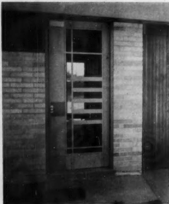
A change of pace is indicated in the width of the rails and stiles of this door. The center cross members protect the screen wire while adding design value to the door. The frame as detailed in the adjoining drawings can be used for a brick veneer or cavity brick wall
