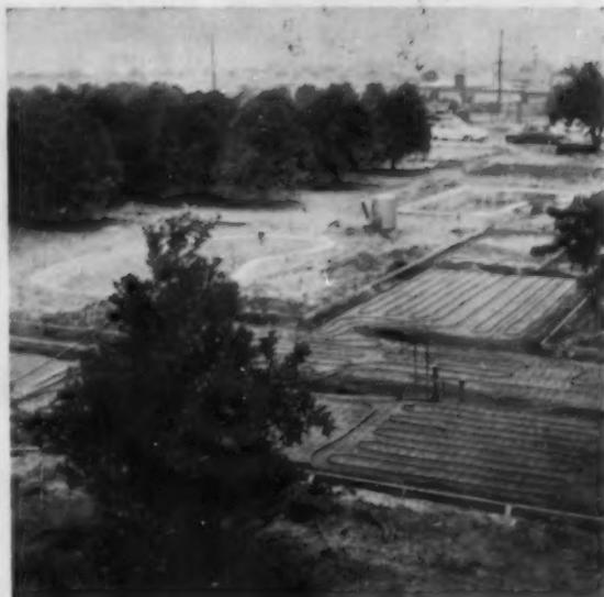
The houses are heated with radiant heat coils embedded in the concrete slab floor. This same system is extended out into the concrete area surrounding the pool and into the pool to heat the concrete and water
