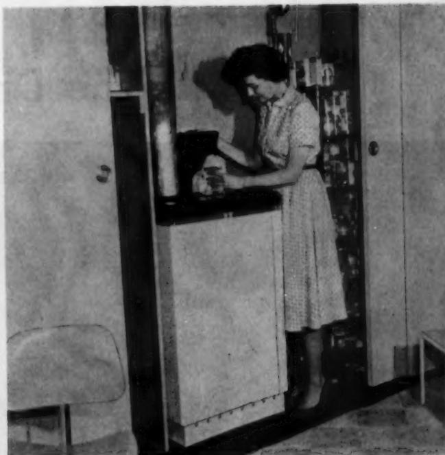
**INCINERATOR**, Brule Model M-1, is at exterior wall side of service lounge and has its own vent through an annular flue collar. Air-cooled sides are safe to touch. Utility meters and more storage shelves share rest of wall space.
