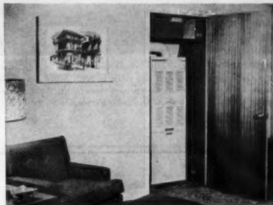
**CLOSET** is comfortable berth for Lennox upright gas-fired furnace, or for counterflow with under-floor ducts. And either type has ample room for add-on air conditioning, as shown at top of closet, using furnace's blower.
