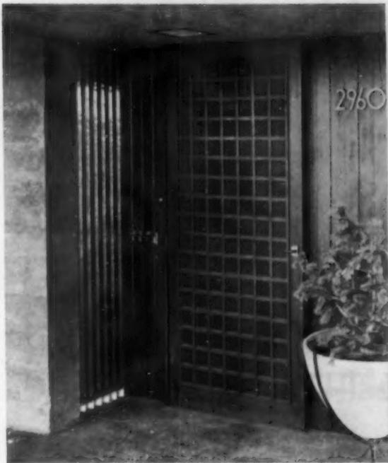
This grid-patterned screen door is hung from the end face of the door frame. The frame can be built of 2x6 or 2x8 inch members, depending upon the adjoining materials
