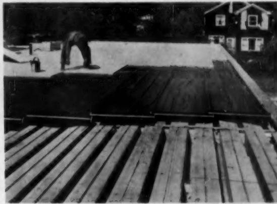
Fibreboard insulation is placed over Koroseal after a mopping of Lexsuco adhesive
