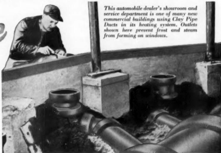
*This automobile dealer's showroom and service department is one of many new commercial buildings using Clay Pipe Ducts in its heating system. Outlets shown here prevent frost and steam from forming on windows.*
