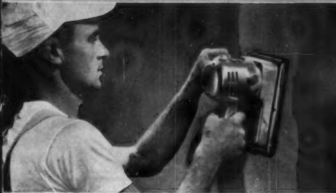
Black & Decker 88 Sander sands joint seams in dry-wall construction satin-smooth in a fraction of the time of old-fashioned hand sanding.
