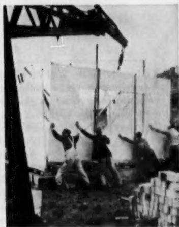
Wall is lifted by crane for placement on hardwood floor joists
