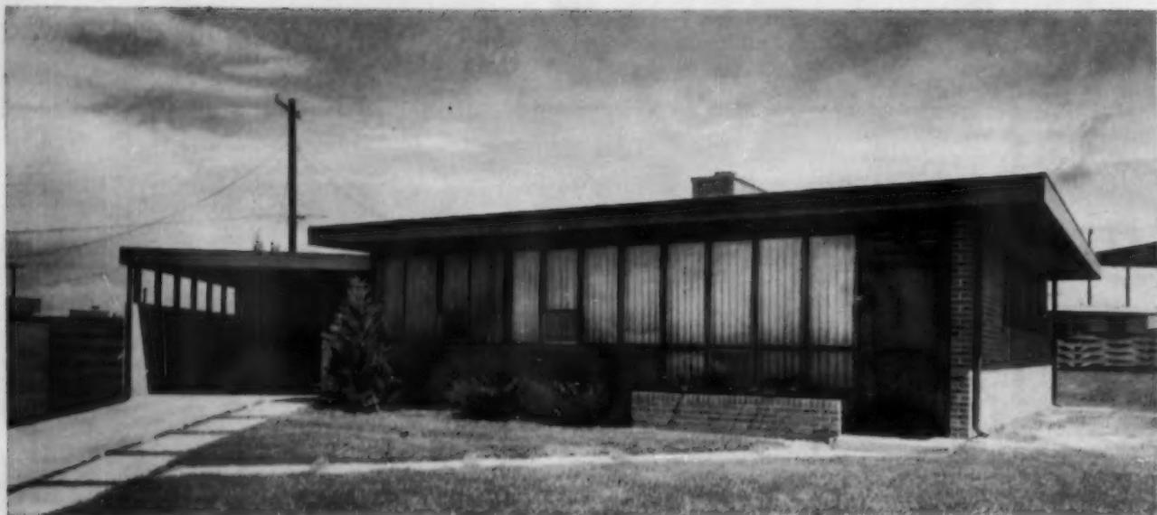
**\$14,000** Brick cavity walls with a combination of face brick and plywood for the interior finish
