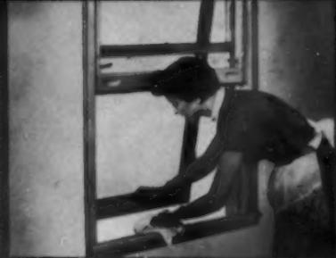
**Cleaning and painting is a cinch.** The entire window unit swings out for easy sill cleaning. Or you can lift unit off entirely for painting.
