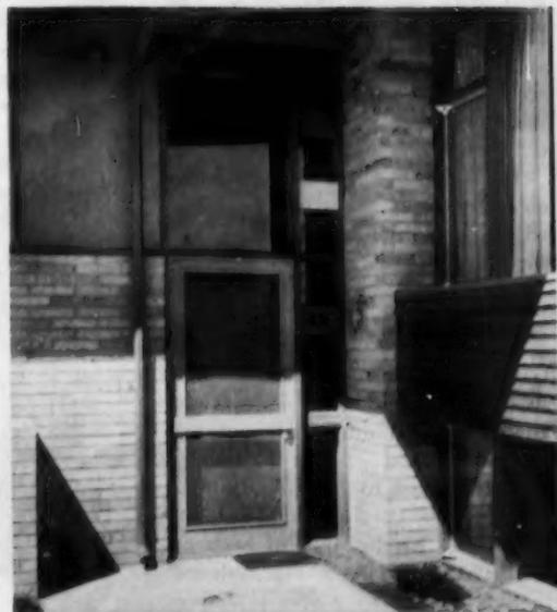
An effective design of screen door, sidelights and transom for a split-level house, with a minimum width required for mullion and transom. The drawing of door frame and adjoining window, left, shows how the door extends across the face of the frame. This can be easily changed to conform to the photo where a 1 1/2-inch rabbet is provided in the frame
