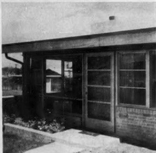
A simple screen door design with a minimum width for rails and stiles. This screen door is particularly effective when used in conjunction with a slab type of exterior door. The drawing of door frame and adjoining window on opposite page is applicable to this installation
