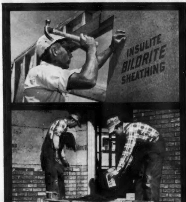
**Bildrite goes up faster, easier.** One carpenter can sheath 1,000 square feet in 8 hours or less with Bildrite. Cuts application time as much as 43% compared with wood. Adds strength. 4' Bildrite has more than twice the bracing strength of horizontal wood sheathing, thus eliminates corner-bracing. Waterproofed throughout with asphalt. No need for building paper. Can be used or stored anywhere in any weather.
