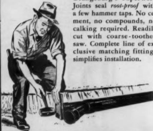
Orangeburg's Taperweld Joints seal *root-proof* with a few hammer taps. No cement, no compounds, no calking required. Readily cut with coarse-toothed saw. Complete line of exclusive matching fittings simplifies installation.
