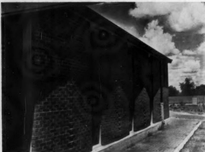
Splayed wall panels were laid on a straight-walled foundation. Front and rear elevations of chapel are built with bent walls, too. Plan of wall construction and window detail are shown in drawing
