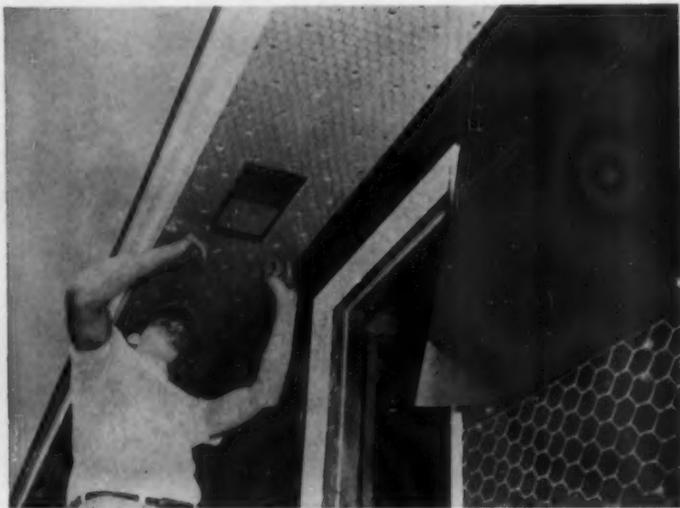
**MESH IS NAILED** at same time that lath is applied. Openings are cut for vents, and mesh is carried short distance down sidewall to provide good ground for stucco. Mesh is then applied over sheathing paper.
