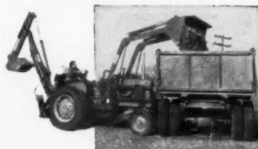
The Henry Hydraulic Tractor Shovel, with its five attachments—utility bucket, manure fork, hoisting crane, dozer blade and fork lift—has no equal for versatility. At the same time its solid steel lift arms and rugged construction enable it to meet the heaviest of demands.
