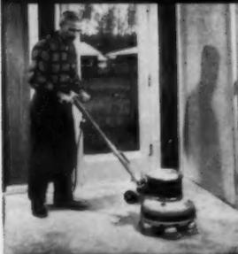
Wire brush quickly removes mortar, paint, plaster droppings.
