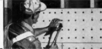
For smooth, fast plastering, specify Certain-teed Beaver® Gypsum Lath. Both plain and perforated. Strong—fireproof. Beaver Insulating Gypsum Lath with aluminum foil back provides insulation and an effective vapor barrier.
