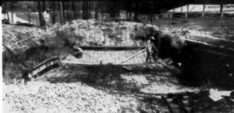
Excavation for pool showing steel reinforcement for floor and inside pool walls.
