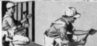
Certain-teed Bestwall® Gypsum Wallboard comes with plain or predecorated wood-grain finishes. For fire-rated construction with single layer application, use Firestop Bestwall,® 5/8" thickness gives 1-hour fire resistance.
