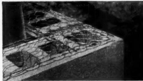
**Key-wall** is lapped at corners without adding thickness to the joint. Quick and easy to do. Provides exceptionally effective reinforcement of corner.
