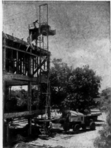
**Self-raising "Hoister" tower handles loads up to 2000 lbs:** You can have it with either material cage or 14 ft. concrete bucket, and in 10 ft. sections for heights to 67 ft. Self-raising up to 37 ft. Moves around on skid base. Positive automatic safety device prevents falling even if cable breaks.
