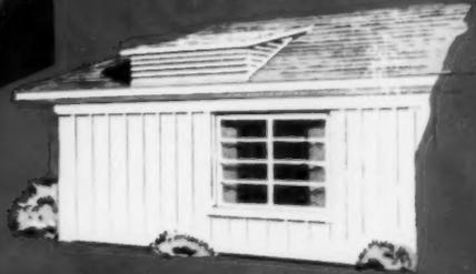
Houses of hip-roof design require only inclusion of an inconspicuous dormer to accommodate the unit.
