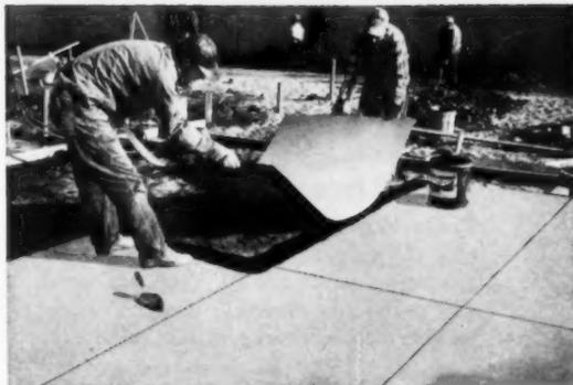
**IDEAL FOR ALL CONSTRUCTION APPLICATIONS...** Premoulded Membrane, supplied in 4' x 8' sheets, is laid directly over the hard tamped<sup>®</sup> grade with a 6" overlap. This overlap is then sealed with Sealtight Catalytic (non-setting) Bonding Asphalt—giving you a monolithic vapor seal that will expand and contract with the slab above . . . without breaking the seal. You actually form a vapor proof "saucer" into which the concrete is poured.
