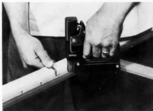
Besides flanged ceiling tile, flashing paper, insulation and metal lath, Bostitch T5-8 fastens screening much faster than other methods. Free hand holds fabric taut for perfect tension control.
