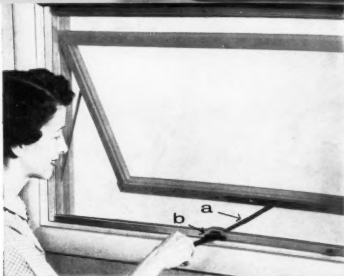
**Strong, spring steel operator arm** moves through housing, attaches to deflection bar anchored to sash bottom rail. Note arm is hinged in two places (a & b), permitting three open sash positions without extending into the room.
