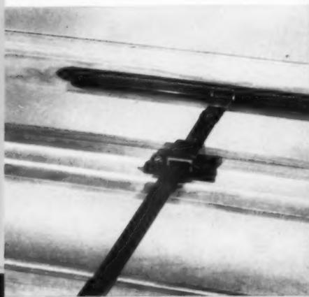
**Operating arm** is instantly detachable from deflection bar to permit wide opening of sash—an important safety feature—also makes it easy to clean glass from the inside.
