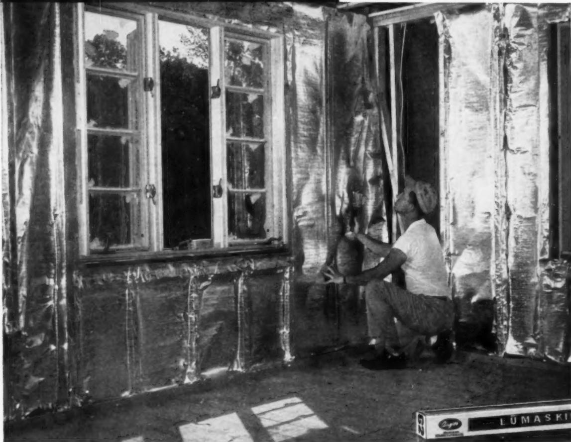
*Lumaskin conforms best to studs because it's the only low cost aluminum sheet that's creped-to-stretch.*
