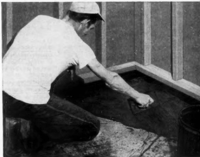
1 Spread mastic over waterproofed slab.
