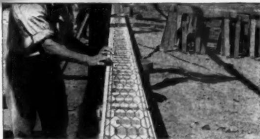
**Key-wall** is made for the following wall thicknesses: 4", 6", 8", 10", and 12".
