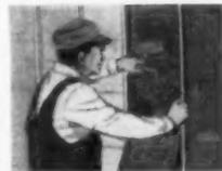
Flintkote Insulating Wool, made of Fiberglas\*\*, is quickly and easily installed in new and old houses. Available in handy sizes and forms. Insulating wool is clean and light in weight. Will not rust, rot or mildew. Won't attract vermin . . . fire-resistant.
