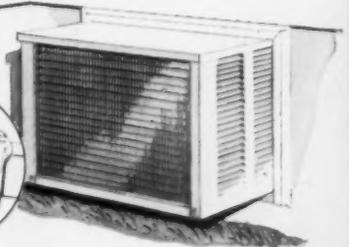
Many builders have successfully tied the unit into existing furnace ductwork by installation through the basement wall. This particular type installation offers reduced cost in duct runs.
