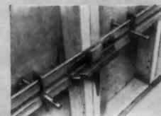
ROCFORM metal walers are permanently bolted into forms. Sections lock together with patented clamps.
