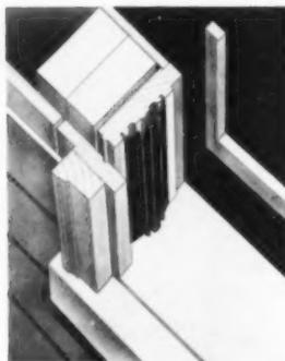
$\frac{1}{2}$ " outside sheathing and dry-wall ( $\frac{3}{8}$ " or  $\frac{1}{2}$ " inside on 2 x 4's, cut-off rib on blind stop and remove inside jamb strip.
