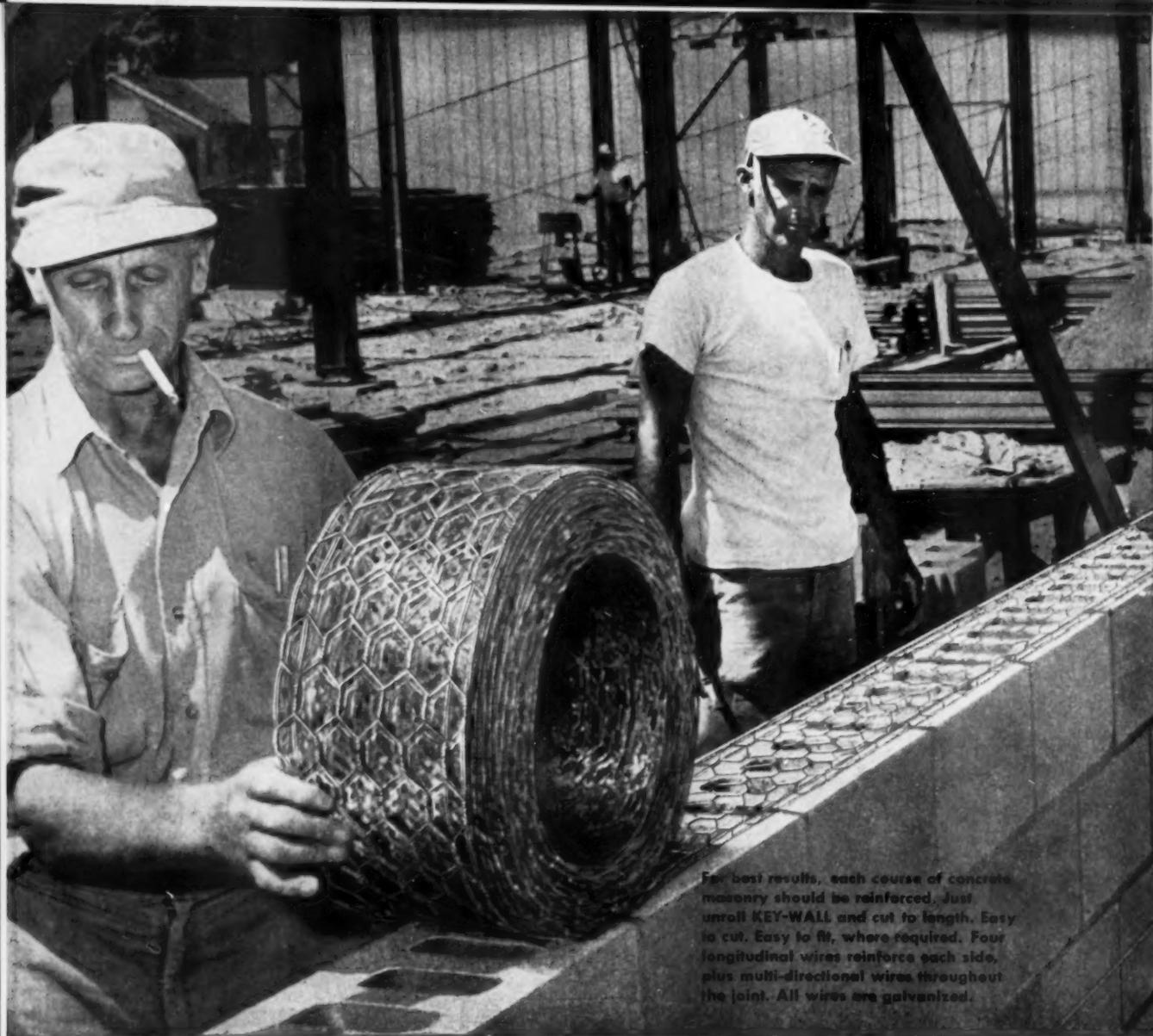
For best results, each course of concrete masonry should be reinforced. Just unroll KEY-WALL and cut to length. Easy to cut. Easy to fit, where required. Four longitudinal wires reinforce each side, plus multi-directional wires throughout the joint. All wires are galvanized.
