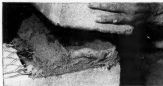
**It is easy** to build up reinforced corners with **KEY-WALL**. Short lengths may be cut and used without reducing effectiveness of reinforcement.
