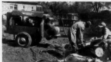
**Jaeger compressors do many jobs:** A Jaeger rotary "125", or smaller, reciprocating type "75", supplies portable power to run air saws, wrenches and hammers, concrete breakers, backfill tampers, sump pumps and many other builder's tools. Noted for low fuel consumption and full output at slower engine speeds. Catalog JCR5.
