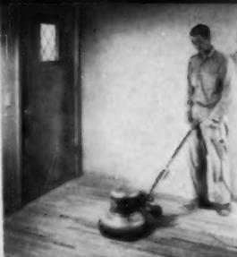
Steel wool removes excess seal, produces satin finish.
