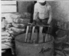
Mix different coat or color in extra tub, using same motor and base. Mixing keeps up with workmen easily.
