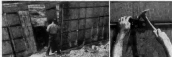
**Speed erection and stripping**—16-24 manhours for stripping, transporting, setting, and pouring of walls, plus layout and pouring of footing for next day's job.
