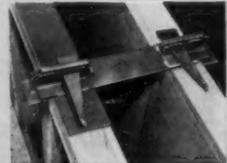
Patented wall aligners automatically give wall of uniform desired thickness and line up tops of panels.
