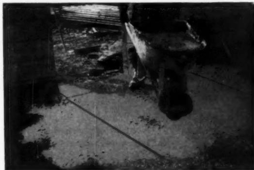
**QUICK, EASY INSTALLATION...** Premoulded Membrane is a strong, permanent vapor seal that will resist the trundling of wheelbarrows and the impact of aggregate during the pouring operation . . . best of all, with Premoulded Membrane you don't need an expensive underlayment of sand to absorb shock. This strength to resist tearing and puncturing is very important . . . as a vapor seal is much like a child's balloon, for only a small hole renders it useless.
