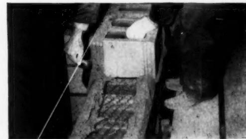
**Masons like** the ease with which block can be laid when they use **KEY-WALL** as reinforcement. The mesh helps hold the mortar in place.
