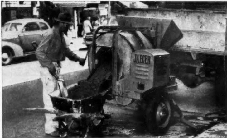
**Same wages . . . 12 to 15 yards more concrete:** Fastest half-bag mixer built—the 3 1/2 S Auto-Loader. You load while you mix, then charge in a flash with automatic shaker hopper. Has equally fast discharging action and same rugged construction as Jaeger 6S, 11S and 16S power loaders. Ask for Catalog.
