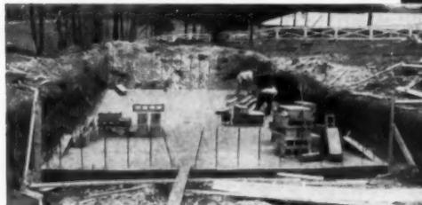
Vertical pre-stressing steel rods are ready for specially grooved pre-cast wall sections to be placed over them. No heavy construction equipment needed. All work can be done with common labor.
