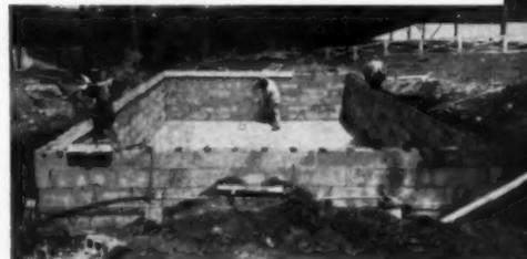
Walls being pre-stressed by tightening nuts above plates of sheet steel, after concrete mixture has been poured inside pre-cast concrete sections. Prevents cracking. No wooden or other forms needed.
