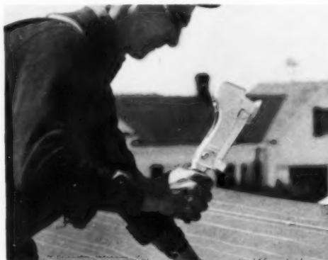
Bostitch H4 saves one-fourth the time in laying asphalt shingles. One hand is free to position the shingle or to maintain balance on steep roofs. Also speeds application of metal lath to studding, plywood underflooring, built-up roofing, etc.
