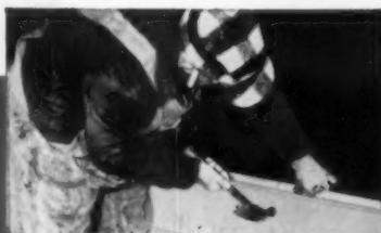
Mounting strip nailed over sheathing eliminates countersinking, puttying and paint bleed through.
