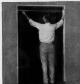
Kenna-pak steel header takes minimum headroom. Eliminates fascia and cutting of doors—standardizes all door opening heights.
