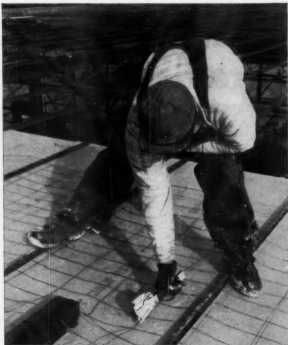
**STAPLING MESH** for poured gypsum roof—When a St. Louis, Mo., company started fastening wire mesh for poured gypsum roofs with staples, instead of plier-fastened hog rings, installation time was cut in half. Using the Bostitch H2B Hammer, this company finds that the wire mesh no longer pops up during the pouring and drying process.
