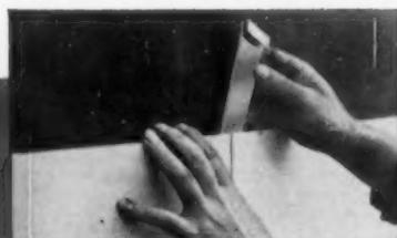
Joint fasteners link butt ends securely together...are concealed by next mounting strip.
