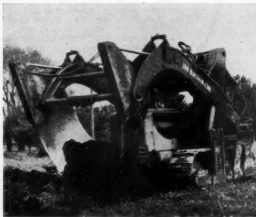
**BIGGEST BUCKET** is mounted on a bulldozer tractor. With it one man can move a tree up to 2 feet in diameter.
