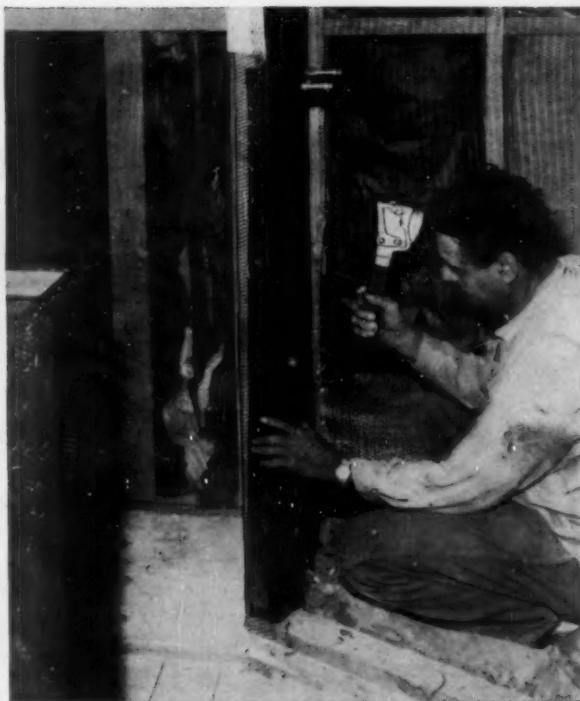
**STAPLING METAL LATH** in bathroom, this Dallas, Texas, tile contractor used to assign two men to install metal lath over sheet rock and studs in bathrooms. One man held the lath in position and held the nail while the other man hammered. With a Bostitch H2B Hammer, only one man is needed—and he does an even better job in one third the time.
