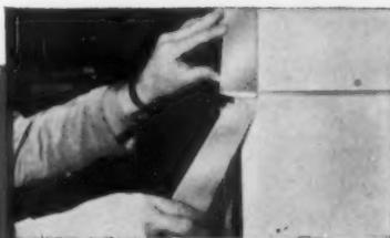
Interlocking corner caps, of bondersized and primed metal, slip easily into place without nails. Weatherproof!
