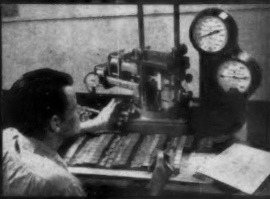
**8** **IN THE DFPA LABORATORY**, independent glue-line testing of samples backs up mill inspectors. Plywood samples tested must meet rigid
