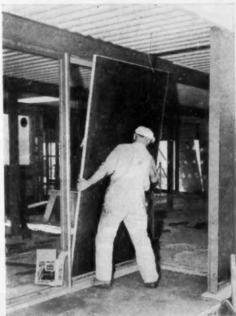
**ONE OF THE PLYWOOD PANELS** is set into place on the outside wall. The shape of the structural members provides the back stop. House was designed by A. Quincy Jones and Frederick E. Emmons.
