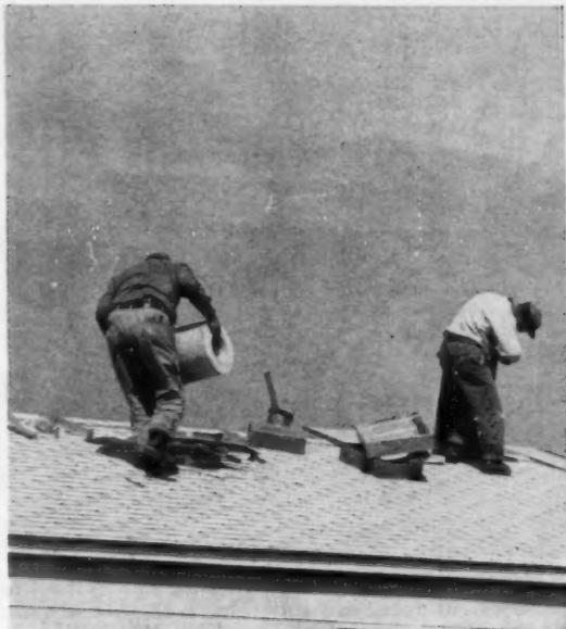
**PACKAGED PREFAB CHIMNEY** for the furnace is quickly installed by a two-man crew. Schmertz buys the packages, but subcontracts the actual installation of them. The cost, representing purely labor, is \$10 per house.
