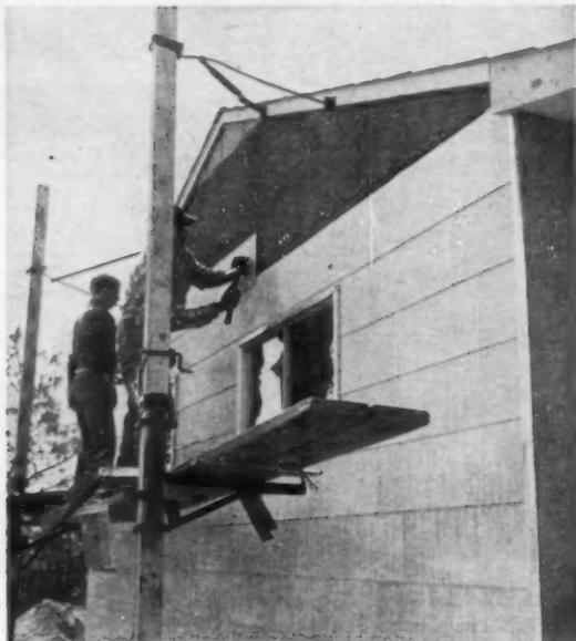
**PREFINISHED ASBESTOS SIDING** is put onto the shell, will require no additional painting. This work is subcontracted with the roofing for \$600 per house. Final paint bill, inside and out, comes to \$200 per house.
