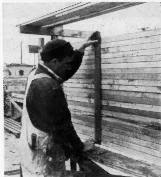
**POSITIONS OF INTERSECTING TIMBERS** are marked on more than 20 pieces at a time—in this case, plates—on this table. Master patterns are at top and bottom, and the straight edge is set on them to mark all at once.
