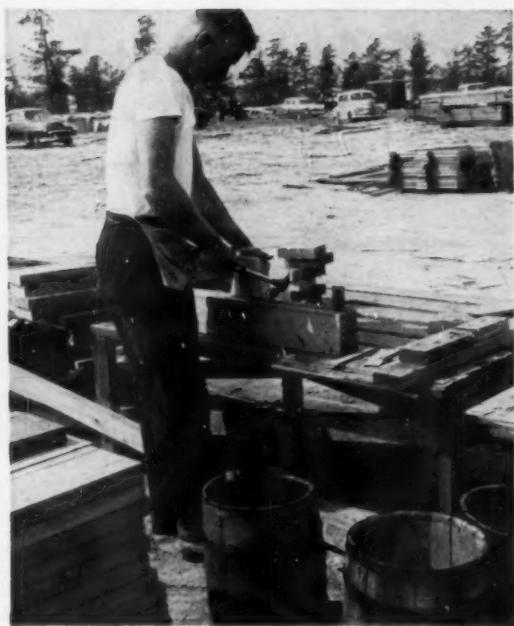
**DOOR HEADERS** are nailed together and blocks added to them on an assembly table. On a subsequent operation, the headers will be incorporated into a panel for the exterior, or a whole wall for the interior.
