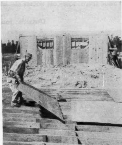
**PLYWOOD SHEETS** are spread out over floor joists so exterior walls can be assembled. This is not subflooring; when the walls are up, the plywood will be taken up and sent to the roof, where it will become the roof sheathing.
