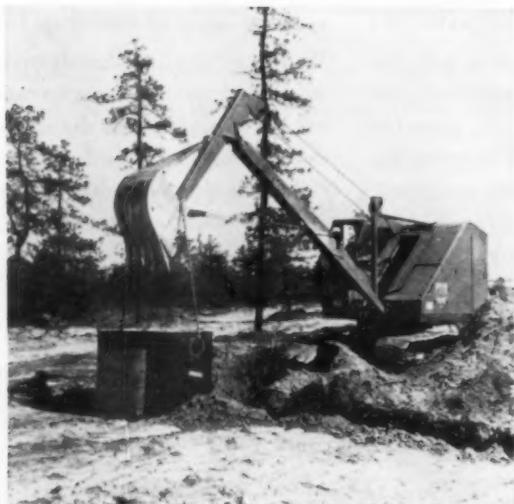
**METAL SEPTIC TANK** is dropped into place by the backhoe that dug the hole. Total cost of the septic system, including tank, digging, pipe, and 240 sq. ft. of drainage field, is approximately \$200.
