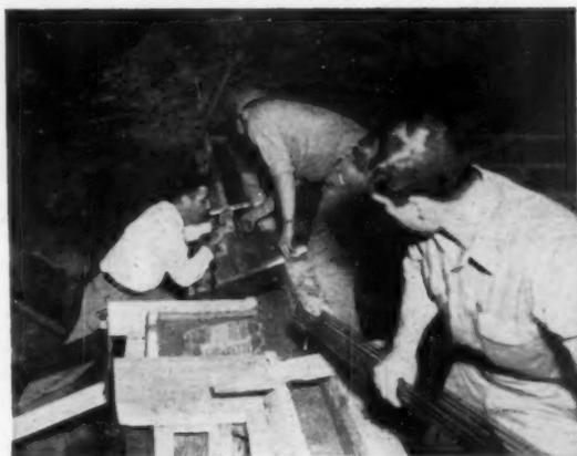
**PERFORATED SOLE PLATE** channel, with attached anchor bolts, is accurately embedded in top of the wet foundation.
