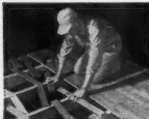
Typical time-consuming assembly job with odd lengths and shorts found in conventional flooring.
