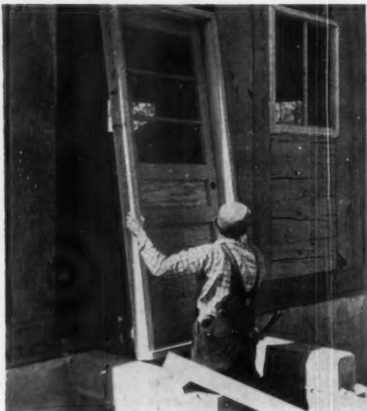
**PREHUNG EXTERIOR DOOR** is set into place. Schmertz does his own prehunging and millwork in two shops that are really just unfinished house shells. Two more of these shells serve as warehouses for finished millwork.
