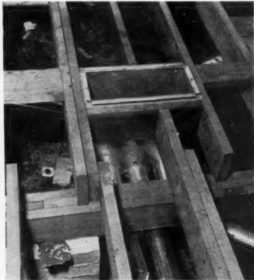
**HOT-AIR PLENUM** is set in place after the deck has been finished, usually after the shell is up. Installation is cheaper in crawl space than it would be in a concrete slab. Entire heating system cost is less than \$275.
