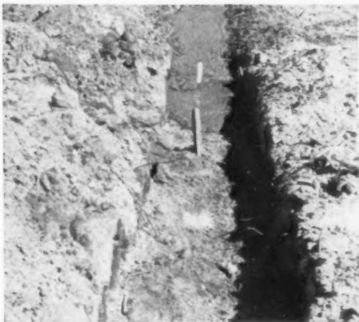
**GRADE STAKES** are driven at intervals into the bottom of the newly dug footing trench. They are set to proper height by a transit man, a job that is done in a fraction of the time needed to set regular footing forms level.
