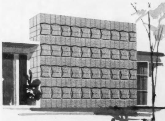
Shadowal block for the exterior of industrial buildings gives the effect of expensive special shapes at only slightly more than the 8" x 8" x 16" units.
