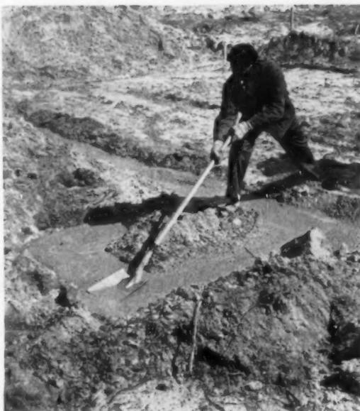
**AS CONCRETE IS POURED** into the footing trench, it is quickly smoothed and levelled to the top of the grade stakes by one man with a shovel. Stakes are left in the concrete. Footing here is for front doorstep.
