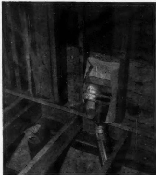
**HOT-AIR REGISTER** is fed by duct which leads up through a break in the sill, requires no break in the flooring. Insulation paper is put between it and the outside wall. Ducts also help heat the insulated crawl space.
