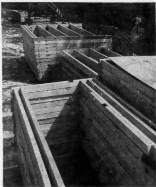
**FINISHED INTERIOR PANELS** are stored in the yard. At night and in bad weather, they are covered with polyethylene tarps. Fork lift will travel from pile to pile, pick up one of each panel, and carry the "package" to the job site.
