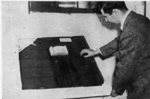
**ROOFING DISPLAY.** When buyer turns on water it pours down into gutter without penetrating layers of plywood, "felt," and asphalt shingles shown in peel-aways.
