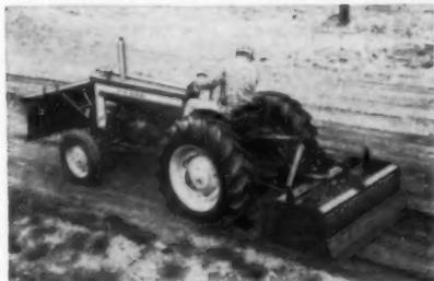
Left—John Deere "420" Utility Tractor and rear-mounted scarifier-scraper. This is one of many "pick up and go" tools that mount on the tractor's standard 3-point hitch.
