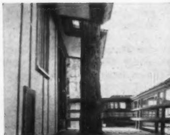
**THE OVERHANG** and balcony are framed around the trunk of the tree. On the hilly terrain, old telephone poles buttress slope beside the house.
