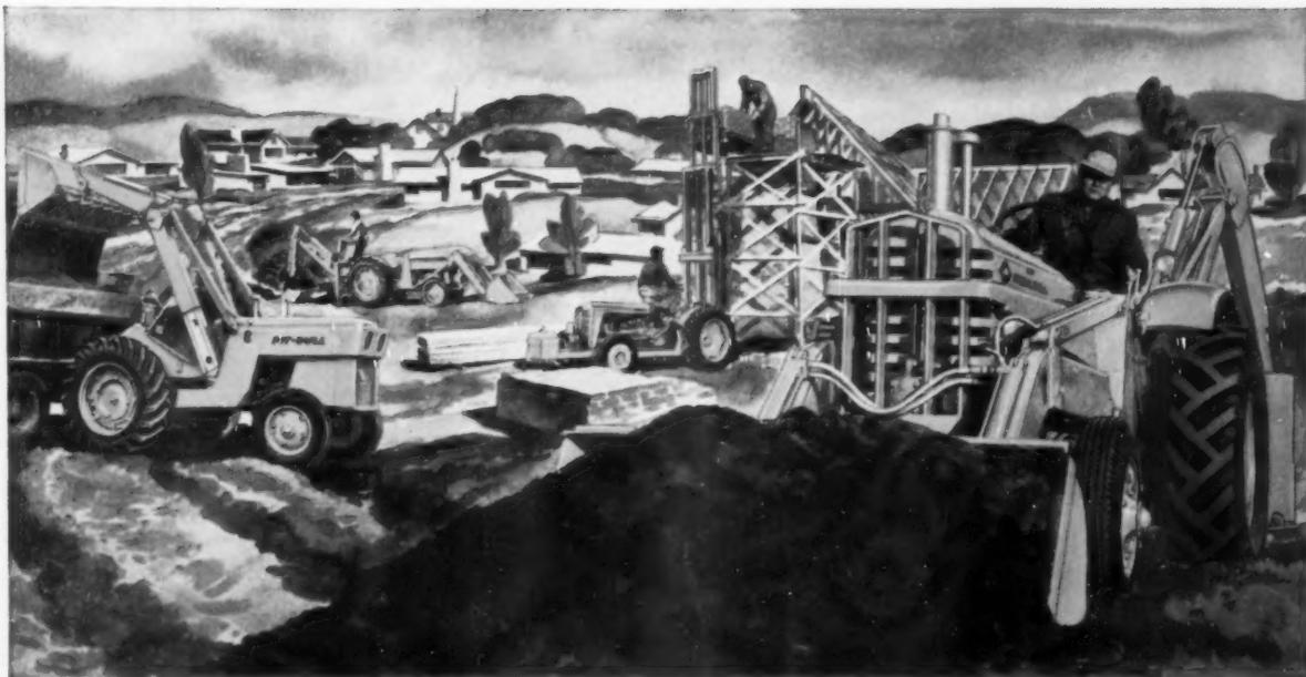
**TYPICAL WORK BULL PACKAGES:** Left foreground — 42-hp Davis Pit Bull with  $\frac{3}{4}$ -yd. loader. Left background — 34-hp Model 202 with 11 cu. ft. loader and rear-mounted backhoe that handles 12 to 36-in. buckets, digs to 12 $\frac{1}{2}$ -ft. depth. Center, Model 202 Fork Lift has standard 10-ft.
