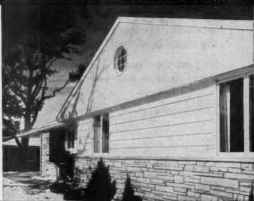
**New sidewall beauty** and fresh, attractive new design ideas come naturally with Insulite Primed Siding. Twelve-inch width of horizontal siding gives full 10 3/4" exposure—a de luxe effect. Vertical grooved panels (grooves 8" o.c.) and board-and-batten treatments with plain panels allow nice blendings and contrasts.
