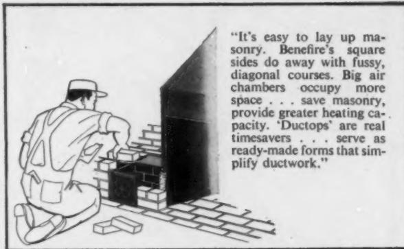
"It's easy to lay up masonry. Benefire's square sides do away with fussy, diagonal courses. Big air chambers occupy more space . . . save masonry, provide greater heating capacity. 'Ductops' are real timesavers . . . serve as ready-made forms that simplify ductwork."
