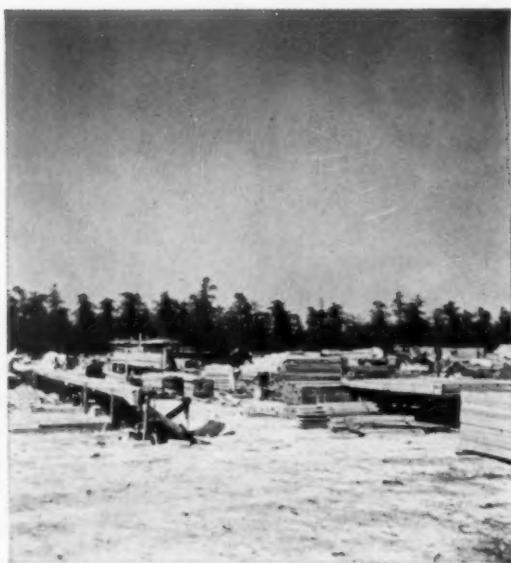
**PREBUILDING:** assembly-line methods and stockpiling of prebuilt and precut parts assures an even flow of materials to the job site. Quality control is easier when all precision work is done in one central location.
