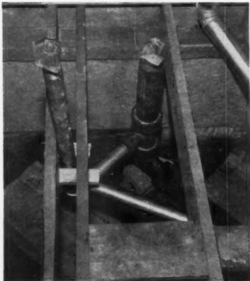
**ROUGH PLUMBING** is usually installed in the crawl space before the deck goes on, in a pinch can go in almost as easily afterwards. Schmertz pays plumbing sub less than \$475 per house for everything, including fixtures.
