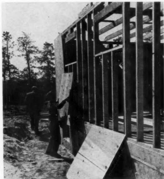
**SIDEWALL SHEATHING** goes up. Like all lumber on the job, it is precut to go in its particular spot. Precision planning like this is the big reason Schmertz can keep his carpentry labor bill for the whole house down to \$350.
