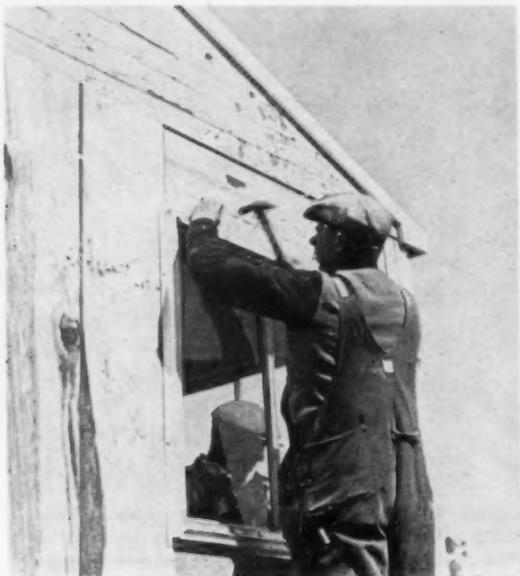
**ALUMINUM SLIDING WINDOWS** are nailed onto the facing of the window frame, require no fitting or shimming. They are made waterproof when the siding laps over the flanges and caulking compound is added to all joints.
