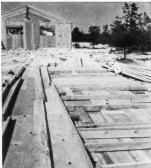
**EXTERIOR WALL** is laid out on the deck, ready to be nailed together and tilted up into position. Position of every stud and jackstud is marked on plates and sills; only the door and window panels are brought assembled to the site.
