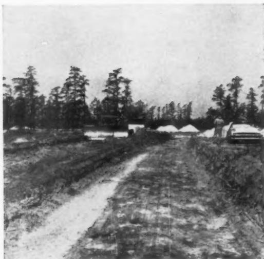
**ROADS ARE CUT** down into the ground, leaving building lots at a higher level for good drainage from the house. This is faster and cheaper than building up lots over the existing ground level. Road cost: \$200 per house.
