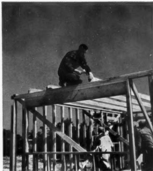
**CEILING JOISTS** are spiked down to the plate. Schmertz finds conventional roof cheaper than trusses; though a bearing wall is required in finished house, it isn't needed during construction so trusses wouldn't help.
