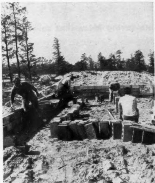
**FOUNDATION WALLS** for crawl space are the first step in building the shell. Considering the sandy soil and his method of installing floors, Schmertz says this is better than slab construction, the wood floors easier to sell.
