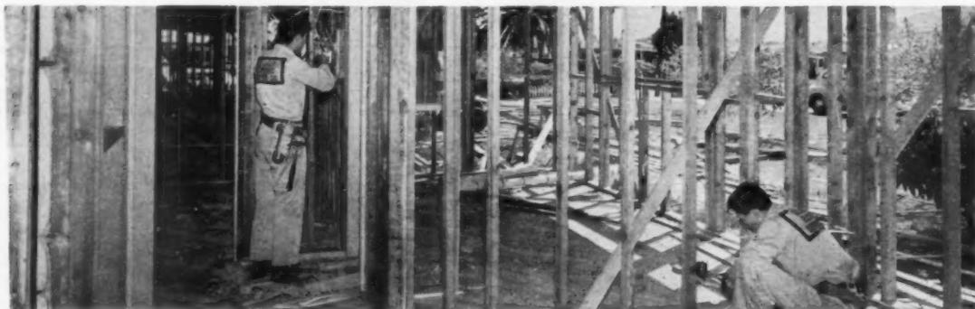
**IN THREE HOURS** these men can finish rough wiring. Work allows for two TV outlets.
