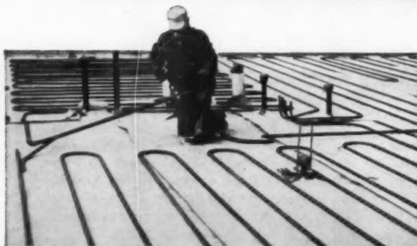
Welding joints of steel pipe on the job for Radiant panels.
