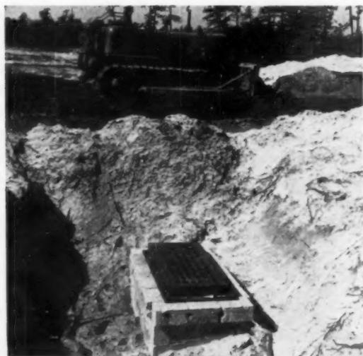
**STORM SEWERS** and their mains are easily and cheaply laid in the sandy soil. The only problem in this flat land is finding a low point to drain to. In this case, it's a stream across the highway. Cost per house, \$100.
