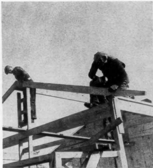
**ROOF RAFTERS** are nailed up. Crew puts up section of ridge with rafters at either end, fills in the rest of the rafters afterwards. This roof is for carport which used to be a \$325 extra, recently became standard.
