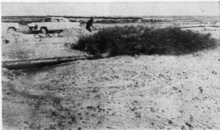
**WATER AND SAND** spray from the discharge pipe at a rate that provides 1,000 yards of fill a day. As the picture at left shows, water, draining to the lower level, carries the fill and levels it as it goes. Water also compacts the fill, making it unnecessary to tamp or roll for foundation.
