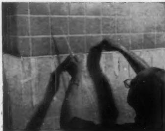
**2 GROUT STRIPS** outline each unit, keep place and whiteness permanently. Horizontal strips, 18" long, are positioned at bottom of rows.
