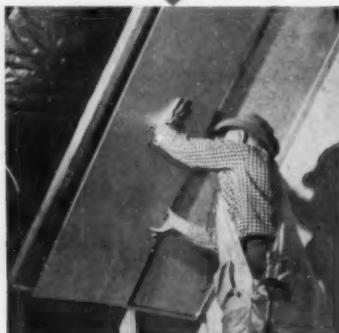
**BETWEEN RAFTERS** went blanket wool insulation, then 1/4" plywood panels. Ceiling was braced by 2x4s with plastic panels to conceal lighting.
