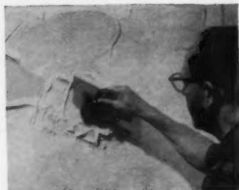
**1 PLASTIC TILE** goes on more easily, with new plastic grout strip. After applying adhesive with trowel, tiles are snapped into position.
