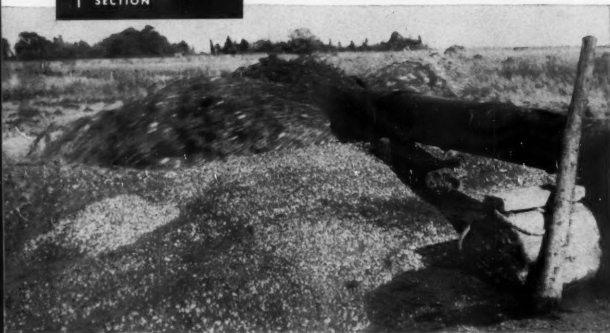
A THOUSAND YARDS A DAY of fill can be dug, moved and pumped in this dredging operation.
