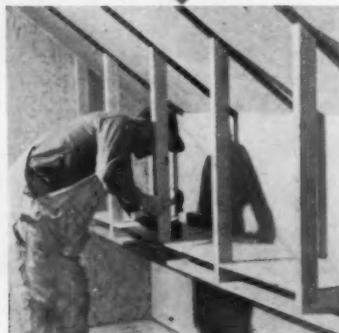
**BASE SURFACES** were covered with plywood; then framing for storage bank under eaves went in, leaving space underneath for roll-out day beds.
