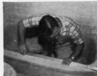
**1 TUB ENCLOSURE** to up-date the bathroom. Job begins with cutting of sill section, and installation after application of adhesive.
