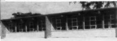
The Vento Champion Steel Basement Window is the best window made and for these reasons: 14 gauge formed steel sections; 3 position ventilation; positive action cam lock gives greater tolerance;
