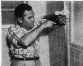
**2 JAMBS ARE SECURED** to tile walls with long flat-head wood screws after drilling is completed and rawl plugs have been inserted.
