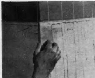
**3 NEXT ROW OF TILE** goes on faster. Strip is same depth as bevelled shoulder of a plastic tile. Artcrest Plastics (No. Y6, p. 128).
