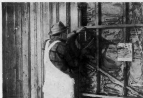
**WOOD BLOCK** is used intelligently here to force groove of lodge pole panelling over tongue of previously-set panel. Such care follows Western Pine Assn. specs. Note aluminum-faced fiber glass insulation.
