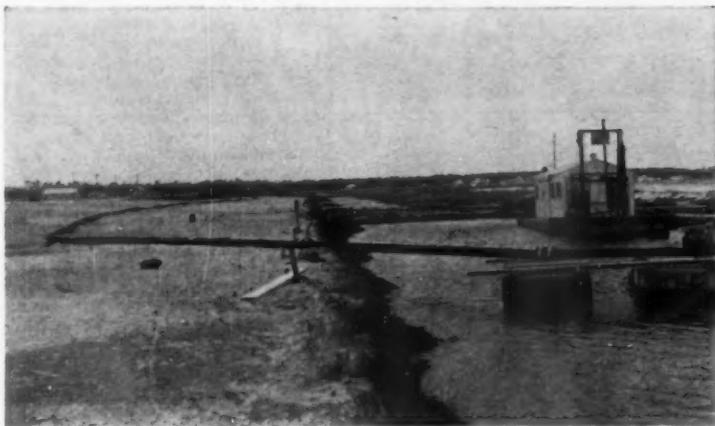
**PIPE LENGTHS** are carried ashore on drum rafts, as shown here. The connections between the sections are flexible enough to allow the dredge to move from side to side of the lagoon without having to uncouple. The pipe will also pass fairly large stones without clogging up.
