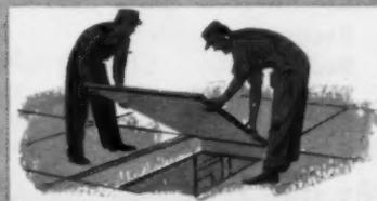
**CEMESTO® STRUCTURAL INSULATING PANELS.** Attractive gray cement-asbestos facings, bonded to fiber board core. Structural roof deck and finished ceiling in one panel; exterior walls and interior partitions. Maintenance-free.
