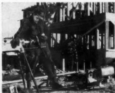
**Carryable Gasoline Engine-Driven Generators . . .** Lightweight Homelite generators can be carried and used anywhere to provide high-cycle and 115 volt power for your electric vibrators, tools and floodlights. Complete range of sizes up to 5,000 watts . . . all standard voltages.
