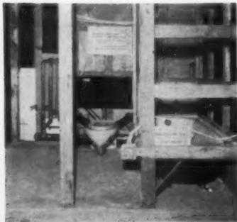
**WALL-HUNG CLOSET**, raised-bottom bathtub eliminate pipes from floor slab. Borg-Warner created new fixtures to cut labor costs.
