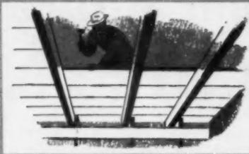
**INSULATING ROOF SLABS.** Roof deck, insulation, built-in vapor barrier, finished ceiling, plus continuous vapor seal at all joints. (Also available without vapor seal.) Ideal for exposed-beam construction.
