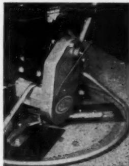
Within one-sixth of a second, the unique manual clutch shown above stops the trowel blades, leaves the engine running. This makes the machine safer to work with, and much easier to start since full throttle can be used if necessary.
