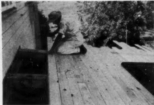
**TONGUE-AND-GROOVE** decking goes down next. Underside provides finished ceiling. After deck is completed, overhang is cut with power saw. Deck's thickness is intrinsic insulation—a "hidden value."
