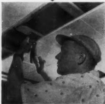
**CEILING TILE** went up next with help of Insulite clips. Clips were inserted along edge of each tile, then nailed directly to the furring strip.
