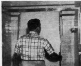
**3 DOORS LIFTED** together as unit and placed with head lowered onto top of jambs and filler strips. From Ludman Corp. (No. Y7, page 128).
