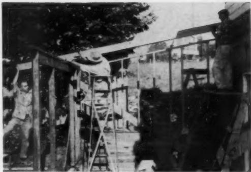
**ONE OF FOUR 6'x6'** roof beams gets toe-nailed to header, here. After securing beam, carpenter will jam beveled strip between beam and header. Note strip of quarter-round at beam and deck seam in photo—left.
