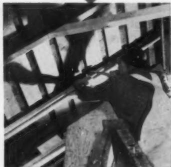
**FIR PLYWOOD** panels, based on 1x3" nailers alongside each rafter, were fitted inside to allow 1/2" exposure of original ceiling rafters.
