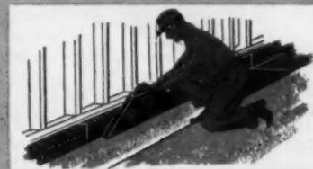
**FLEXCELL® PERIMETER INSULATION.** Asphalt impregnated throughout entire thickness of the board. For concrete slabs at grade. Like all Celotex Fiber Board products, effectively protected against dry rot and termites by exclusive Ferox® process.
