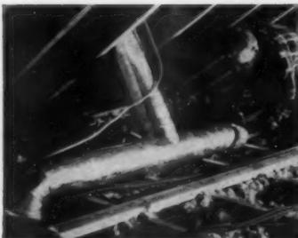
**2 DUCT GOES** into attic. Seven-inch spur goes to range hood; shorter duct to intake grille in bath. Same ventilator will serve both rooms.
