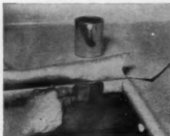
**2 AFTER CUTTING** the surfacing, adhesive is applied and covering is fitted on. Rounded moldings need contact bond adhesive.
