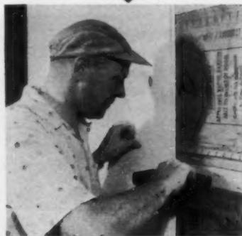
**WALL FINISH** of Duro-lite Plank was easy to apply because of its t&g nailing flange. Plank was stapled through flange to furring strip.
