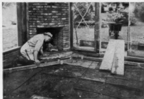
**CONCRETE MAN** checks level for slab. Vapor-proof building paper goes down first, followed by reinforcing metal rods (both "hidden values"). Slab will be topped with asphalt tile to run flush with hearth brick.
