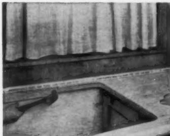
**1 PLASTIC SURFACING** for countertop begins with metal binding and fillet strips where needed, wood molding nailed to front of surface.
