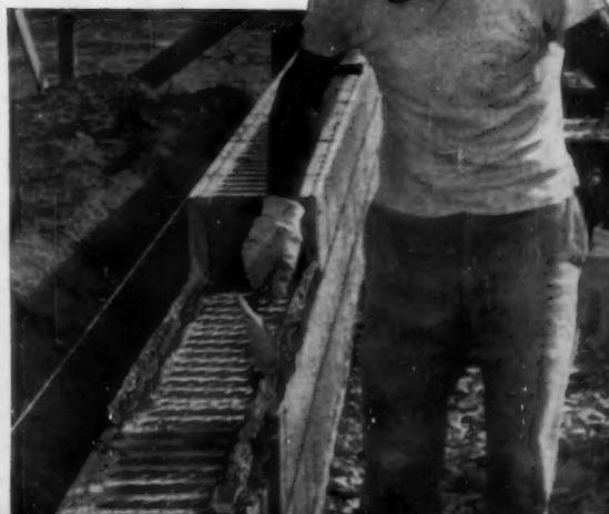
Mr. Ehman finds that mortar flows in, under and around Key-Wall to give exceptional bonding and provide full mortar embedment. Key-Wall is galvanized for protection against weather, assuring a strong bond. It is easy to store on the job. 200-ft. rolls are compact, and can be carried with ease.
