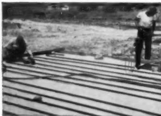
Typical installation of steel pipe radiant heating coils on slab.
