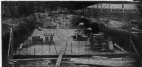
Vertical pre-stressing steel rods are ready for specially grooved pre-cast wall sections to be placed over them. No heavy construction equipment needed. All work can be done with common labor.
