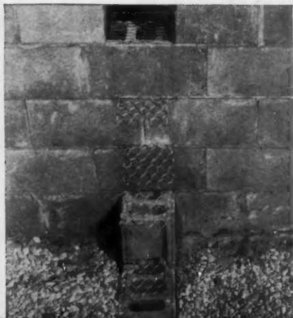
Another reason Mr. Hand rates Key-Wall the best is because it is so easy to tie in curtain walls. On this job, an 8" block was tied into the outer wall, with Key-Wall being used as reinforcement at every joint. Short lengths are used for convenience.
