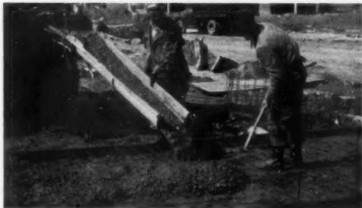
**HIDDEN VALUE** added to every house at Aurora Gardens is steel-wire reinforced driveway. Sidewalk is put in with similar reinforcement—gives sidewalk longer life.
