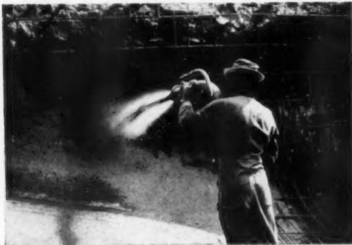
**GUNITE** is pneumatically applied concrete. The process forms a material of great density. This job, requires the know-how and tools of a specialist.
