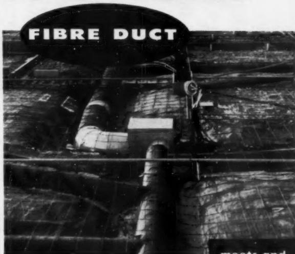
The perimeter heating-cooling system for this \$30,000 residence included a GE Weathertron heat pump and economical Sonoco SONOAIRDUCT fibre duct. Lightweight, long-length SONOAIRDUCT was easy to handle and level, thus saving time, labor and money in installation. By mitering the duct, all T-joints were made WITHOUT metal fittings.
