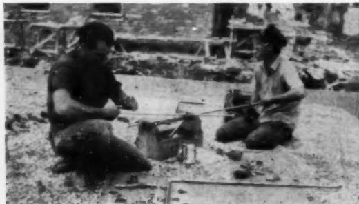
**HIDDEN VALUE** is this copper tubing which plumbers are preassembling here before frame goes up—a step which cuts time and labor costs from the overall expense.
