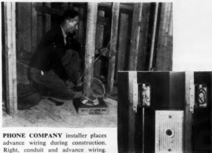
**PHONE COMPANY** installer places advance wiring during construction. Right, conduit and advance wiring.
