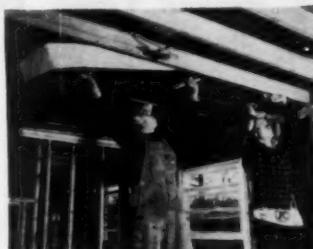
**SIX-INCH THICK** insulation of spun mineral wool batt suggested as "hidden value," particularly for builders of air-conditioned homes. From Baldwin-Hill Co. (No. Z21, p. 114).
