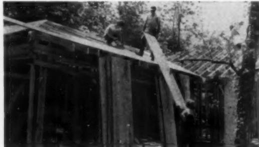
**HIDDEN VALUES** as well are edge-laminated sheets of southern pine lumber used to provide a tight roof economically without sacrificing quality construction methods.
