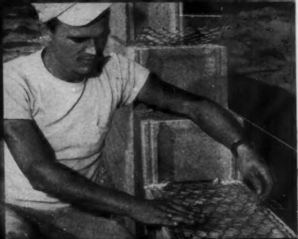
Brickmason Ted Ehman, working on the Russellville Indiana High School, likes the way Key-Wall can be iapped without interfering with embedment or adding thickness to the joint. This is particularly important at corners. With Key-Wall, masons find it just as easy to reinforce corners as on straight runs.
