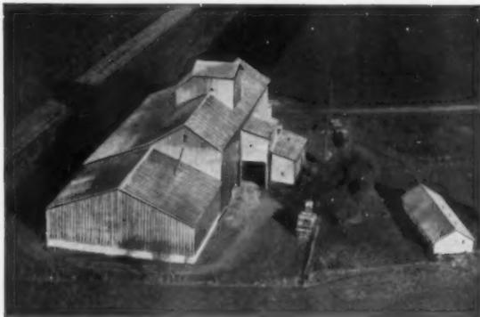
**FIRE PROTECTION** was the number one reason this Oregon grain storage mill was built with steel. The owner lost his first mill to fire, so vowing it would never happen again, he specified USS Corrugated Roofing and Siding Sheets and USS Floor Plate for his new building. This also lowered his insurance costs.
