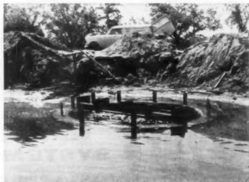
**DRAIN AT END OF LAKE SHERWOOD** serves as overflow to maintain a constant water level, also allows the whole lake to be drained dry for future cleaning.
