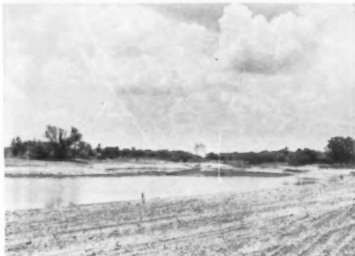
**FINAL GRADING** has been done on the bottom here, and lake is beginning to fill. Areas close to shore drop off sharply to prevent weed growth, but vegetation is left in
