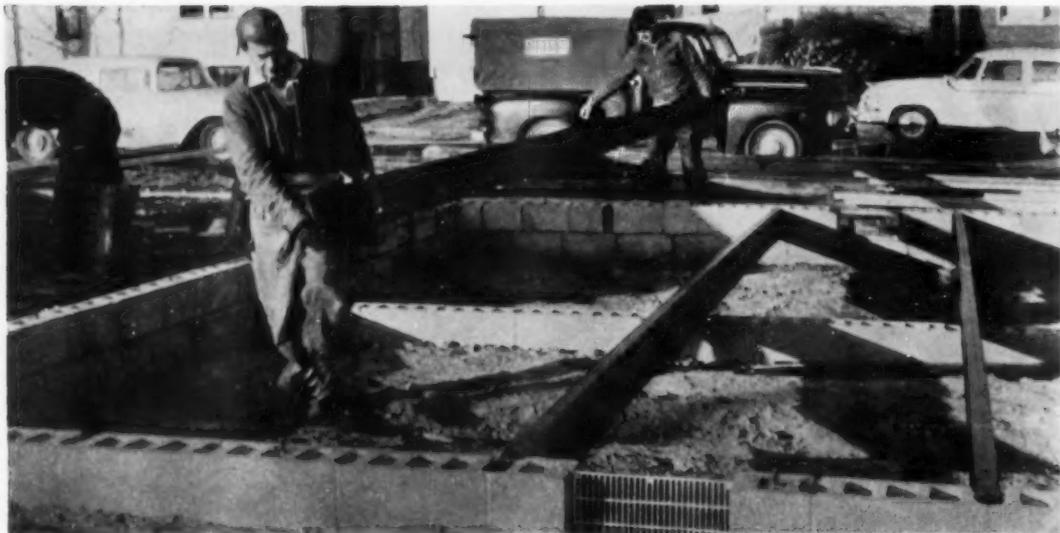
**STEEL IN FOUNDATION** used in flooring system with 2.4.1 Plywood Panels. Time-saving method allows five
