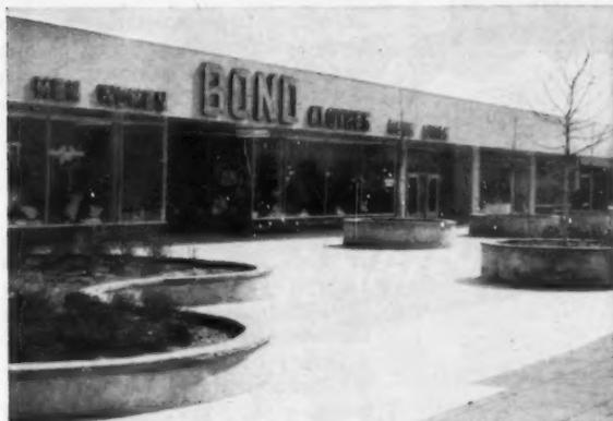
Forty thousand sq. ft. of Weldwood Porc-Lin-Ply were used for fascia of soffits in this shopping center in Valley Stream, N. Y.  $\frac{1}{16}$ " thick panels weigh only 1.75 lbs./sq. ft. Hard, semi-matte finish panels in 9 colors are easily wiped clean.
