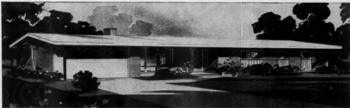
FINISHED HOME, all brick veneer and fully insulated, will cost about the same as an identical house with conventional frame construction. The use of Styrofoam (Dow expanded polystyrene)
