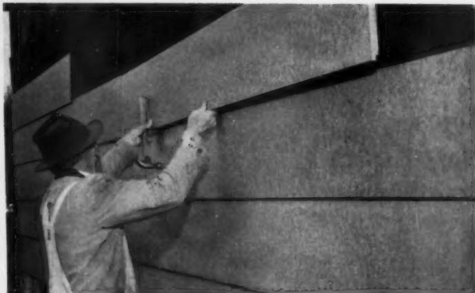
**SELF-ALIGNING**, the siding is easily applied by one man. Rabbeted joints eliminate the necessity of carefully lining up each piece.
