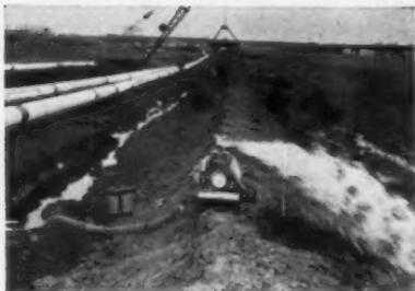
**Self-Priming Centrifugal Pumps . . .** Carry these lightweight, dependable pumps anywhere. Non-clogging design . . . 28 foot suction lift . . . capacities up to 15,000 g.p.h. . . sizes from 1½" to 3". Diaphragm pump also available.
