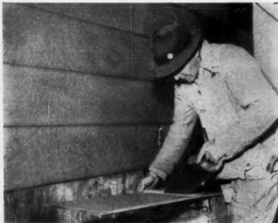
**EITHER HAND OR POWER TOOLS** can be used. Cross-ply veneer face prevents splits in nailing—boards stay firmly in place.
