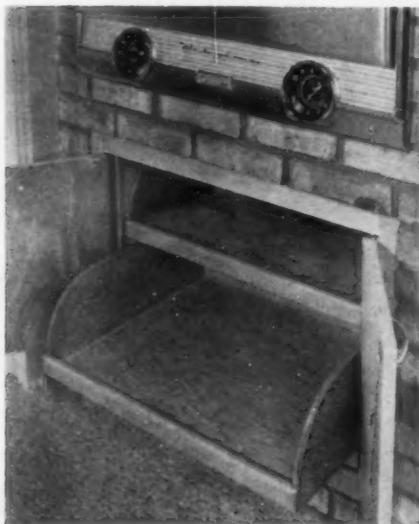
**PULL-OUT SHELVES** under oven are similar to those under range. Half-inch plywood side piece for pull-out shelves, not shown, is 21" deep by  $16\frac{3}{4}$ " tall with a slide 8" from top.
