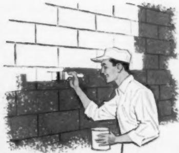
Brick, concrete block or poured concrete walls take on a smoothness and beauty when finished with aluminum paint. It bonds tightly, seals pores, reflects light and heat.
