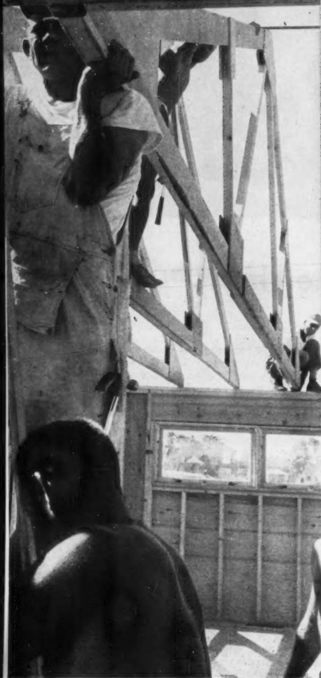
**INTERIOR PARTITIONS** start with shoe nailed to slab on chalk lines. Cut at same time are a second shoe, of one inch stock, and top plate. Heavy paper is used to protect the finished floor.
