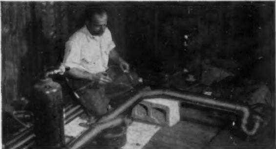
The light weight of copper tube makes it possible to pre-assemble sections. Units like this, or even larger, can be handled and set in place easily.
