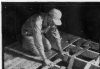
Odd lengths and shorts make assembly of conventional flooring a time-consuming job.
