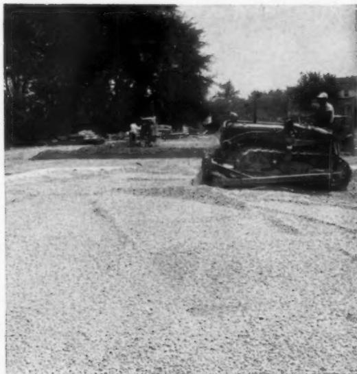
**PERIMETER DUCTS ARE IN PLACE**, and slag is spread by bulldozer. Trenches for feeder ducts will be hand dug. When bulldozer finishes, blocks between garage and house slabs will be set, ductwork carried on across.
