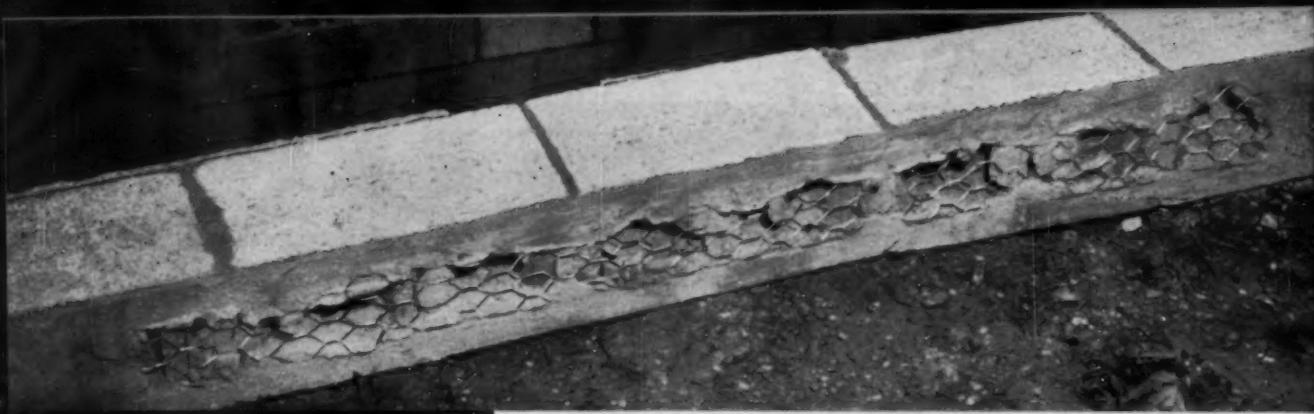
Note the full embedment of the face shell of these units. KEYWALL helps hold mortar in place, giving a stronger, more weather-tight wall.
