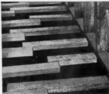
**5** Leave a minimum gap of 1" between ends of screeds and baseplate around edges of room to allow for normal expansion of the finish flooring.
