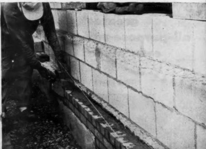
"You can't beat KEYWALL as a wall tie," according to Mr. Gans. "It does everything a wall tie should do, and does it better. In addition, it gives reinforcement. What's more, this double-duty product costs no more in the wall than the ordinary non-reinforcing type of wall tie. With KEYWALL I omit header courses, too. KEYWALL doesn't shear when walls move, as header brick do. It's easy to see why I'm so enthusiastic about KEYWALL."
