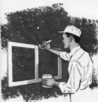
Paint all metal components with Aluminum Metal and Masonry Paint for longer life and better finish coats.
