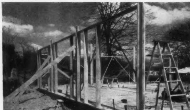
Wall framing sections and panel components were assembled by National Homes in its Lafayette factory. Rabbedted 2x6" frame is made to receive flanged panel (see photo below). Termite shield of extruded aluminum (drawing below), serves also as drip cap, slab stop. Pre-assembled posts are used at corners.
