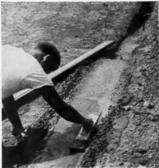
**FOOTINGS ARE POURED** directly into trench, leveled to top of stakes. Machine digging makes a highly accurate 8-inch trench, saves concrete. Accurate leveling will speed up blockwork, produce a better slab.
