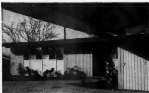
**"Board and Batten"** siding is easily achieved by applying Exterior fir plywood vertically and covering with moldings.
