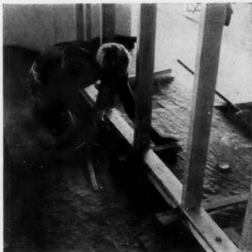
**SHIMS ARE DRIVEN BETWEEN** top and bottom shoe to set wall tight to ceiling before nailing; shims are then trimmed. Three men can set partitions in a day, and the remaining drywall is hung and taped in same time.
