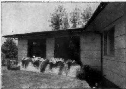
**Wide-lapped** siding made by ripping panels in half or thirds has unusual "scale." Use standard PlyShield grade or, for smoother, more durable paint finishes, overlaid plywood.
