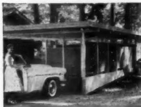
Use Exterior fir plywood for single wall carport construction. Panels add bracing strength.
