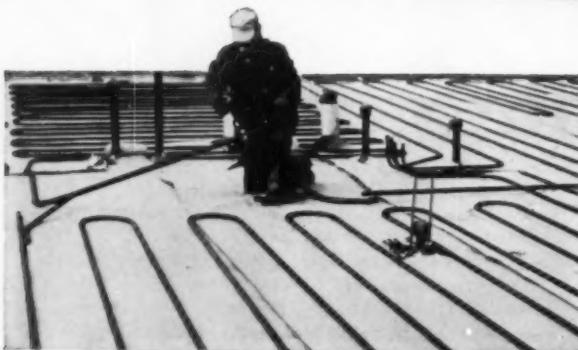
Welding joints of steel pipe on the job for Radiant panels.
