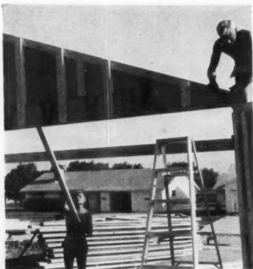
**FIRST TRUSS IN GARAGE "L"** has joist hangers to carry the ends of the main trusses across width of garage. The whole "L" will be framed and sheathed for stiffness before the main trusses are set in place.
