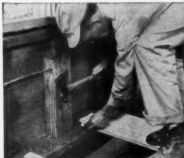
**7** Wide baseplate along two walls is recommended to provide a good nailing surface for flooring ends, increasing rigidity of the installation.
