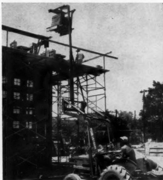
**UTILITY BOOM** is attached to front-end loader frame, can lift material up to 20 feet, high enough for two-story houses. One accessory is a one-third yard concrete bucket. Made by the Henry Manufacturing Co.
