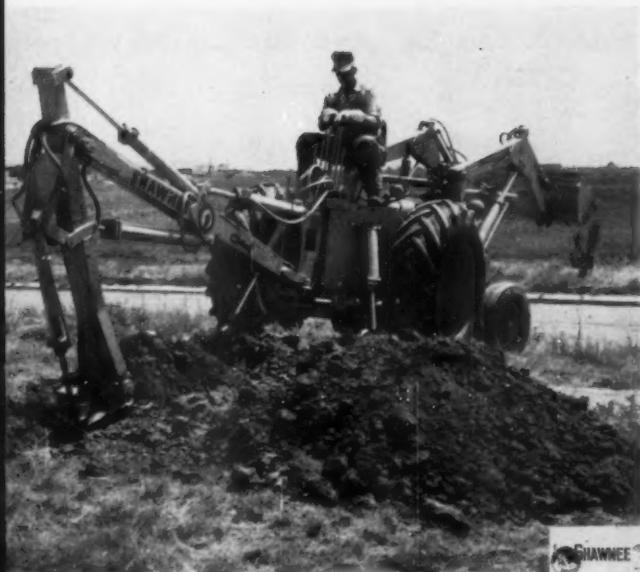
**MOST IMPORTANT ATTACHMENT** for most builders is the backhoe. Average unit can dig about 12 feet deep, has buckets from 12" to 24" wide, can dig anything from a sewer-line trench to a full cellar excavation.
