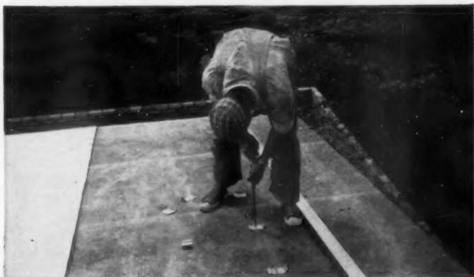
Despite newness of this work to the roofers, they installed entire roof in slightly less than two days. Here, mechanic affixes aluminum clips 18" o.c. to sheathing which is covered with roofing felt, necessary only as emergency wet-weather protection. Clips will receive batten extrusion, below.
