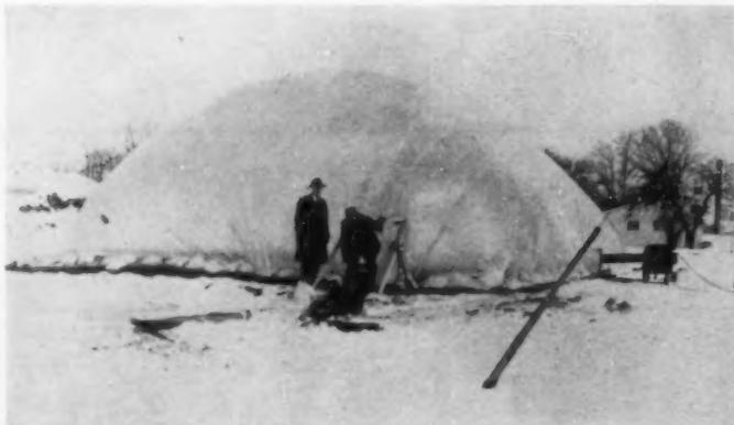
**P**olyethylene sheet is one of the most versatile materials a builder can use in winter or summer. Here, looking like a gigantic balloon, is a warehouse made out of the material. Sandbags around the edges keep it from taking off, and an old oil burner blower provides enough pressure to keep it ballooned up. At night the blower can be turned off; during the day it allows a man to walk around inside and move material.
