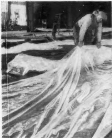
You can reduce surface shrinkage of concrete to a minimum if you use Durethene polyethylene film as a "blanket" both over and under the concrete you pour. Too, Durethene film keeps in the moisture required for a low even cure so that the set concrete is up to 60 per cent harder, stronger and more durable. What's more, Durethene film is waterproof and readily protects slabs from sudden showers.
