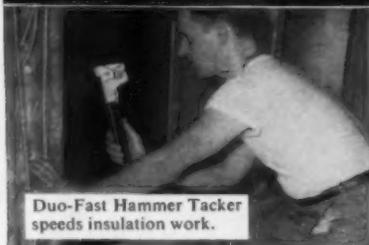
Duo-Fast Hammer Tacker speeds insulation work.
