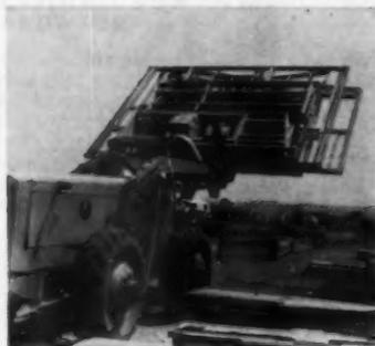
**IDEA . . .** Assembly line construction. Your houses can be broken down into component parts, lined up for on-the-field assembly, using tilt-up construction. A Hough Payloader readies materials. (No. Z13, p. 114.)
