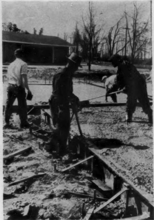
“We find an electric vibrator saves time by floating out the water more quickly. Also it compacts better. We can use a stiffer mixture, which is stronger, and less cement, which is cheaper.”
