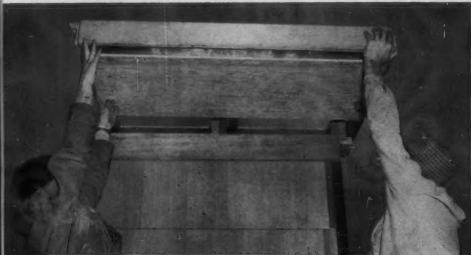
TWO MEN position component. Plywood soffit rests on frieze board.
