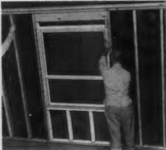
**IDEA . . .** Faster framing, done with the help of a Structural Windowwall from Andersen. Whole window component is joined to adjacent framing, then tilted up with wall. (Circle No. Z1, p. 114.)
