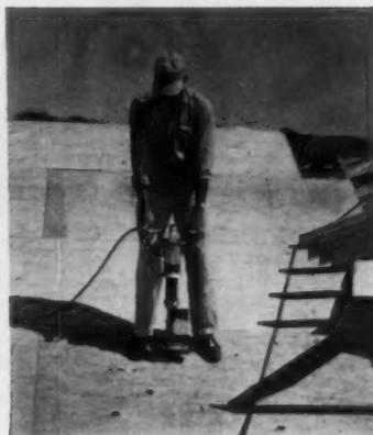
**IDEA . . .** Three nails a second is the record for this electric nailer. Speeds, by three to five times, nailing of subflooring, roof sheathing, trusses. This one, from B & H Homes. (No. Z11, p. 114.)
