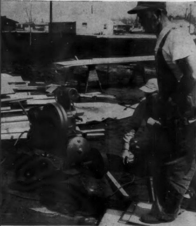
“This is the compressor end of our compressor-pneumatic stapler rig. The stapler drives a divergent point staple up to about 1½” long, and it has tremendous holding power.”
