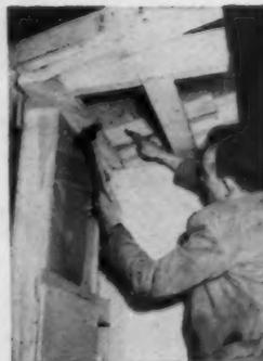
OUTLOOKER (2x4) is nailed to upper chord of truss. Before nailing, the component supports itself by leverage of outlooker against roof sheathing.
