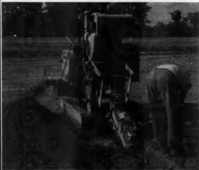
““We use this trencher mostly for digging foundations. Two men can do a 2,000 sq. ft. house in an hour and a half. The trenches are exactly 8" wide, so we don't waste concrete.””
