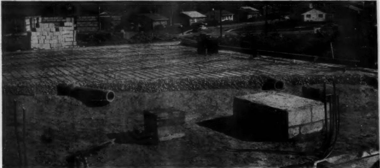
CROSS-SECTIONAL photo of slab shows backfill, layer of gravel, vapor barrier and steel mesh. Blocks at right are the top of one of the piers. Clay pipe sections are heating ducts.
