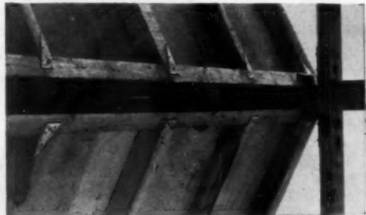
**HALF-INCH** bolts drew up pairs of panels forming valleys. ⅝" Fir Plywood, 5'6"x4', was nailed to frame of 3x4's, alternating with 2x4's on 2' centers.
