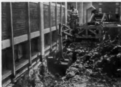
**EXCLUSIVE FLUSH-DIGGING!** Entire mast and boom assembly shifts from center to either side for flush digging alongside buildings, fences, by trees, and other obstructions. Only Davis offers this advanced feature!
