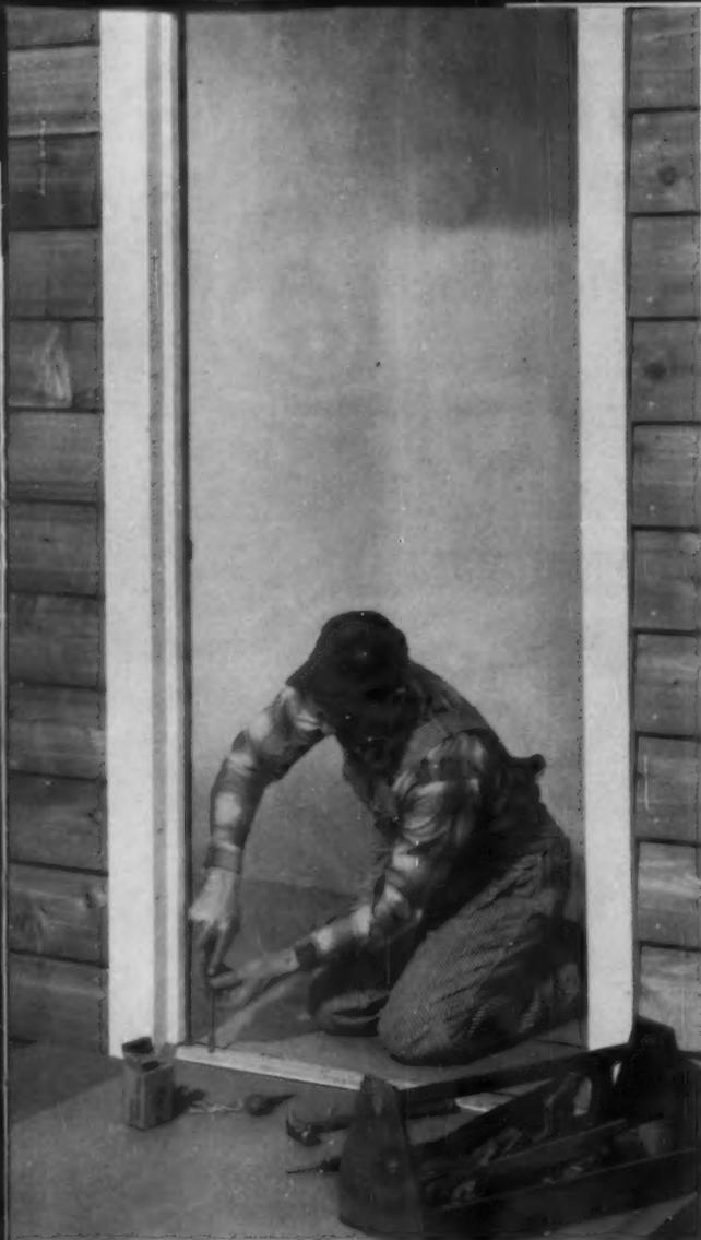
**Easy-to-use** corrosion-resistant nails of Alcoa Aluminum reduce labor costs by eliminating time-consuming countersinking and puttying. They drive easily—are etched to hold tightly.
