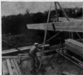
**IDEA . . .** One man can make use of mechanization with a wall jack like this one from Proctor. Rigged as gin pole, it lifts huge beams; holds them in place. Only one man needed for job. (Circle No. Z12, p. 114.)
