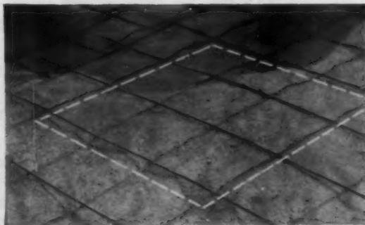
**DOTTED LINE** indicates pier position. Mesh must be lifted an inch off barrier as the concrete is poured.
