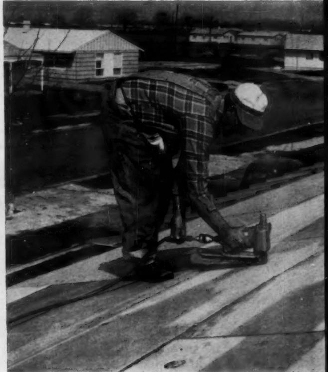
“One man with a stapling gun can keep up with two men laying and tacking down roof sheathing. We can do the whole roof in four hours. The only problem is loading the gun fast enough.”
