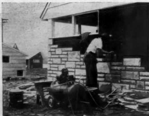
**ON A JOB** as big as Levitt's, even the simplest operations are mechanized. This stone facing is an optional item, yet the applicator has a special pneumatic hammer rig for it.
