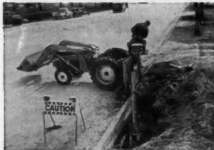
**YOU ALWAYS FACE YOUR WORK!** Seat and control assembly is mounted on a mast assembly... swing to face the job regardless of operating angle. You work fast because bucket is visible, controls at your fingertips.
