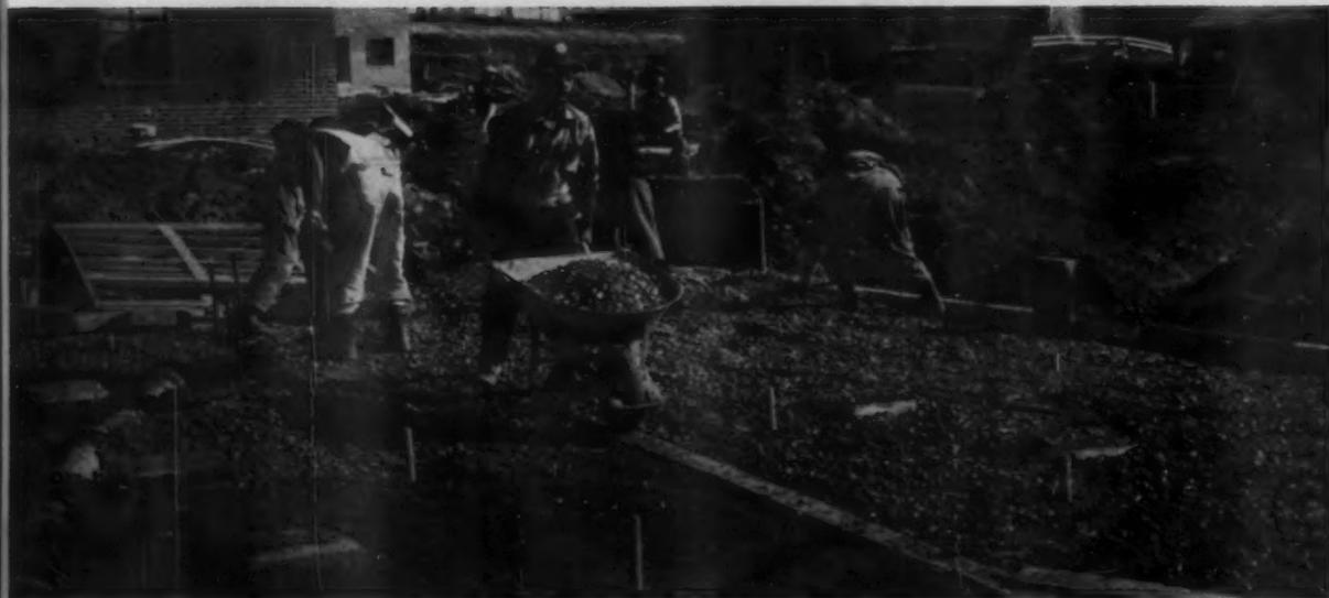
**SIX-INCH LAYER** of washed gravel is spread over the uncompacted backfill in this foundation. Note hilly site, the reason why so much cutting and filling are necessary in this area.
