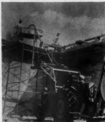
**IDEA . . .** How to mechanize your materials handling. Add a special boom attachment to a front-end loader. It hoists material to 2nd and 3rd story. Attachment is from Sherman. (No. Z8, p. 114).
