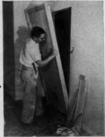
**IDEA . . .** in the near future perhaps you'll mechanize with a brick panel. SCPI has a panel out, one brick in width, that's designed to be a 2½" thick bearing wall with stacked joints. Speeds up, simplifies construction. See Feb. '58 American Builder, p. 206, or (No. Z3, p. 114)
