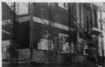
**IDEA . . .** Mechanize your brick laying. SCR Process includes self-elevating scaffold, new guide-line system. (No. Z9, p. 114.)
