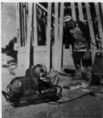
**IDEA . . .** On-site power tools are the first and most important step in mechanizing. If power isn't available, a generator is a must. Above, Homelite's. (No. Z7, p. 114.)
