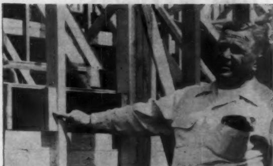
**"YOU CAN SAVE \$60 per house balloon framing your splits,"** says Harry Lubell. "We've tried it both ways. Balloon framing is better all-around construction. Once partitions with ledger boards are in place: unskilled labor does the rest."
