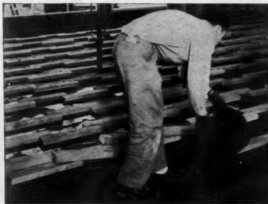
**1** Apply surface moisture barrier to slab and lay flat, dry, preservative-treated 2 x 4 wood screeds in hot mastic. Use random length screeds, 18" to 30".
