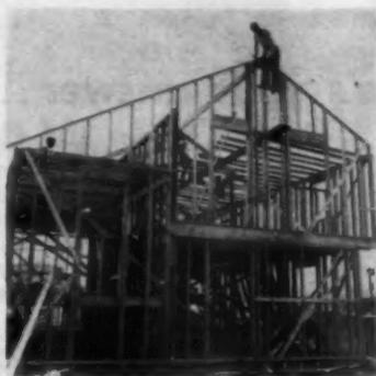
**BECAUSE** of 2nd floor projection, front half of house is framed conventionally. 2x12's are used at openings.
