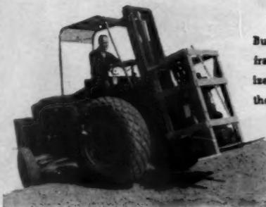
Built with a new sub-frame design for equalized weight distribution, the large tractor tires give more ground clearance and traction, and greater cushioned mobility regardless of ground conditions.
