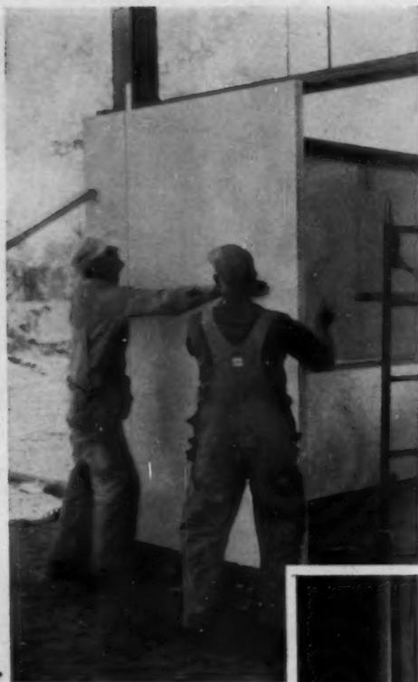
**LIGHTWEIGHT** plastic panels were easily erected and dismantled by A.F. of L. carpenters. The fastening details are given below.
