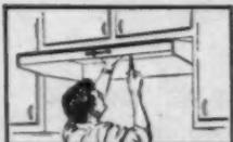
Fasten hood to cabinet. Use standard 9" round duct or a Fasco damper reducer Model 886 with 8" round duct.
