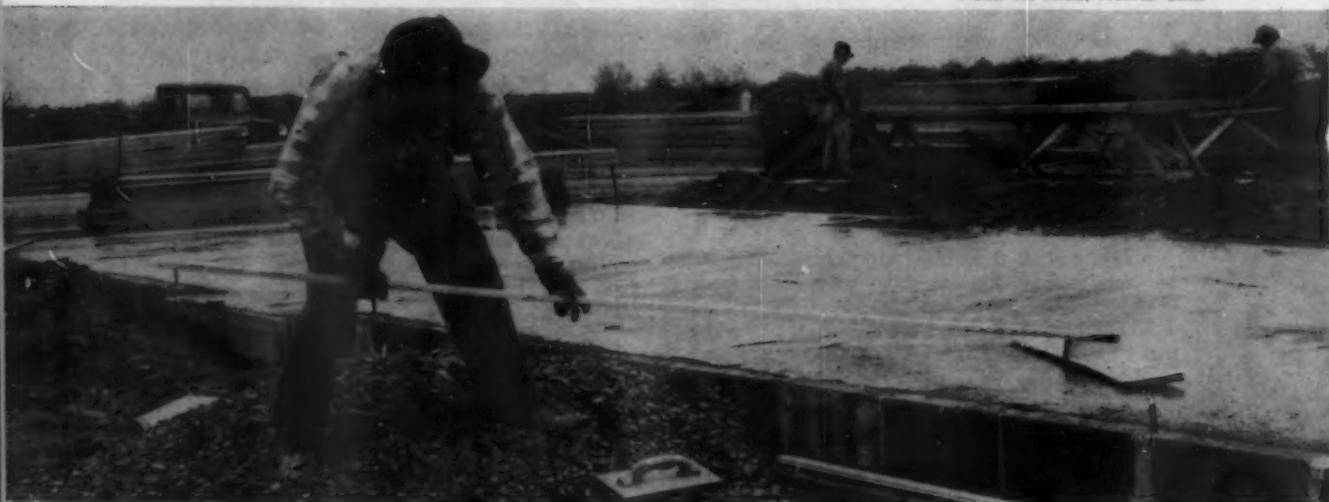
**POURING** center bearing footing and slab monolithically saves four courses of block.
