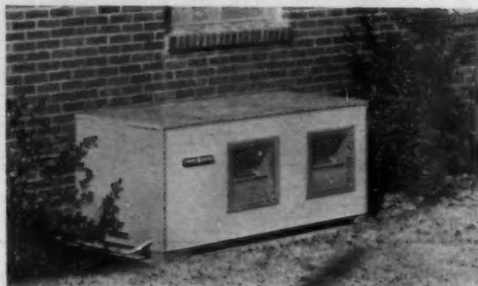
**SPACE-SAVER DESIGN . . .** in a new gas furnace from General Electric. Unit (left) has a front line flue for simple closet installation. Close clearances allow space saving. Small cooling coil attaches to top for air-conditioning. Right, outdoor compressor-condenser section. (No. S1, p. 150.)
