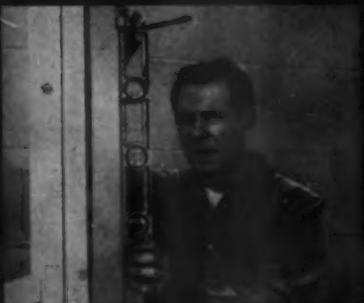
**2. SET FRAME IN PLACE.** Set frame in opening; plumb. Bend over stud anchors.
