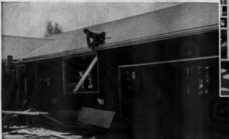
**HANG REPUBLIC HOUSE-LONG "K" GUTTERS** and cut installation time in half. New Republic 26 and 28 gage Galvanized Steel Gutters now are made as long as 32 feet. Hang them in one piece. Cut installation time. Ideal for long-roofed contemporaries. No need to measure, cut, and solder as with "old style" short gutters. No seams to detract from appearance, or to become potential points of failure. Sold through Republic Sheet Metal Distributors. Send for data.
