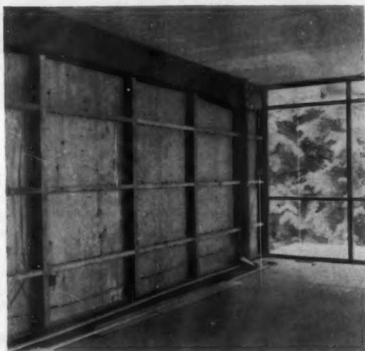
CONVENTIONAL studs weren't used for the wall. Instead 3x4 verticals, 4' o.c., and 2x4 horizontal blocks, 2' o.c., were specified. Fir plywood sheathing was glued to verticals and blocks. The floor is ready for vinyl finish.
