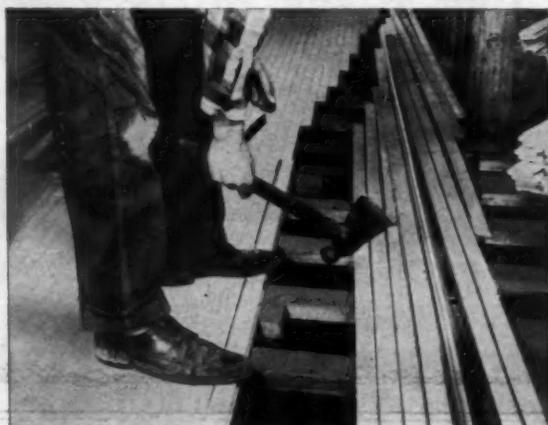
**3** Blind nail tongued-and-grooved, end-matched strip oak flooring at each screed intersection. Double-nail at lapped screeds. Finished floor is beautiful and durable.
