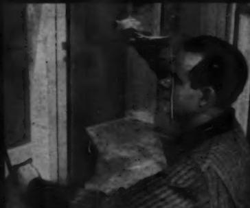
**3. NAIL TO STUD.** Nail bottom anchors first. Then, the rest. Recheck for trueness.
