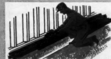
**FLEXCELL® PERIMETER INSULATION.** Asphalt impregnated throughout entire thickness of the board. For concrete slabs at grade. Like all Celotex Fiber Board products, effectively protected against dry rot and termites by exclusive Farox® process.
