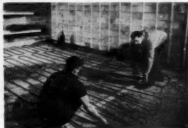
**Heat for this basement game room** will be provided by 1/2" PG's embedded in a concrete slab. For floor or ceiling radiant panel heating systems, Anaconda PG's offer many installation economies. 5815
