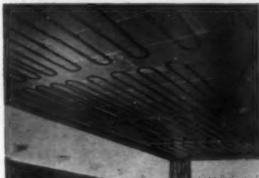
**Ceiling installation on gypsum lath.** Note changes in spacings—4 1/2" centers near the outside walls where heat loss is greatest but with the c-c spacing increased at the center and inside areas.
