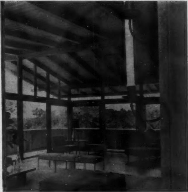
**TYPICAL** of the wood ceiling finish desired by home buyers, these glued, laminated ceiling beams provide an interior of large dimension. Roof deck is of the same wood. Southern Pine Assn. (Circle No. S74, p. 150.)
