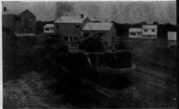
**LARGE EQUIPMENT** like this 25-yard scraper and D-8 bulldozer can cost many times the rate of the little machine. But on big jobs, their speed will more than make up the difference in rate.
