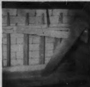
**PLYWOOD** patterns fastened to wood frame hold fire brick in place until mortar sets—it saves time—gives better job—and it's reusable too.
