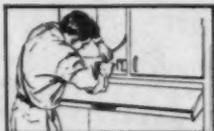
Remove junction box cover and connect two white to white of line and black to black of line. Replace junction box cover.
