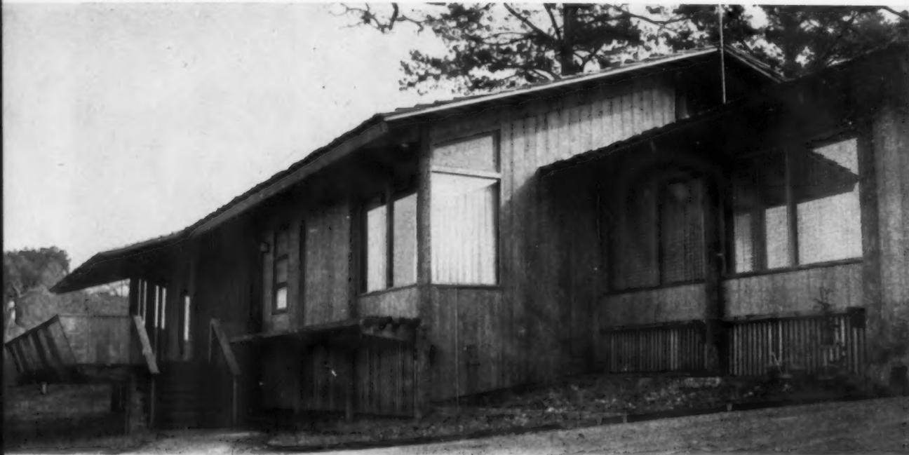
**FROM OUTSIDE**, poles are visible as attractive modular bays. Ends of cantilevered floor beams support front
