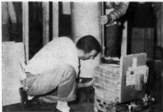
1. **HOT WATER TANK** is nipped to the boiler. Only two union connectors necessary. This job took 10 min.
