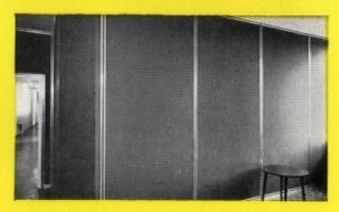
Stramit partitions in aluminium framing—a system within a system for large blocks of offices and flats
