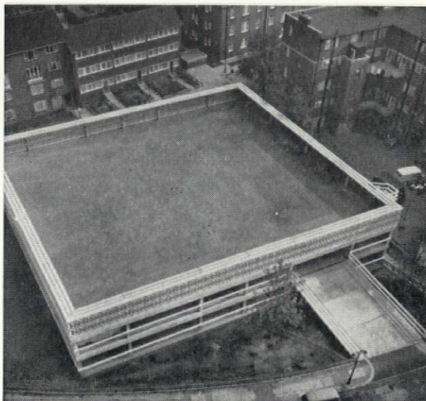
Below: Roof of Car Park surfaced with Permanite Paving Asphalt to form Children's Playground
