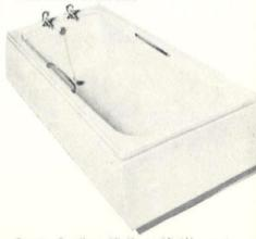
Carron, Swallow, 6ft 0in  $\times$  2ft  $4\frac{1}{2}$ in, cast iron porcelain enamelled, fibreglass side
