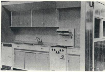
The Howard Heart Unit 11ft 1in  $\times$  8ft 3in, sandwich construction with fire-resistant phenolic foam core, PVC soil pipe, acrylic and FRP bath. Cupboards outside bathroom contain heating equipment for hot water supply and warm air circulation. Kitchen provided with extract fan
