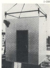
Concrete bathroom unit being placed in position, Budapest
